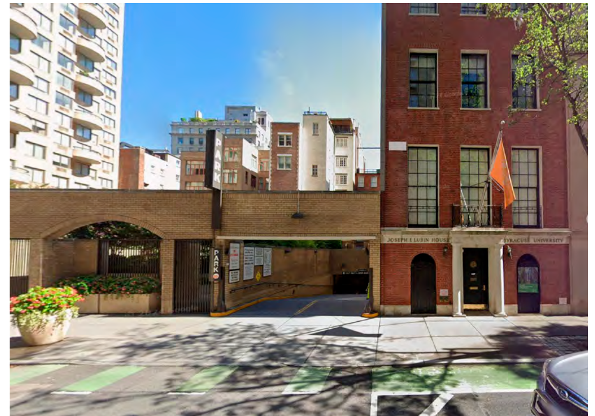
View of parking garage entrance.
