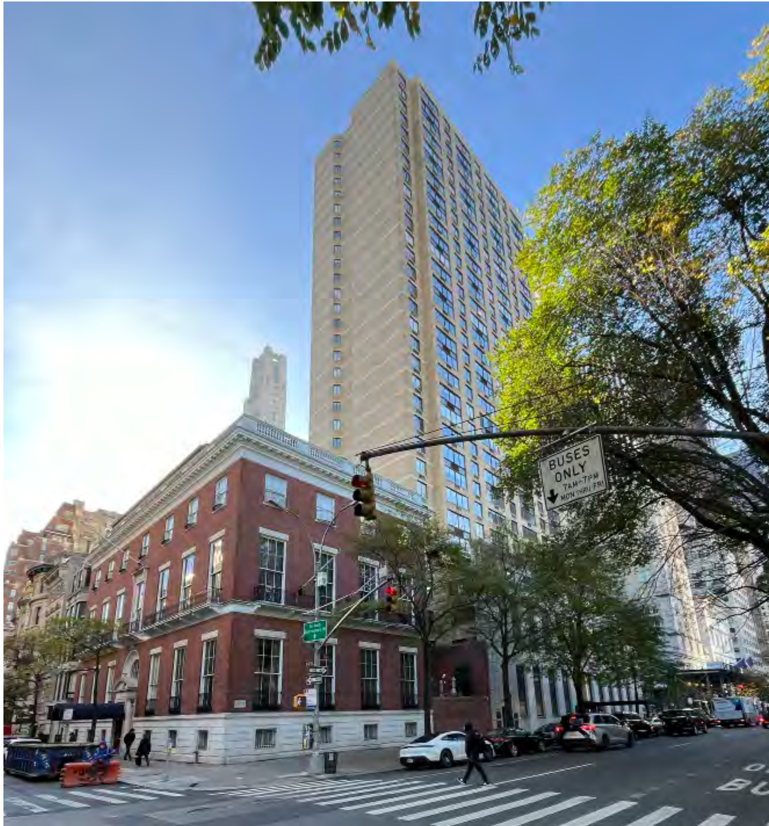
View of building looking southeast.
