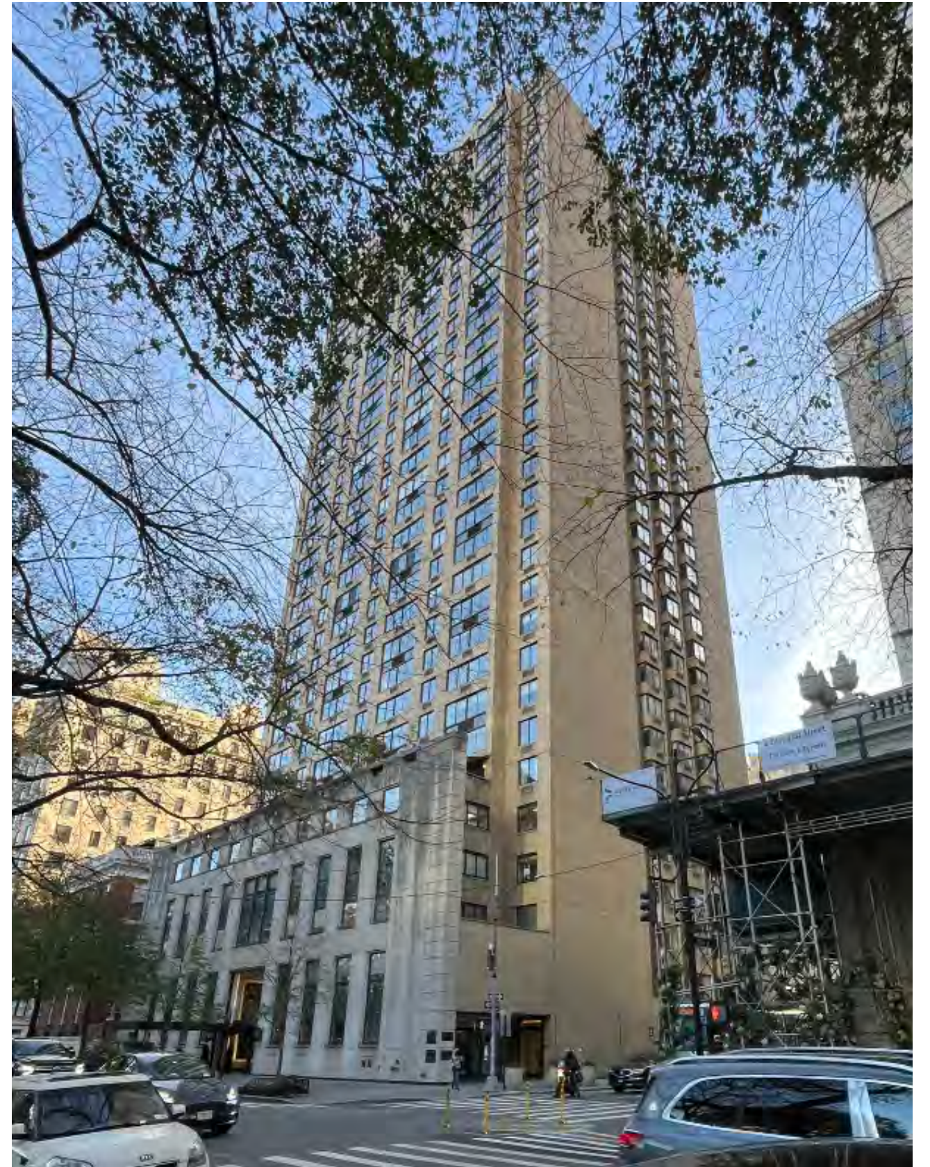
View of building looking northeast.
