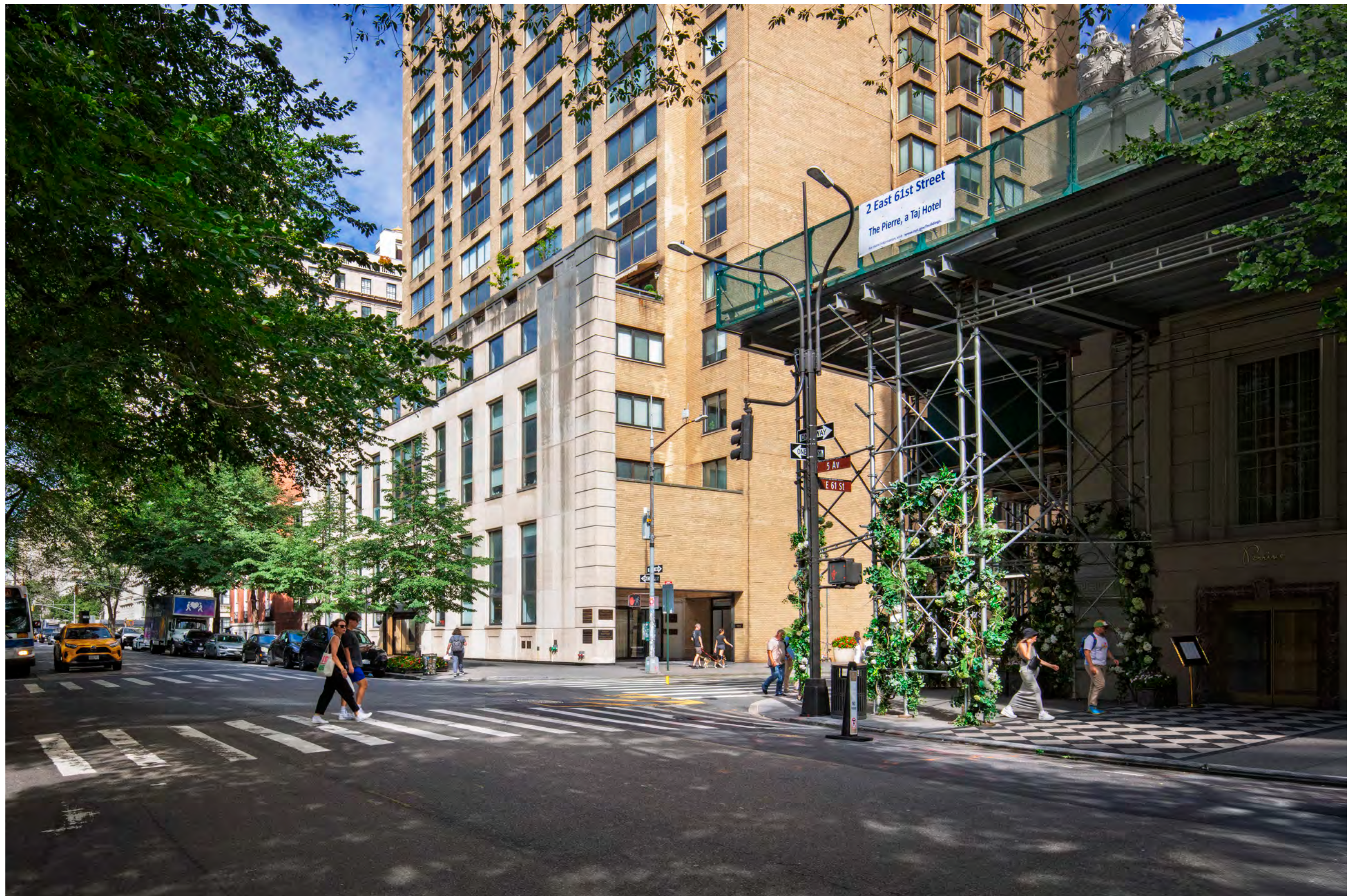
View From 5th Avenue Looking North East Existing
