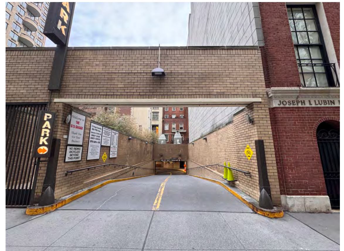
View of parking garage ramp.
