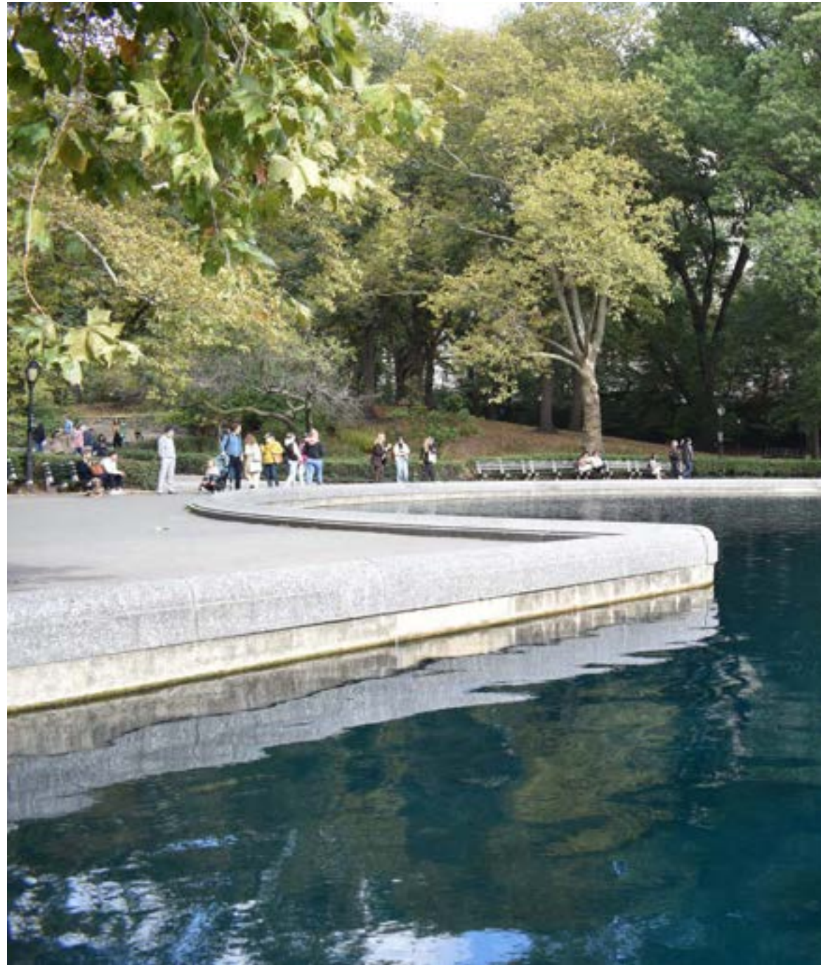
Existing perimeter wall, looking north towards Alice in Wonderland
