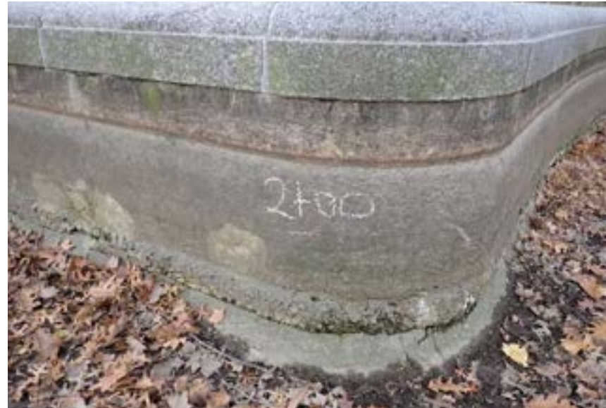
Early 20th Century Concrete Walls
