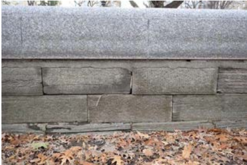
Masonry Block Walls
