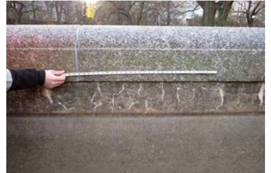
CPC Replacement Concrete Walls
