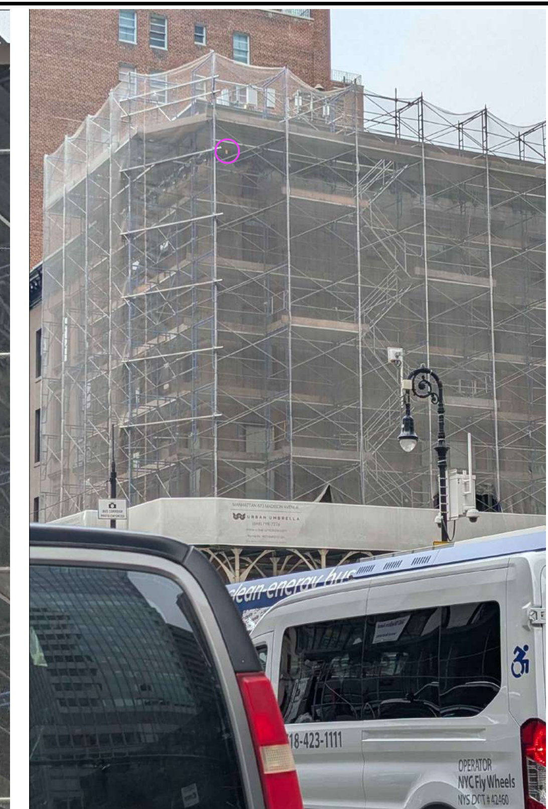
PHOTO 7. POINT C. ORANGE CYLINDER MOCKUP VISIBLE, BUT BLACK FIXTURE ISN'T VISIBLE @ TOP CORNICE
