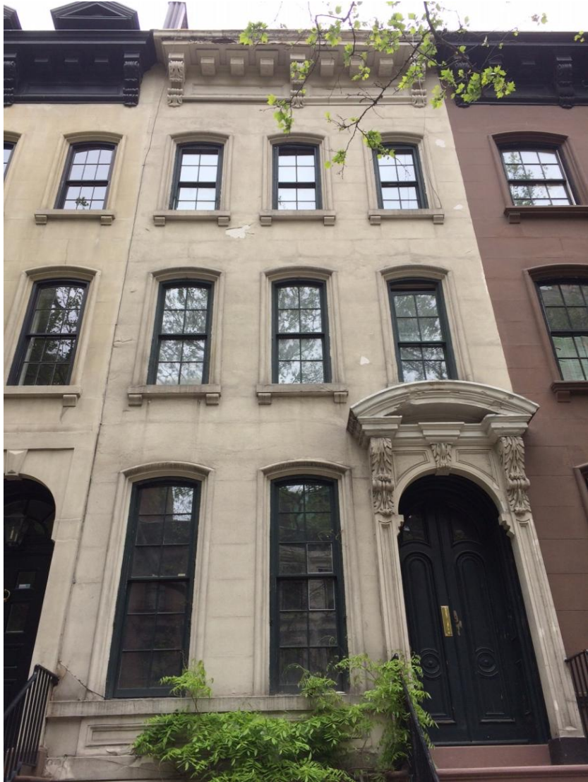
PRE CONSTRUCTION – SOUTH STREET FAÇADE
