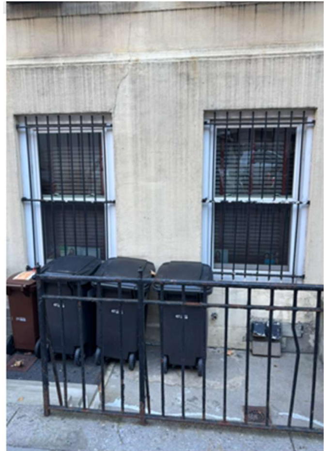
CLOSE UP OF 2 GROUND FLOOR WINDOWS, EXISTING
