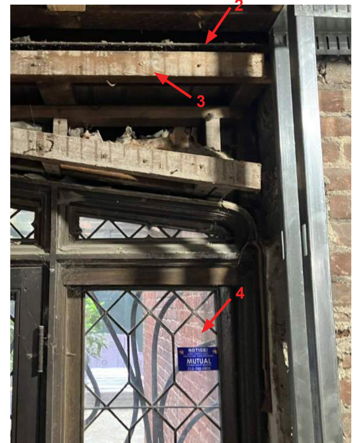
PHOTO OF EXISTING LINTEL FROM INTERIOR
