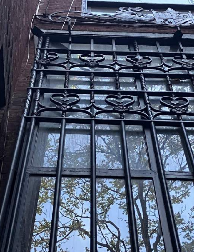
PHOTO OF EXISTING FROM EXTERIOR
