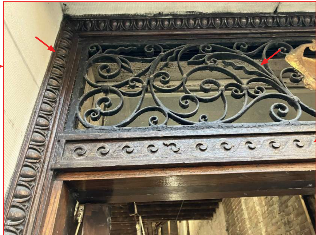
EXISTING BRICK MOLDING, TRANSOM TRIM, AND IRONWORK TO REMAIN
