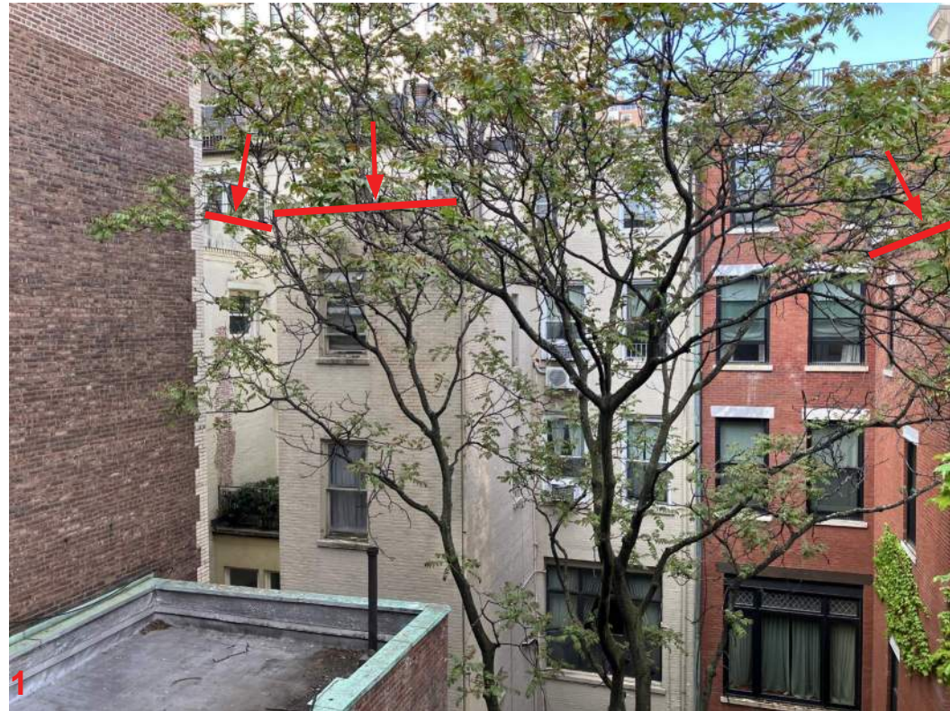
VIEW FROM EXIST REAR 4TH FLOOR WINDOW
