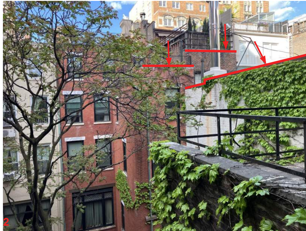
VIEW FROM EXIST REAR 4TH FLOOR WINDOW
