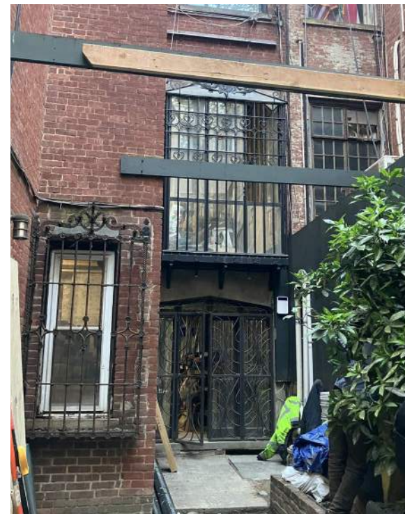
PHOTO OF EXISTING FROM EXTERIOR
