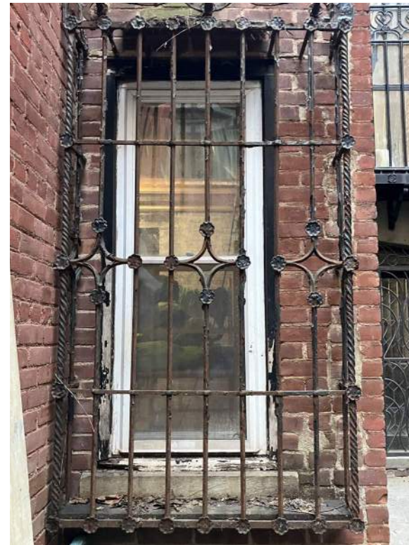
PHOTO OF EXISTING FROM EXTERIOR
