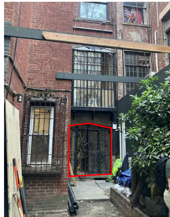
PHOTO OF EXISTING FROM EXTERIOR
