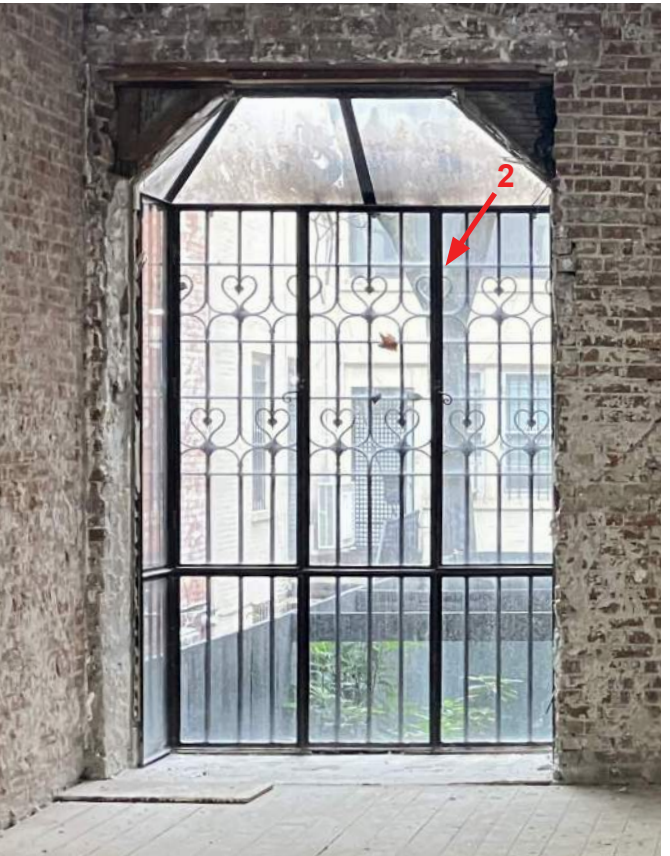
PHOTO OF EXISTING FROM INTERIOR
