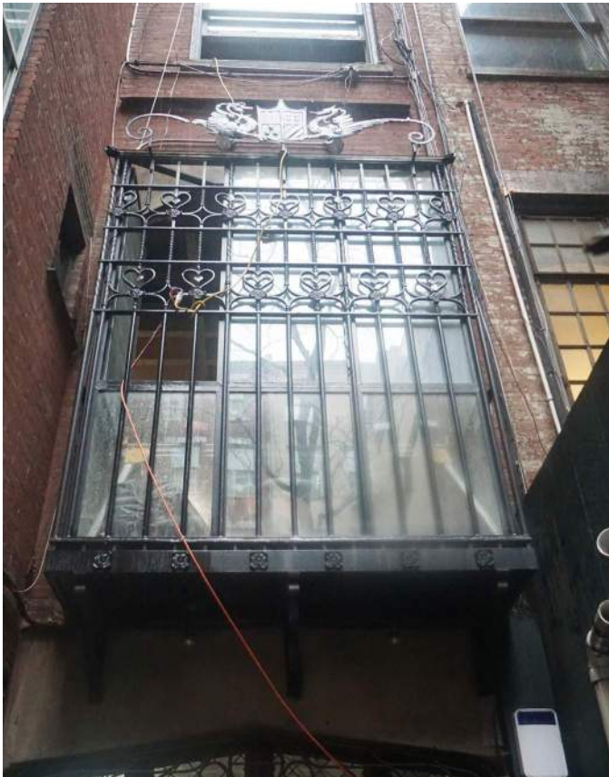
PHOTO OF EXISTING FROM EXTERIOR
