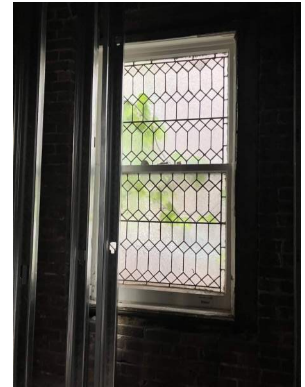
PHOTO OF EXISTING WINDOW FROM INTERIOR
