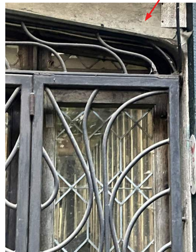
PHOTO OF EXISTING FROM EXTERIOR
