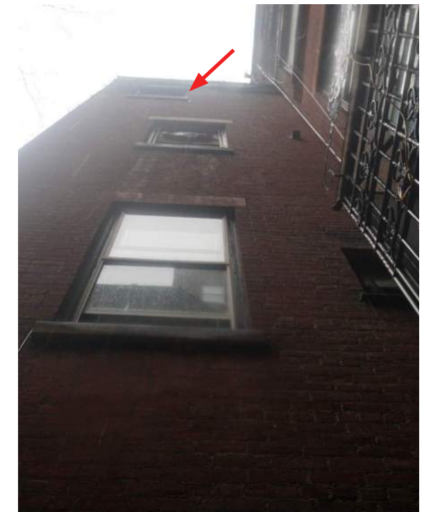
PHOTO OF EXISTING WINDOW FROM EXTERIOR
