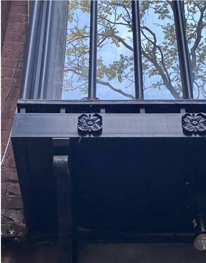
PHOTO OF EXISTING FROM EXTERIOR
