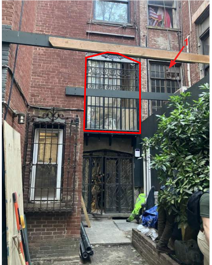
PHOTO OF EXISTING FROM EXTERIOR
