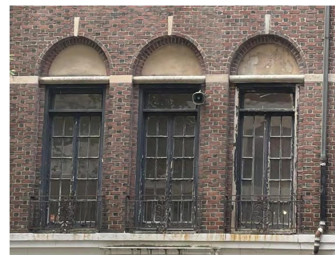
EXISTING WINDOWS AT 48 EAST 73RD STREET. THE ARCHES ARE SOLID AND APPEAR TO HAVE BEEN COVERED WITH PAINT. THE HALF-ROUND LINTELS BETWEEN THE FRENCH DOORS AND ARCHES ARE NOT ORIGINAL (SEE 1940'S TAX PHOTO BELOW).
