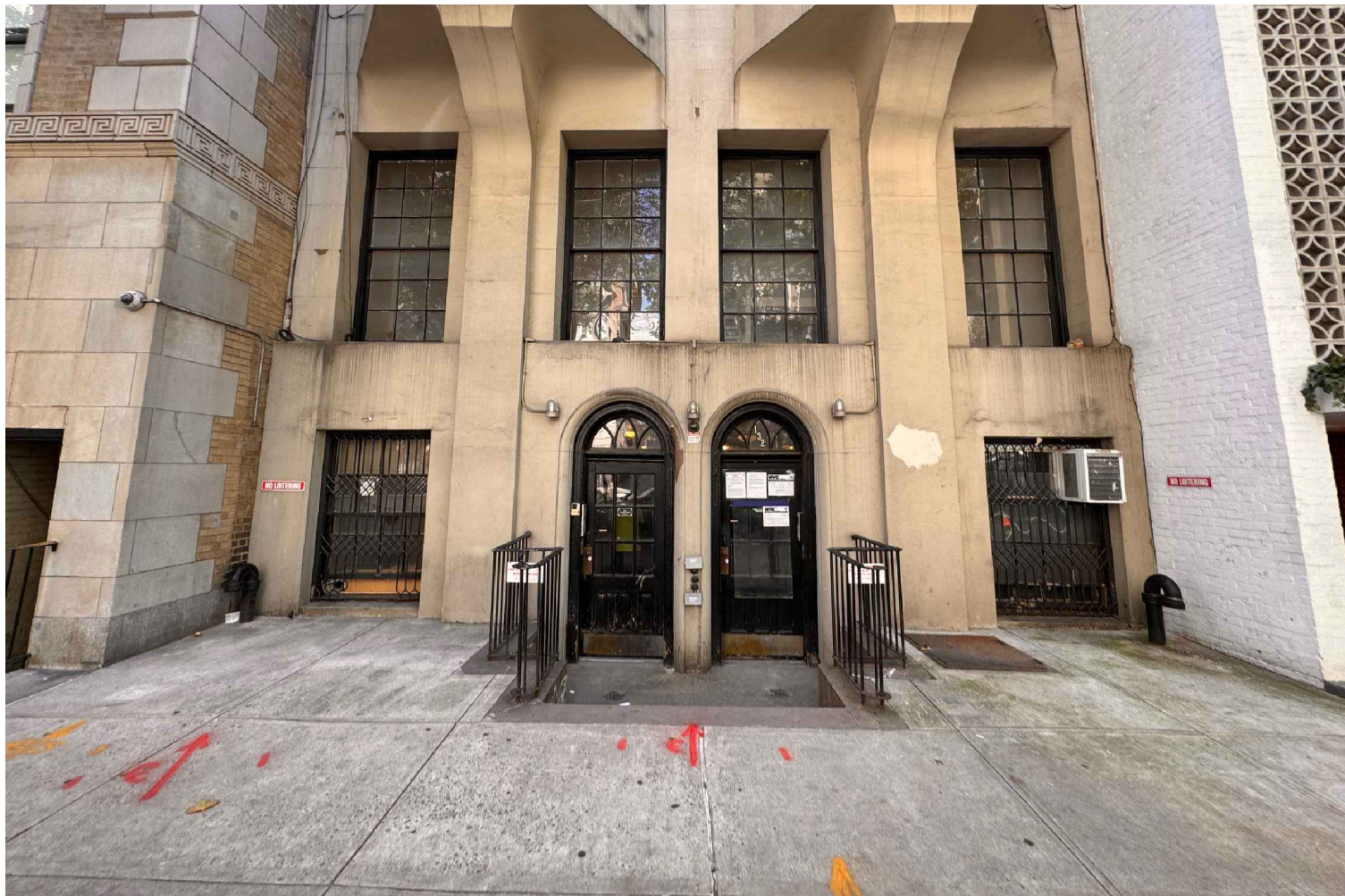
3. SITE PHOTOGRAPH- PERSPECTIVE LOOKING SOUTHWEST
