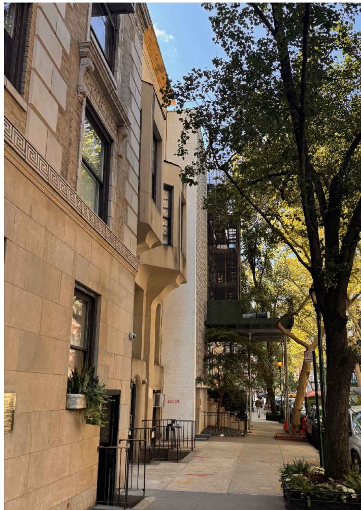
1. SITE PHOTOGRAPH- PERSPECTIVE LOOKING NORTHWEST
