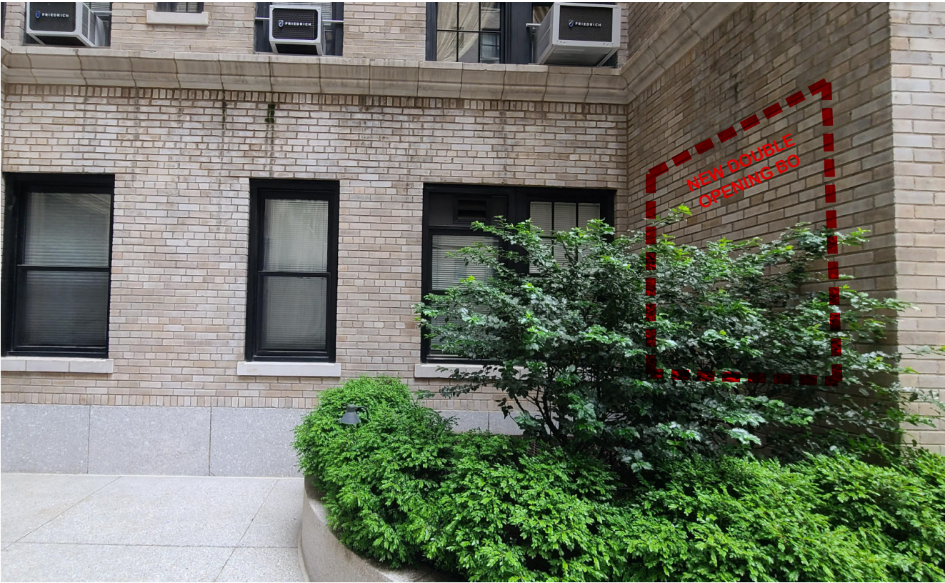
Existing wall Condition - Exterior View (West facade Inner courtyard) 23A
