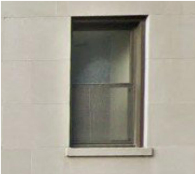
Existing Windows Condition - Exterior View 5
