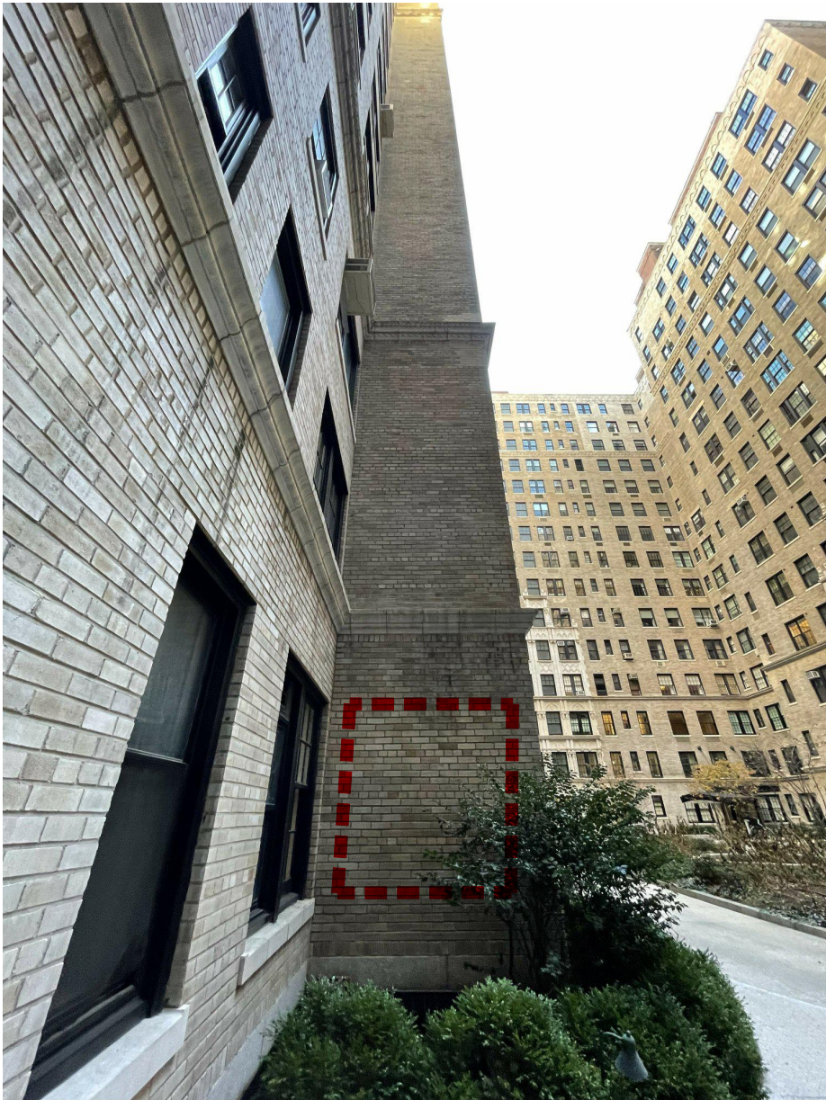
Existing Windows Condition - North Courtyard (Showing Proposed Window Opening for Louver)
