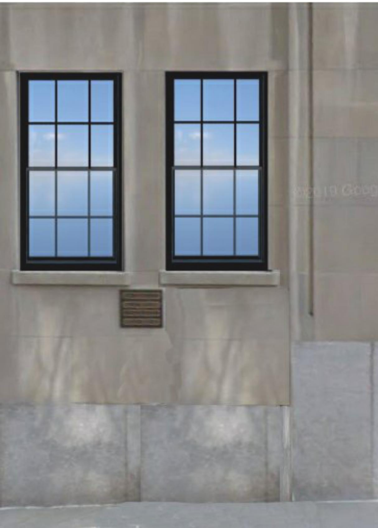
Proposed Window Condition - Exterior View 10
