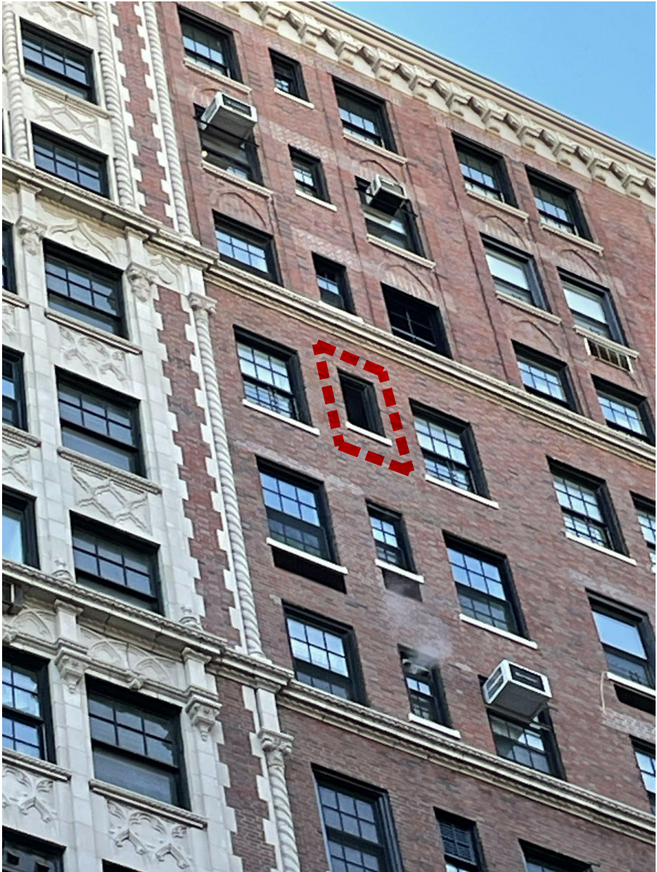
Existing Windows Condition - 94th Street (Showing Existing Window Openings With Louvers)
