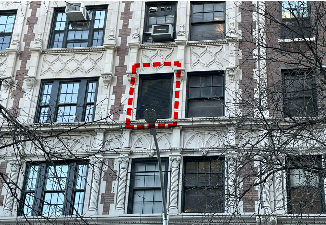
Existing Windows Condition - 94th Street (Showing Existing Window Openings With Louvers)
