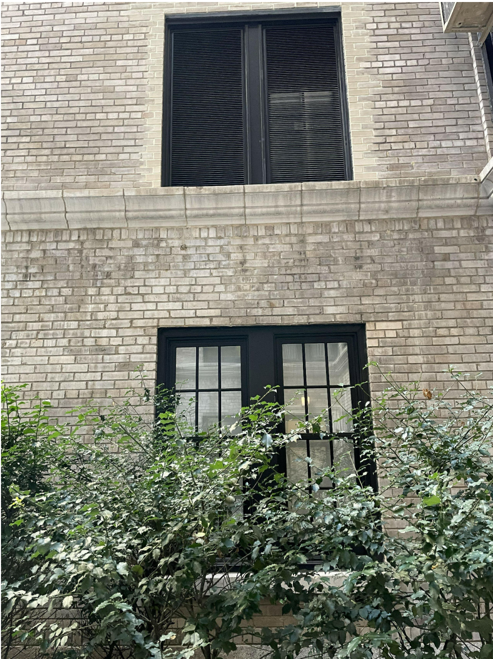
Existing Windows Condition - South Courtyard
