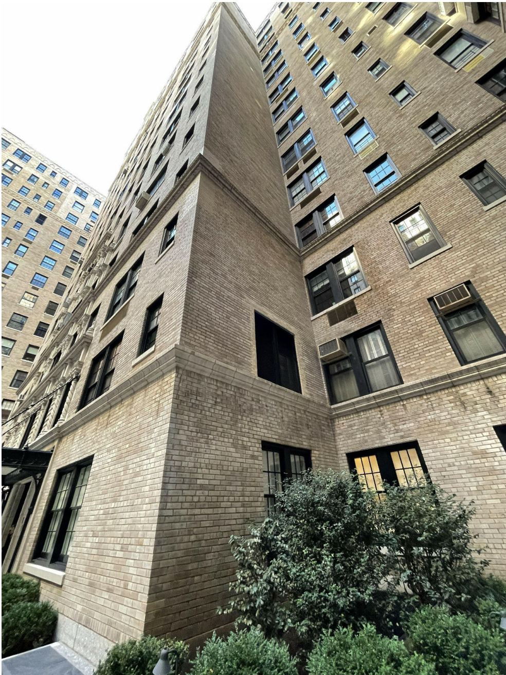
Existing Windows Condition - South Courtyard
