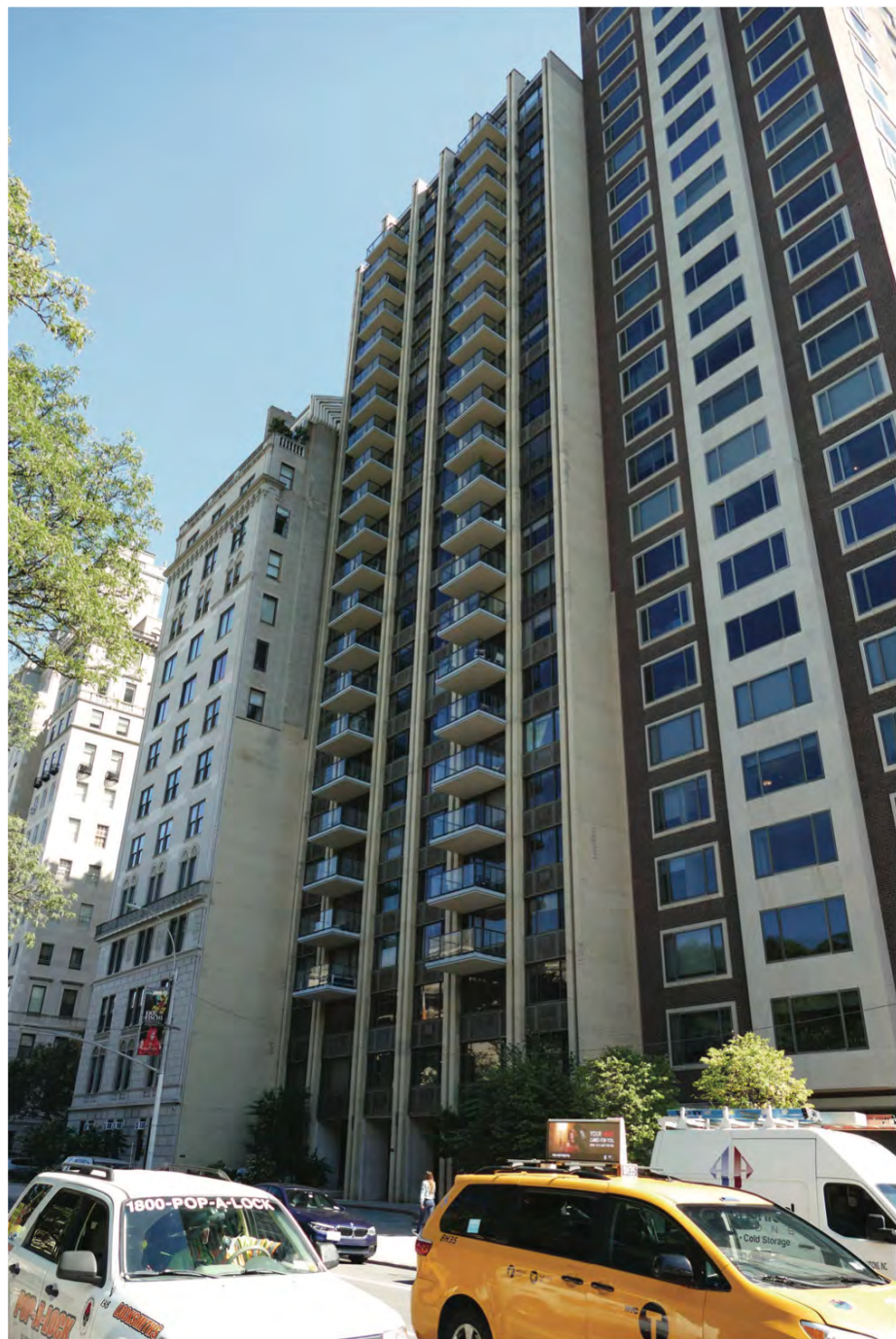
Existing Condition on Fifth Avenue.
