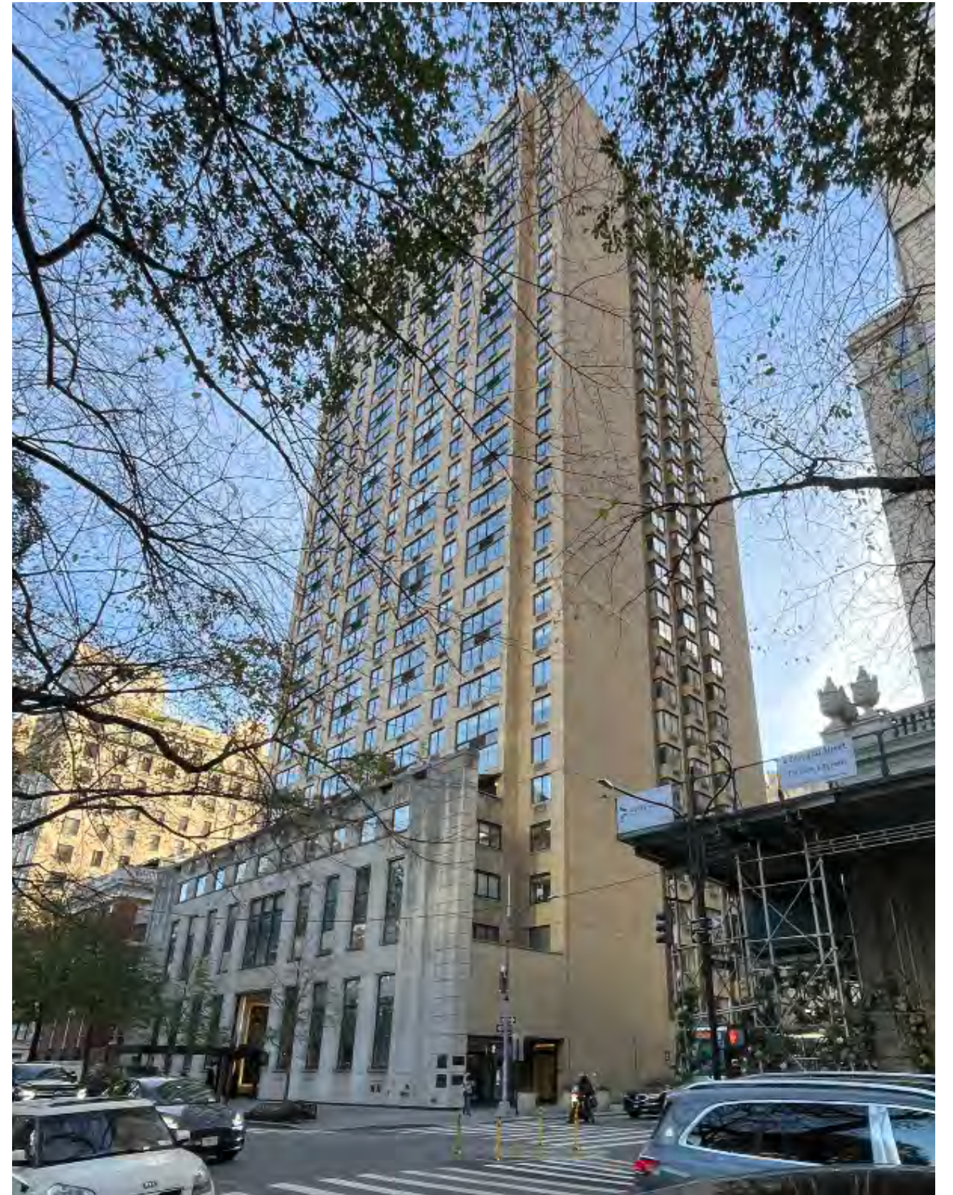
View of building looking northeast.
