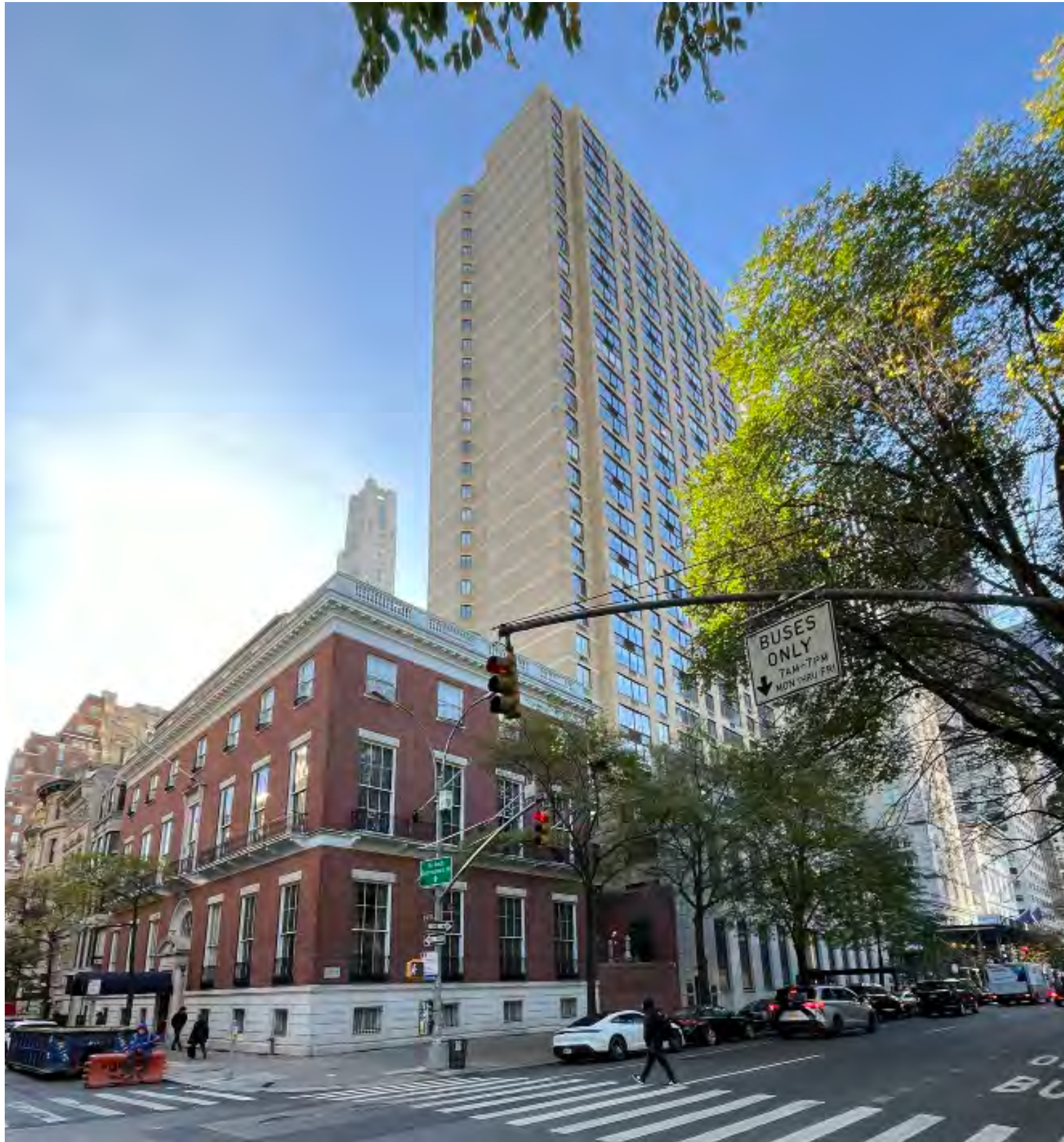
View of building looking southeast.
