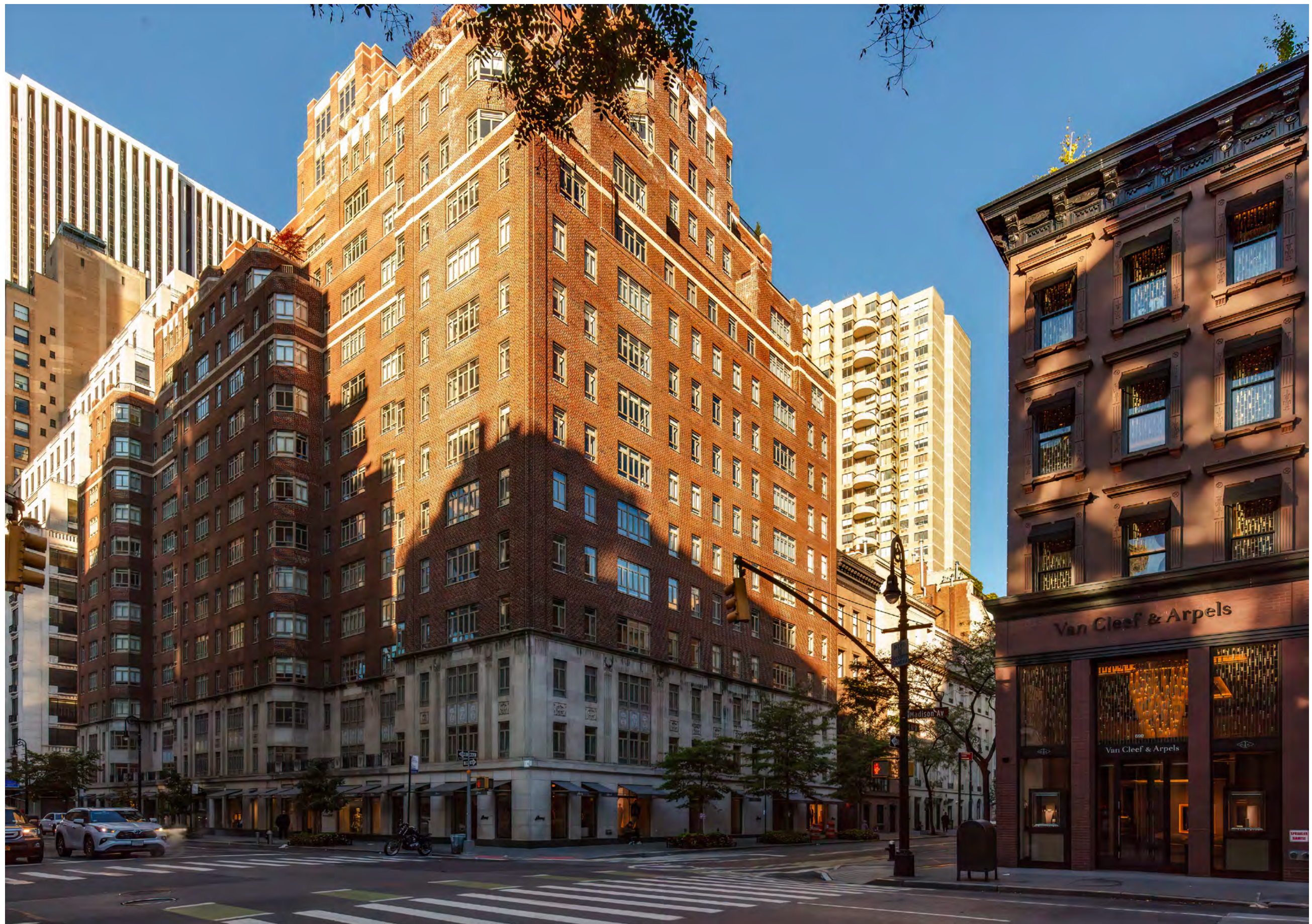
VIEW FROM MADISON AVENUE LOOKING SOUTHWEST EXISTING
