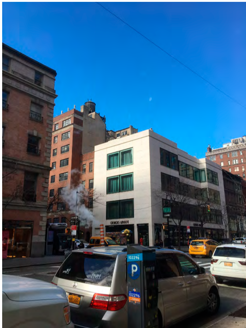
Existing Condition on Madison Avenue.
