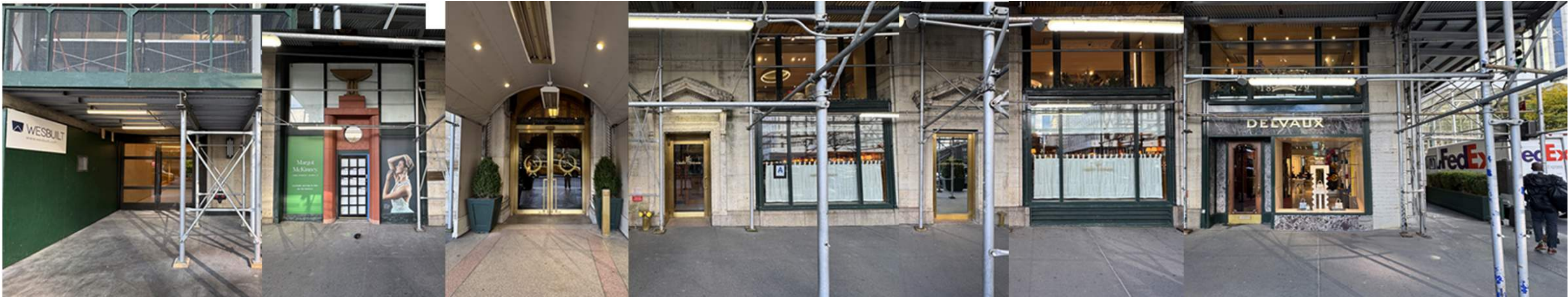
PANORAMA OF 5TH AVENUE BETWEEN 60TH & 59TH ST LOOKING EAST SHERRY NETHERLAND STOREFRONTS
