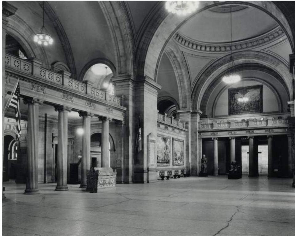
GREAT HALL, LOOKING NORTH, 1940'S The light post fixtures on the balcony parapet have been removed.
