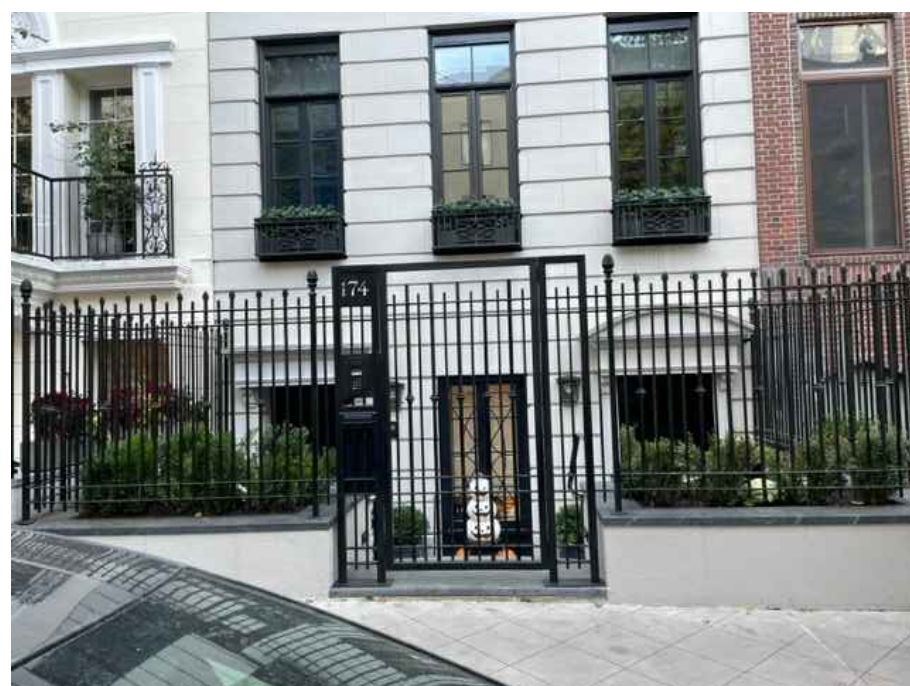
#174 EAST 64TH ST. FENCE HEIGHT: 7'-4"
