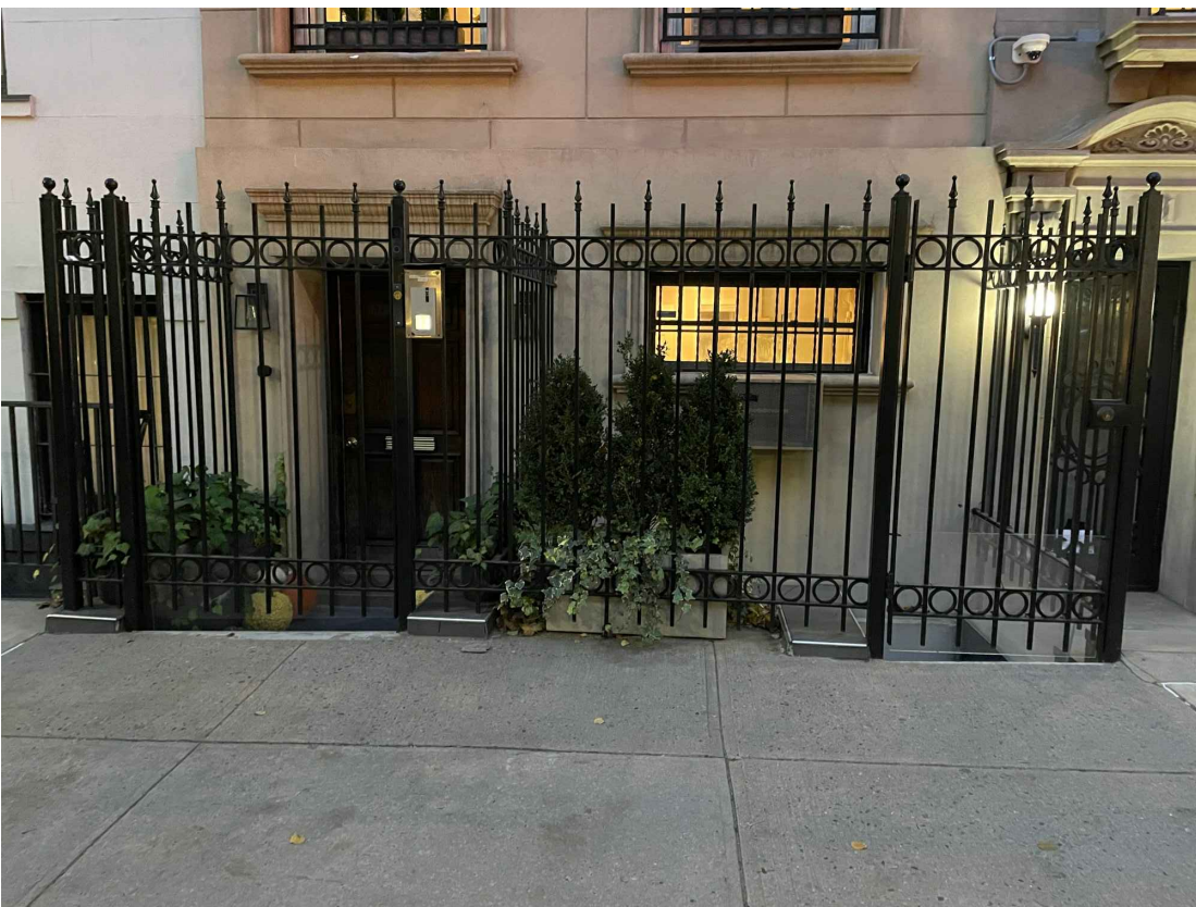
#179 EAST 64TH ST. FENCE HEIGHT: 6'-5"
