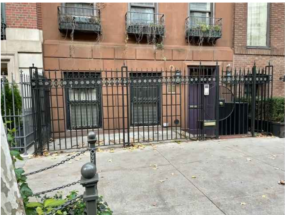
#165 EAST 64TH ST. FENCE HEIGHT: 6'-2"
