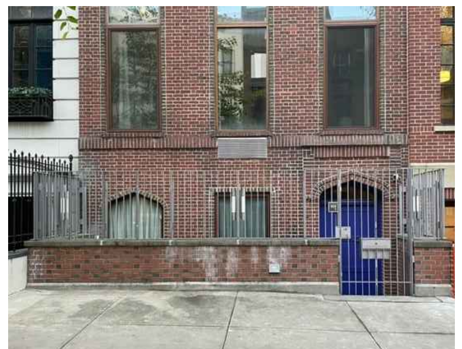
#172 EAST 64TH ST. FENCE HEIGHT: 6'-0"
