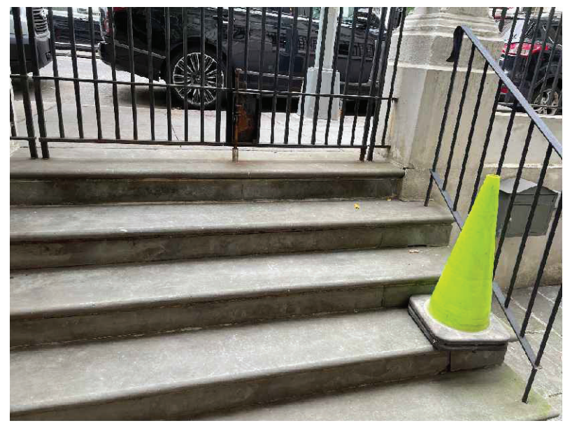
2 SITE PHOTO DOT-1
