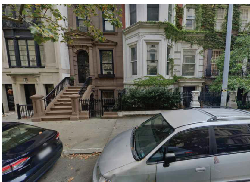
3 SITE PHOTO DOT-1
