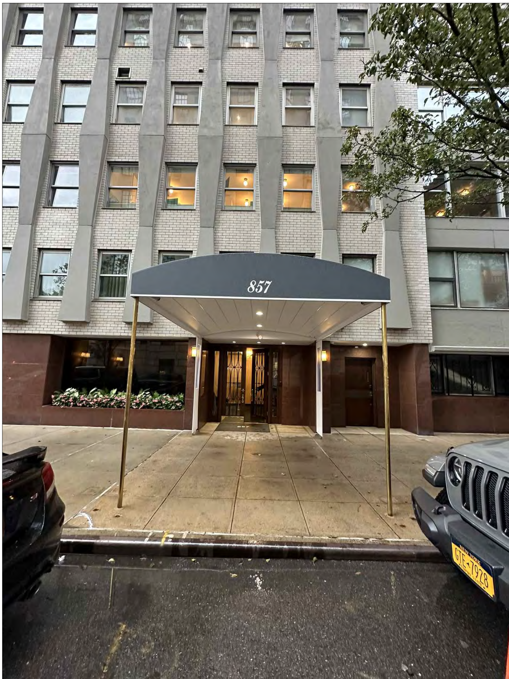
6 EXISTING SOUTH ELEVATION - VIEW TOWARDS ENTRY Scale: NTS
