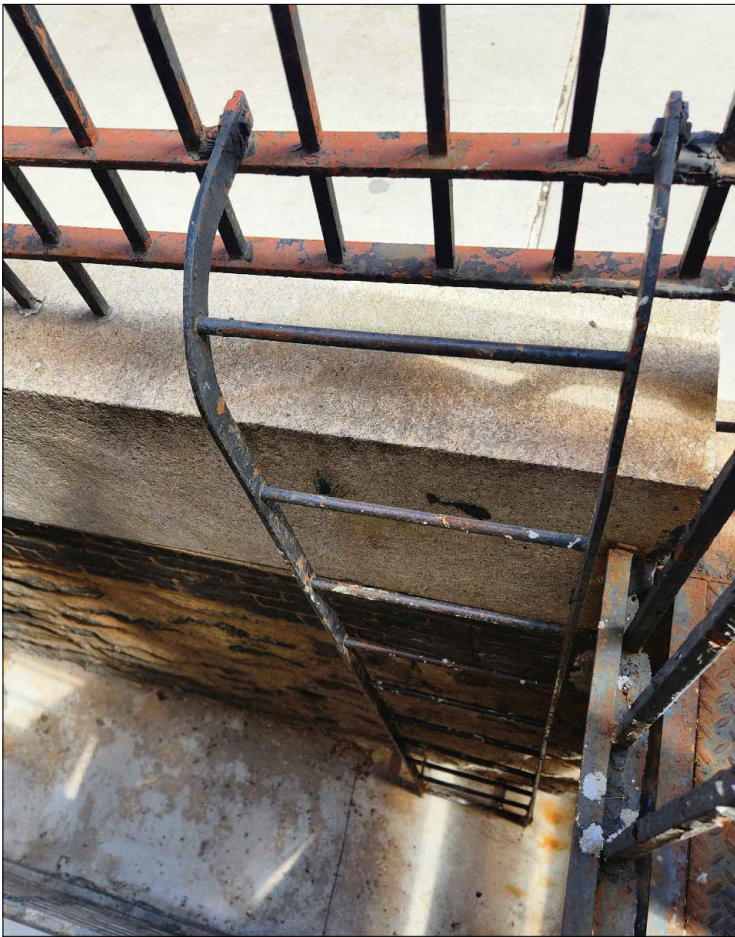
5 EXISTING AREAWAY SERVICE LADDER NOT TO SCALE
