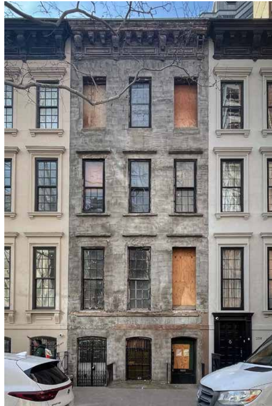
As-Built Photograph of Street Facade (with Scratch Coat Applied)
