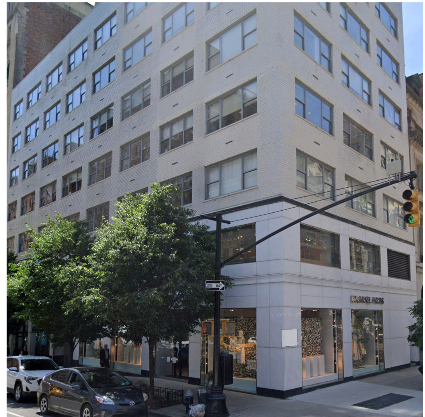
790 Madison Avenue, 2023. 2010 COFA for removal of granite veneer at ground floor and brick from second floor; installation of new masonry cladding at bottom two floors. No style building in UES.
