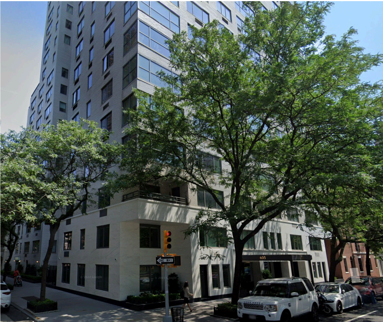
605 Park Avenue. 2016 COFA to remove the first and second floor cladding, and install white marble cladding with a black granite water table.
