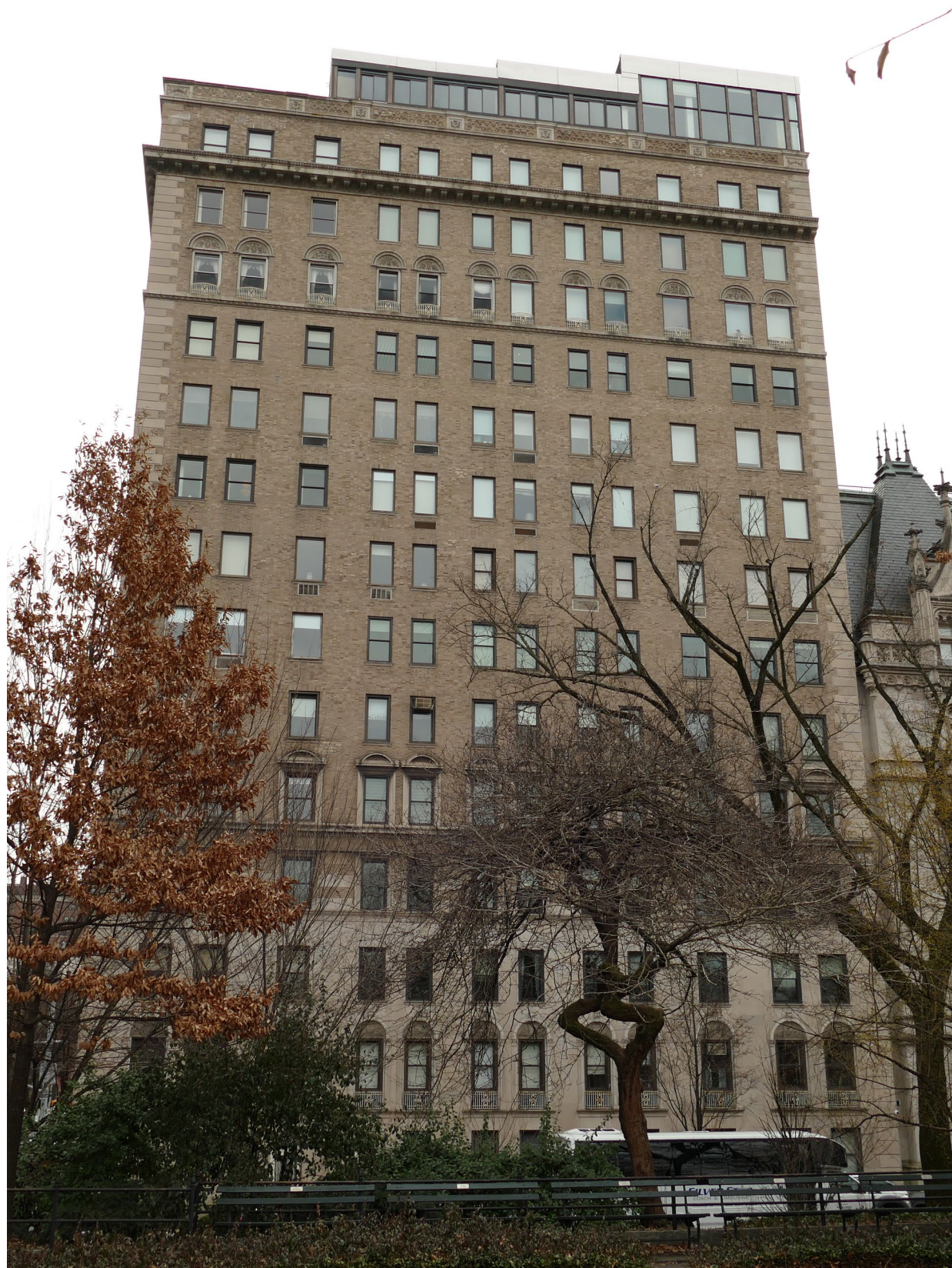
1115 Fifth Ave - primary facade.
