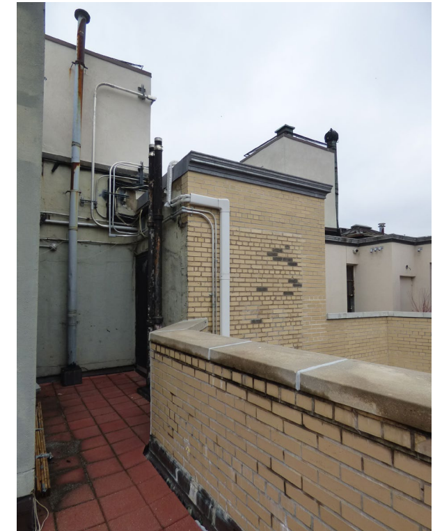
3. East elevation at the south lightwell, looking northwest.
