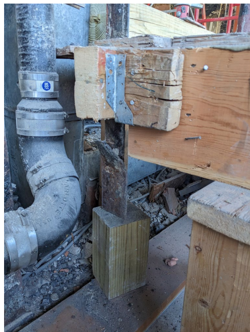
EXISTING INTERIOR STRUCTURAL CONDITIONS
