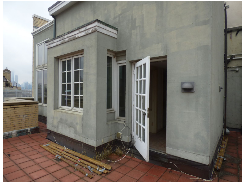
2. East elevation, looking southwest
