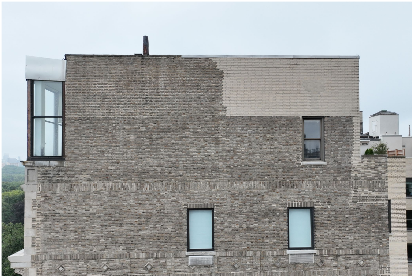
4. Overview of the south elevation
