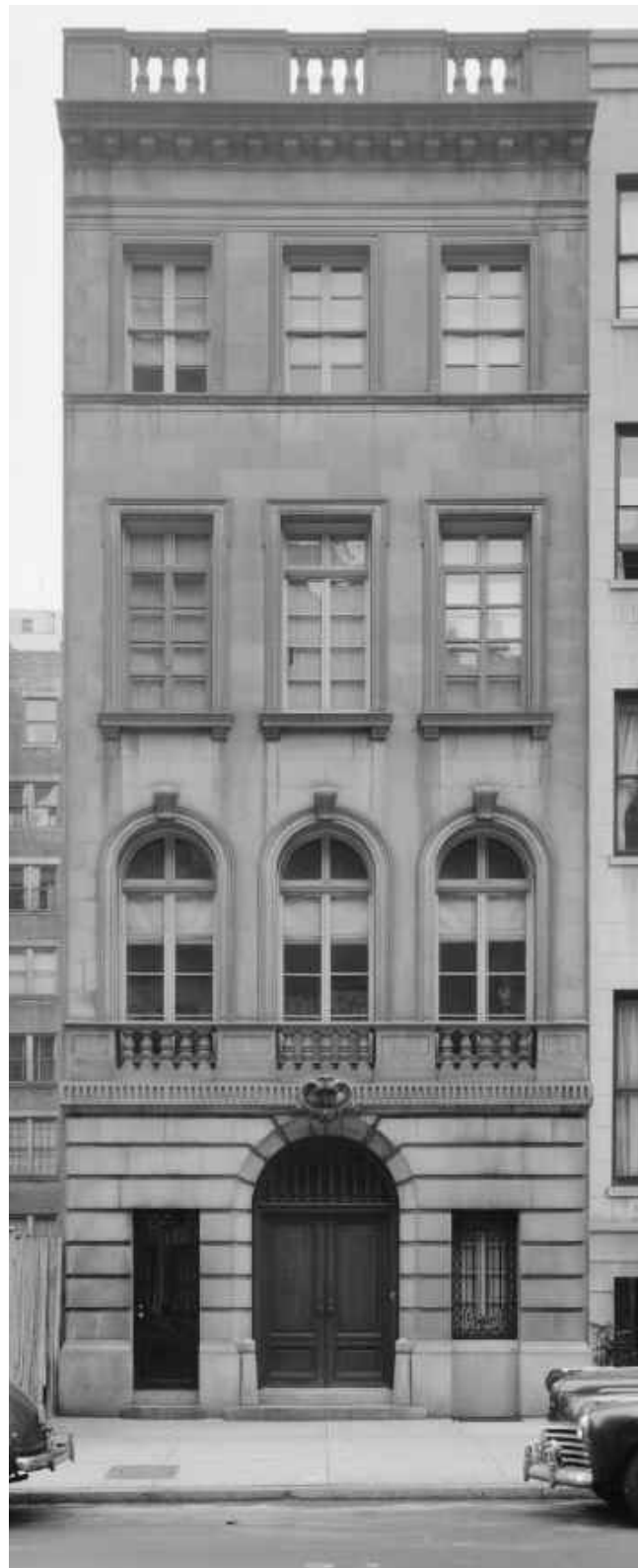
FRONT (NORTH) FACADE) - 1946
