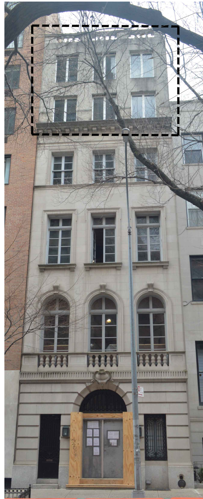
FRONT (NORTH) FACADE - CURRENT
