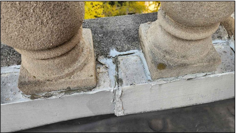
Salvaged stone balusters bearing on EIFS/CMU
