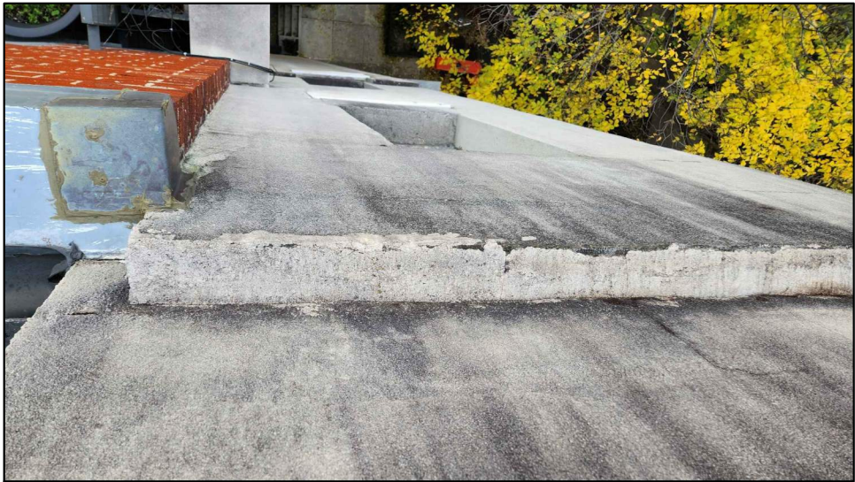
Ragged edges & discoloration of deteriorated EIFS
