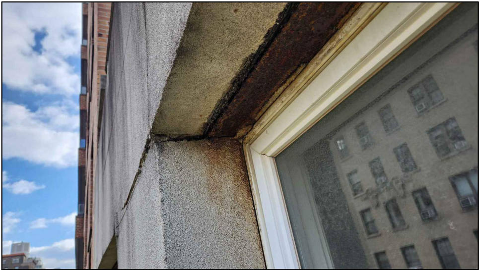
Corroded lintels, rust-jacking, rust-staining around window, delaminating EIFS, no sign of flashing
