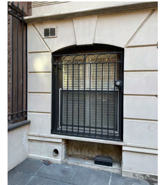
Existing Grille at 17 E77th Street
