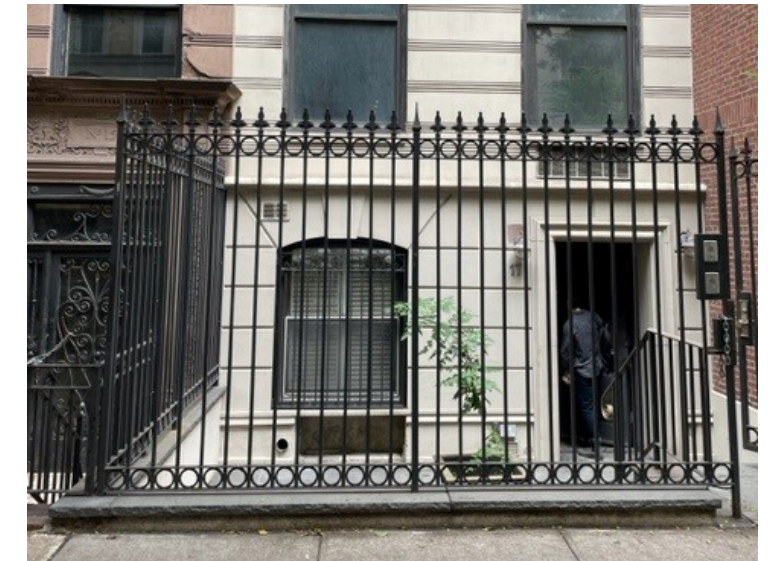
Existing Fence at 17 E77th Street
