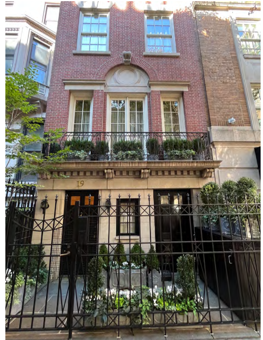
Areaway at 19 E77th Street
