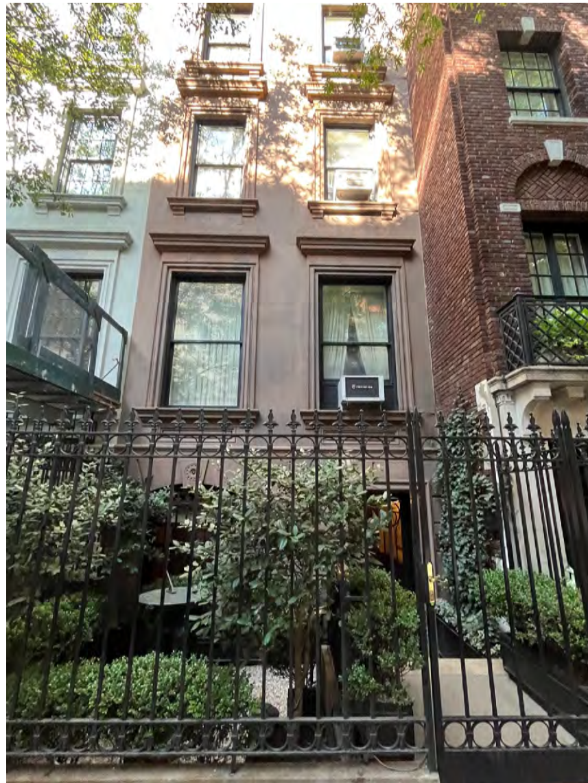
Areaway at 11 E77th Street
