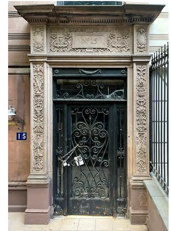
Existing Stone Door Surround at 15 E77th Street
