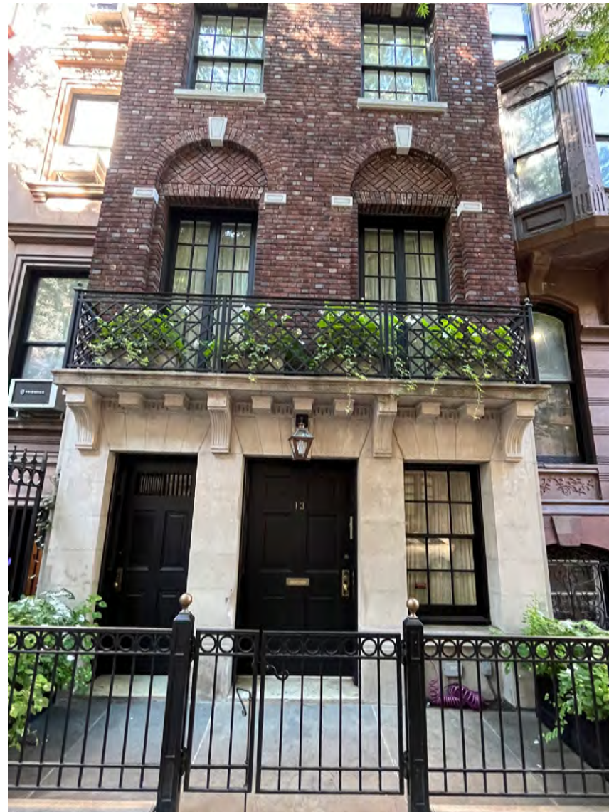
Areaway at 13 E77th Street
