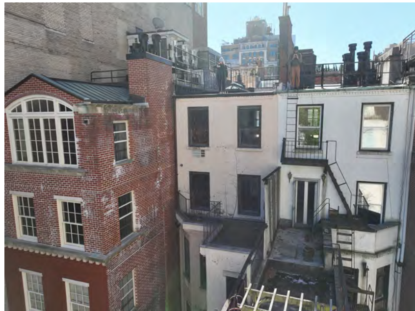
Existing Rear Facade at 15-17 E77th Street
