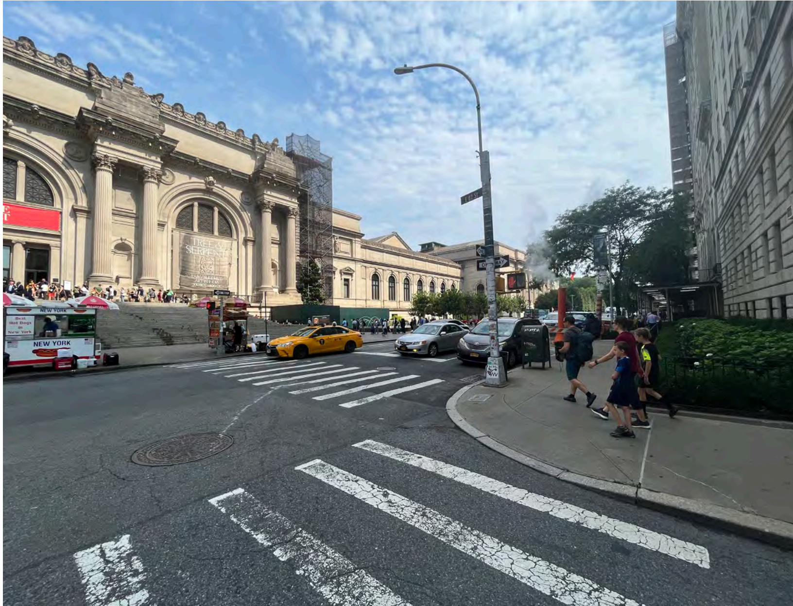
EXISTING CONDITION PHOTO WING E
