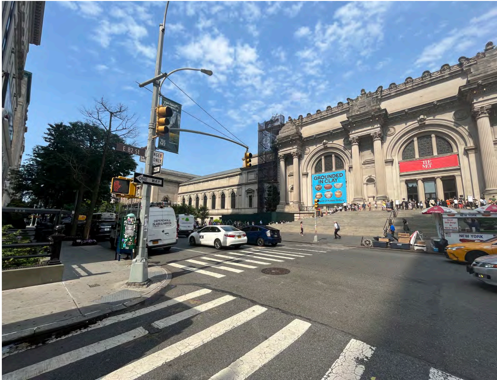
EXISTING CONDITION PHOTO WING J
