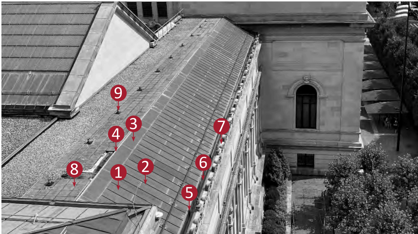
2 VIEW OF WING E ROOF LOOKING NORTH
