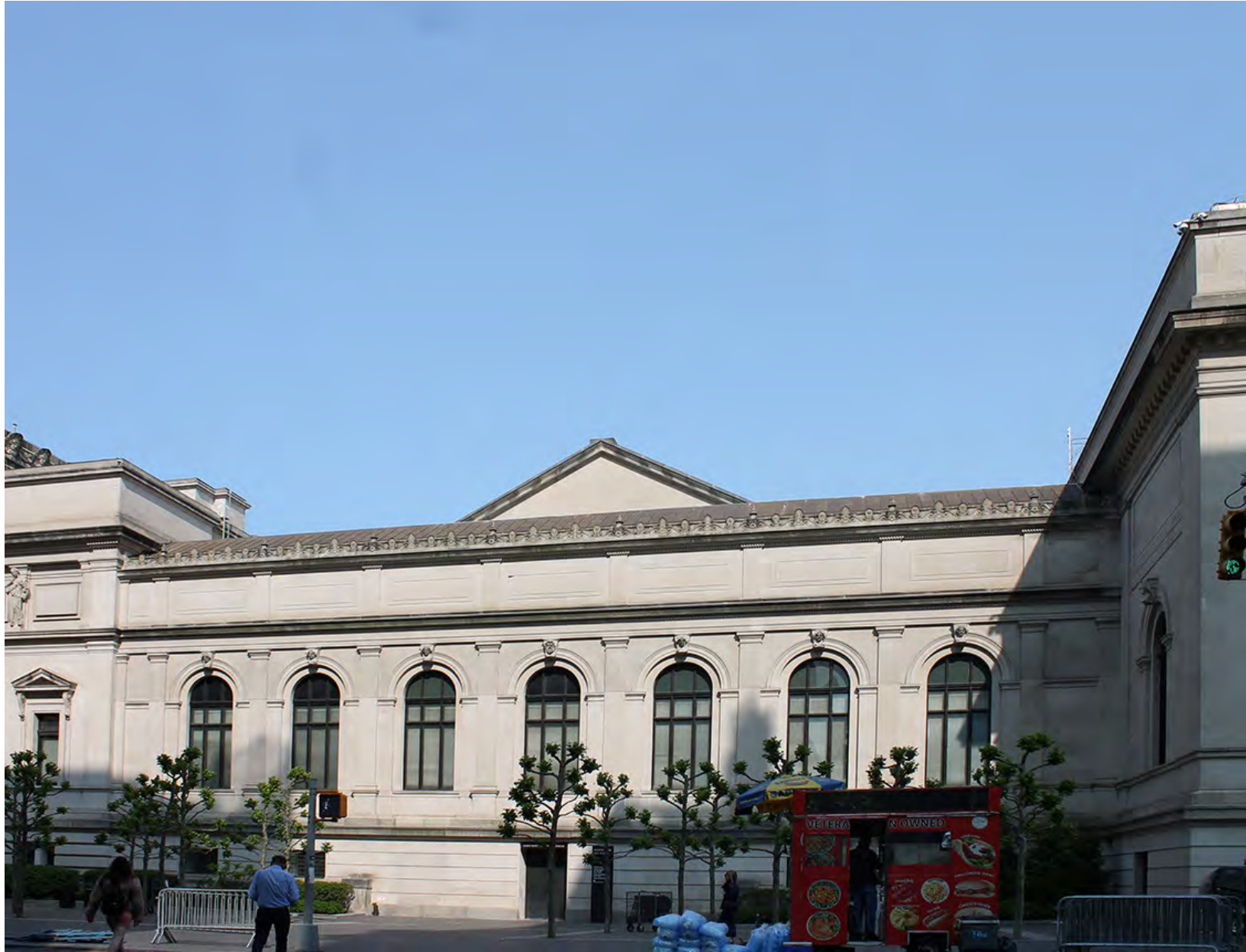
EXISTING CONDITION PHOTO WING E MONEL
