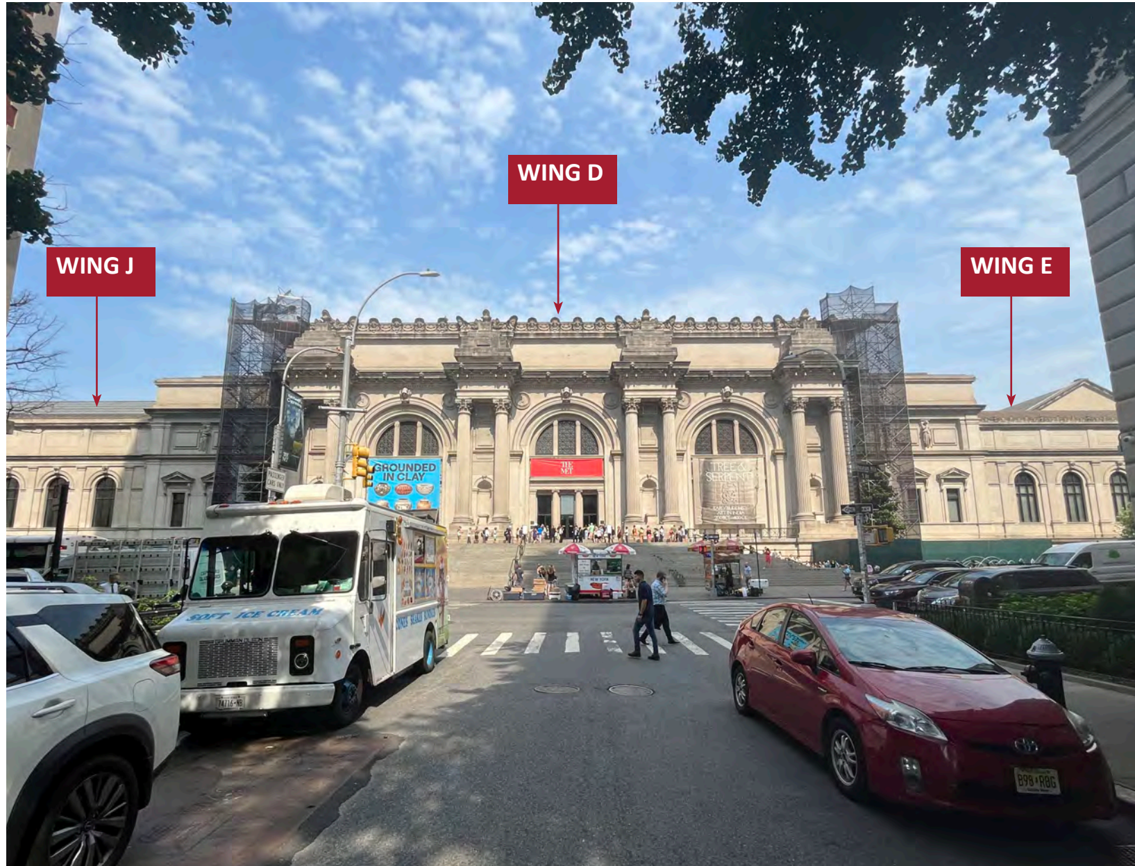
EXISTING CONDITION PHOTO WINGS J, D, AND E
