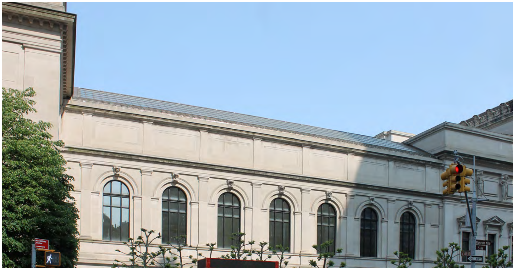
EXISTING CONDITION PHOTO WING J SKYLIGHT
