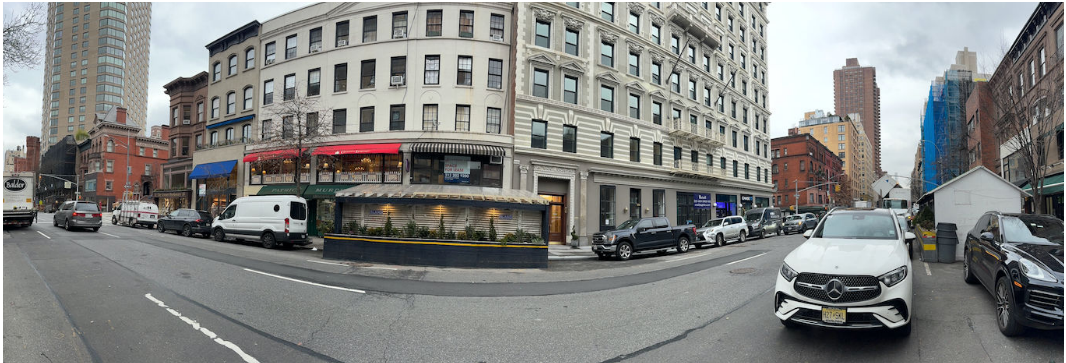
Madison Ave (East Elevation)
