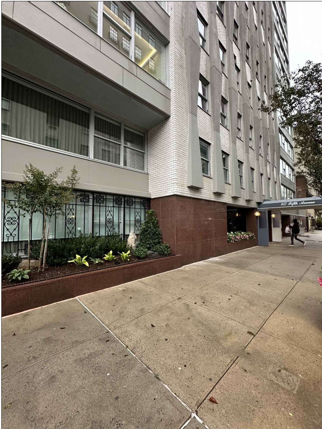
3 EXISTING NORTH ELEVATION - YARD ACCESS Scale: NTS
