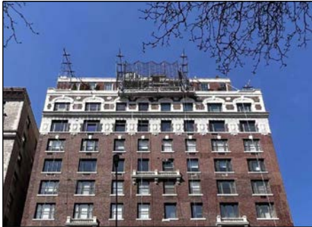
STREET VIEW, 970 PARK AVE
