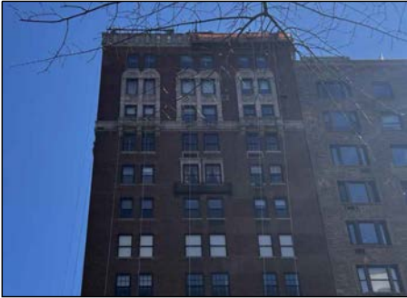
STREET VIEW, 935 PARK AVE
