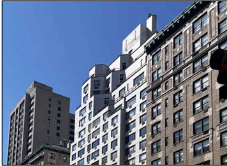
STREET VIEW, 920 PARK AVE
