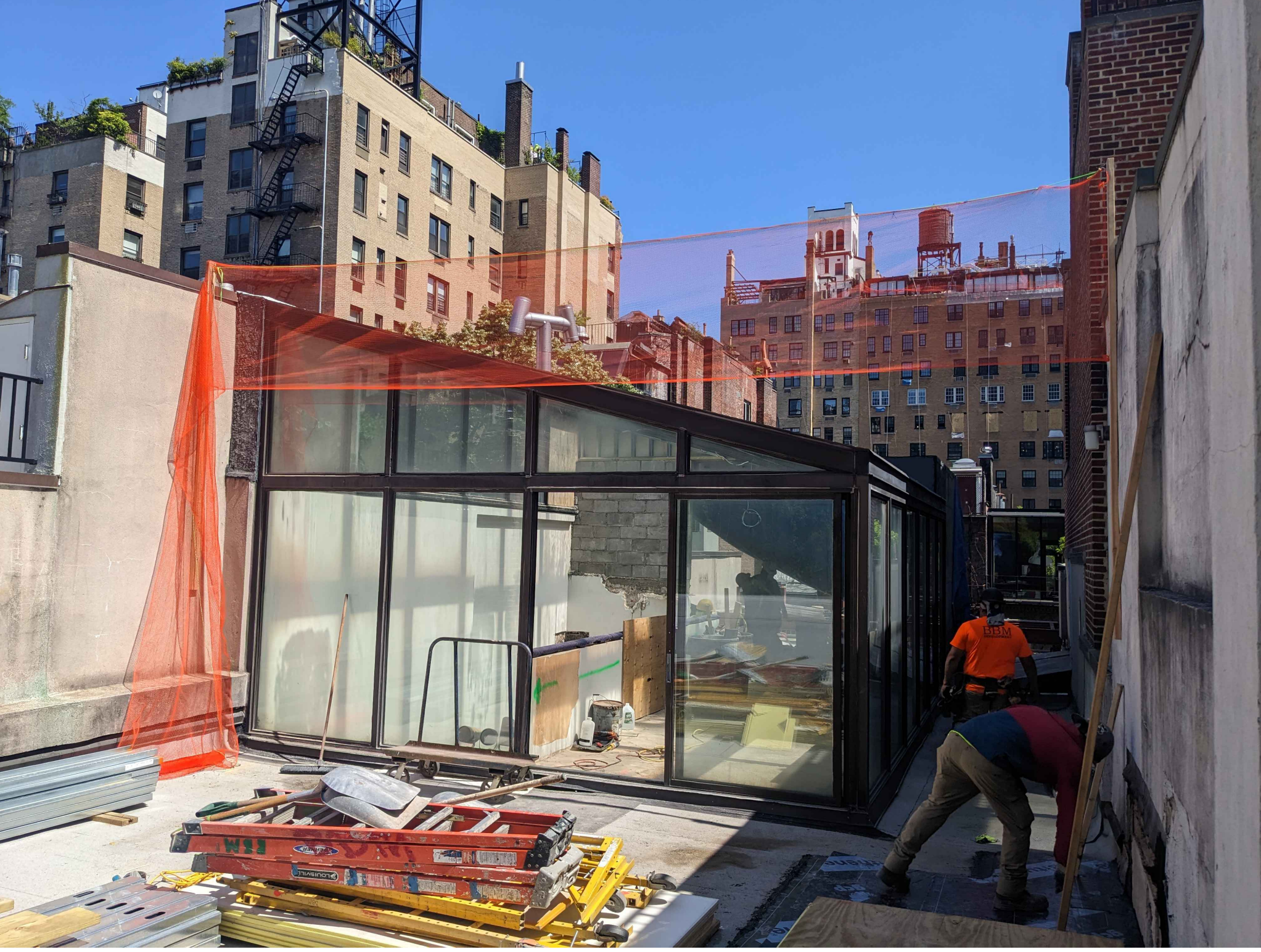
4 MOCKUP VIEW FROM ROOF
