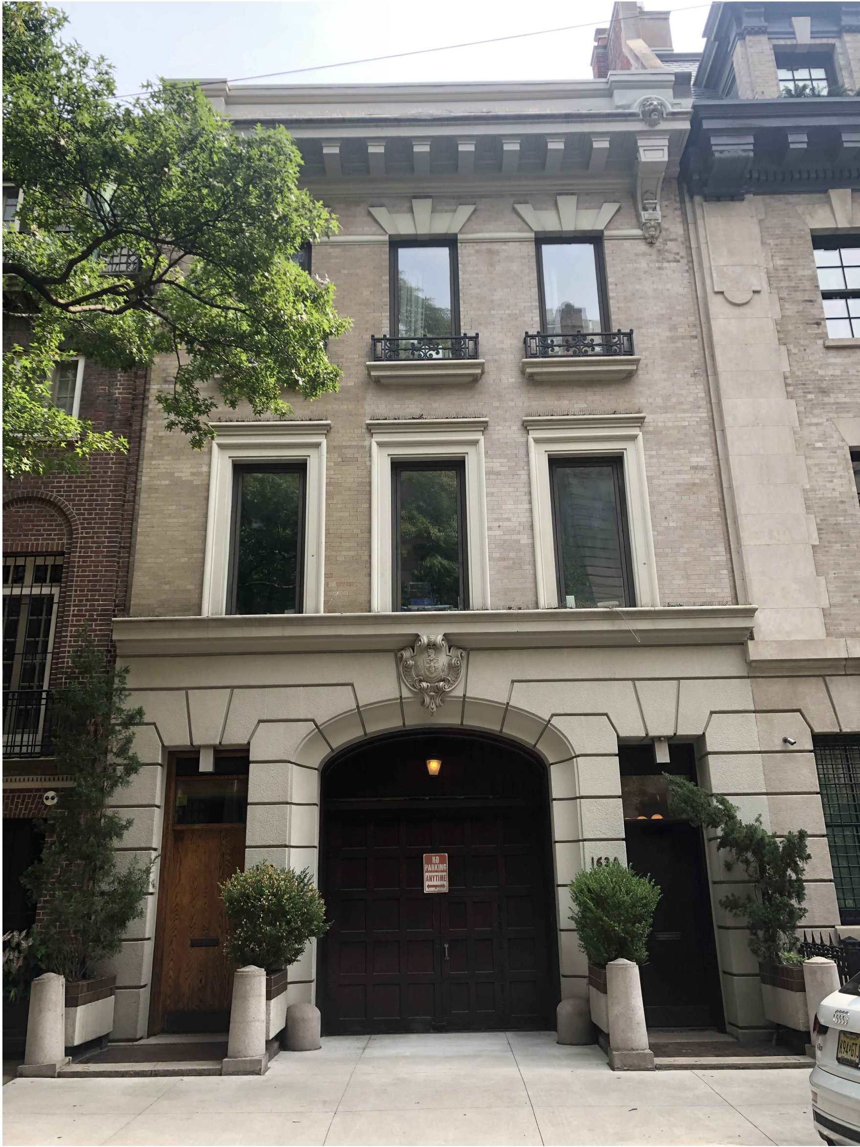
3 EXISTING BUILDING PHOTO EAST 70TH STREET FACADE
