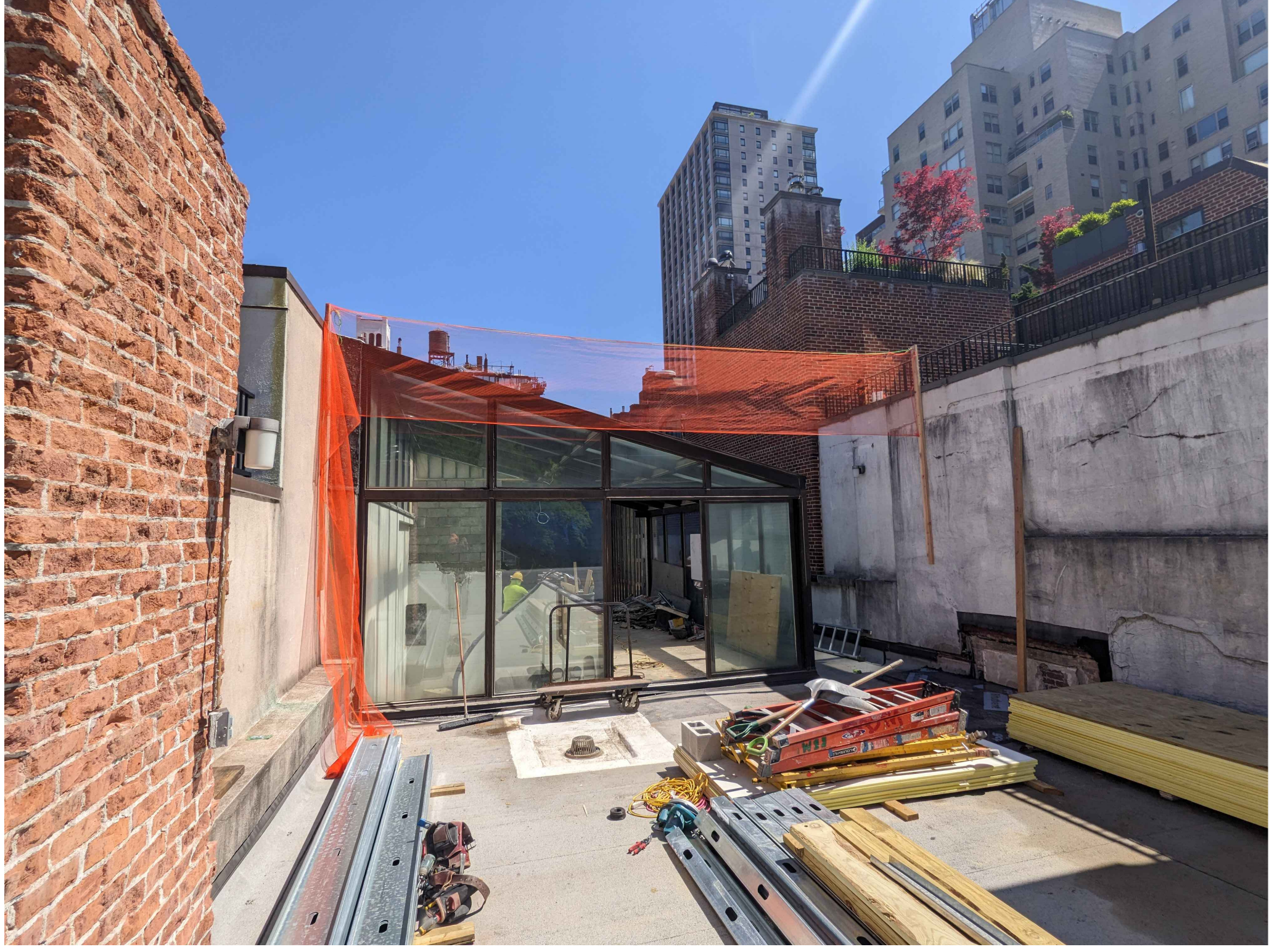
5 MOCKUP VIEW FROM ROOF
