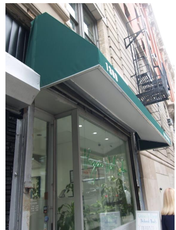
Awning at 1369 Madison Avenue has enclosed underside, with framed sides and skirt.
