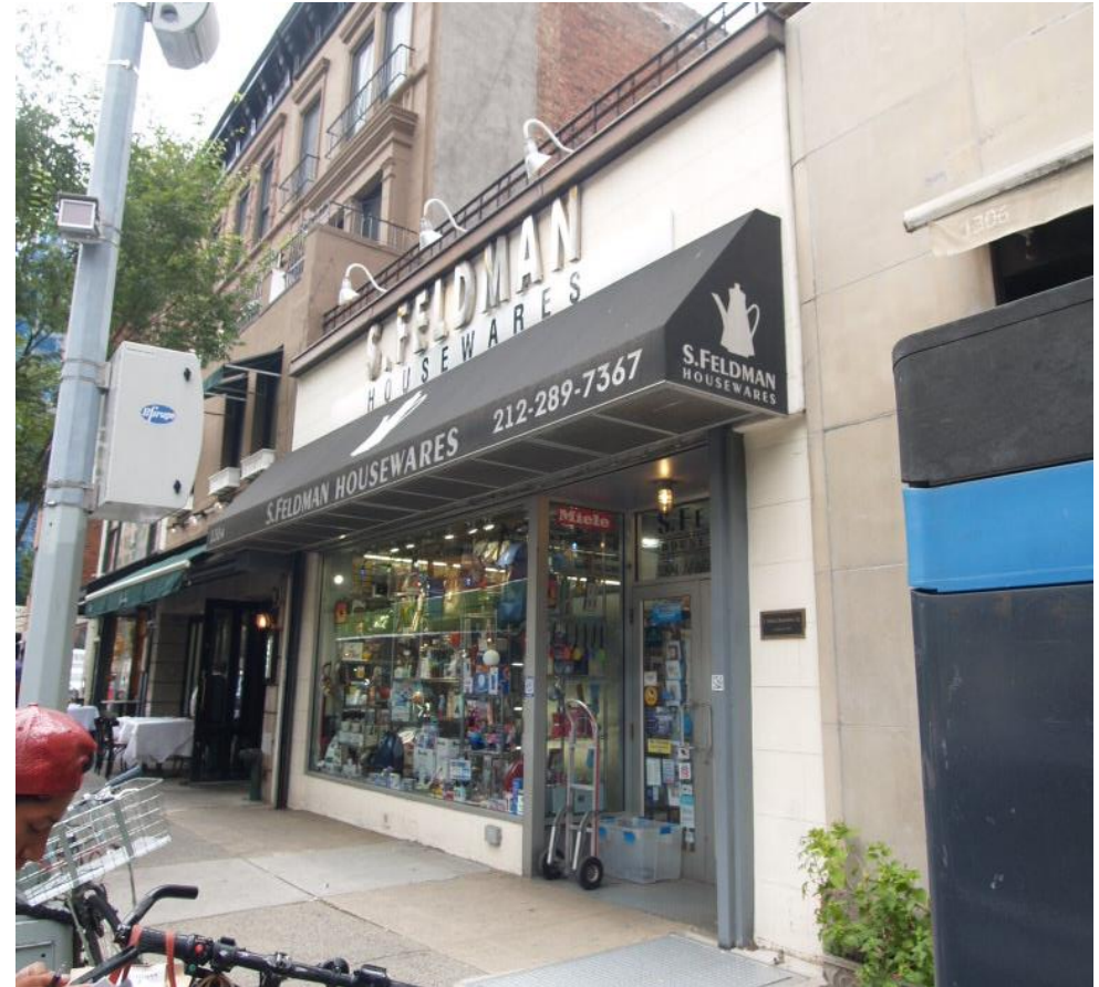
Awning at 1304 Madison Avenue has enclosed underside, with framed sides and skirt. The length of awning extends beyond the storefront opening.
