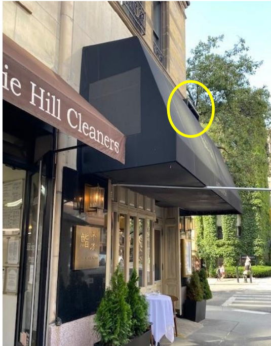
Details showing existing HVAC units with and without mesh enclosure at the underside of the awning. Also installed a small boxed area at top of awning to allow air intake/exhaust. The small vent is nearly invisible from the sidewalk.
