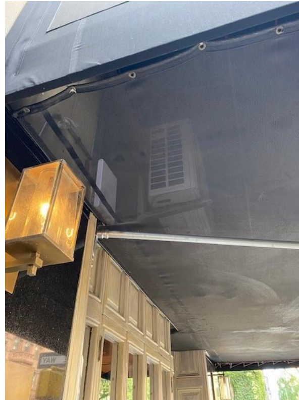
Details showing existing HVAC units with and without mesh enclosure at the underside of the awning. Also installed a small boxed area at top of awning to allow air intake/exhaust. The small vent is nearly invisible from the sidewalk.
