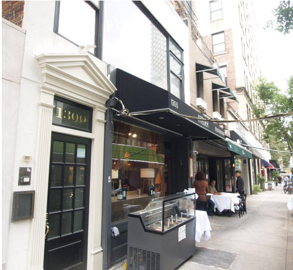
Awning at 1300 Madison Avenue has enclosed underside, with framed sides and skirt.
