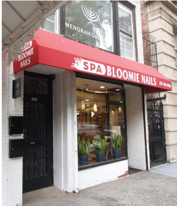
Awning at 1320 Madison Avenue has framed sides and skirt. The length of awning extends beyond storefront opening.
