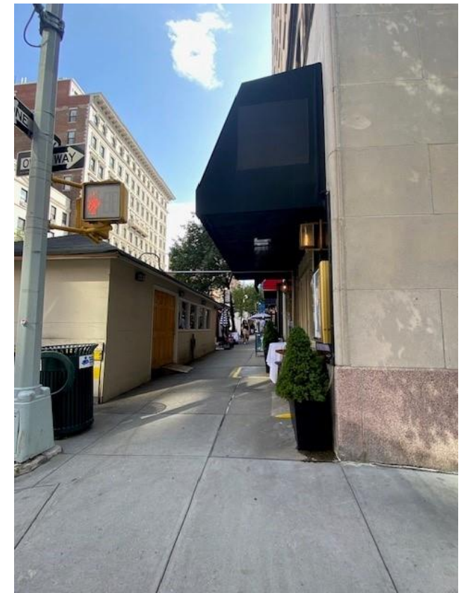
Profile got more boxy to enclose new HVAC units. Also added a fixed skirt, side panels, and mesh at underside
