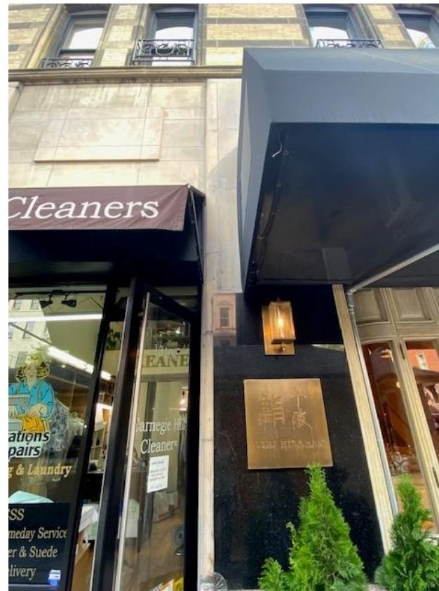
Frame extends beyond the storefront infill/opening and was elongated further from the prior condition.
