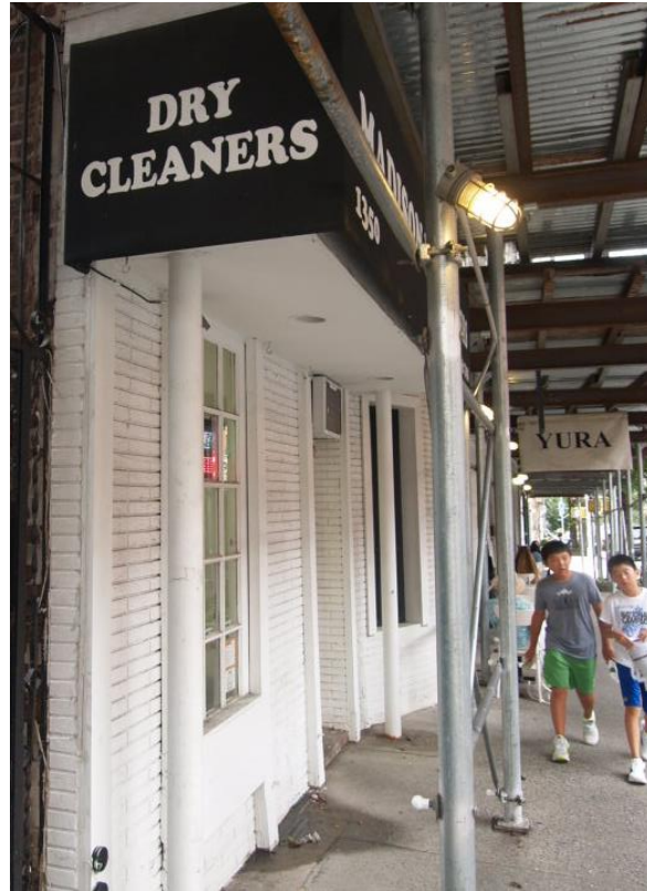
Awning at 1350 Madison Avenue has enclosed underside, with framed sides and skirt. The length of awning extends beyond storefront opening.
