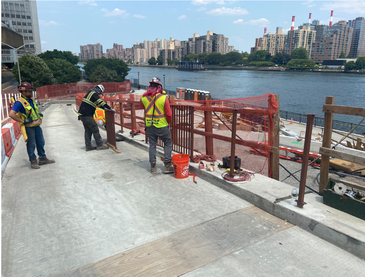
Installing picket fence
