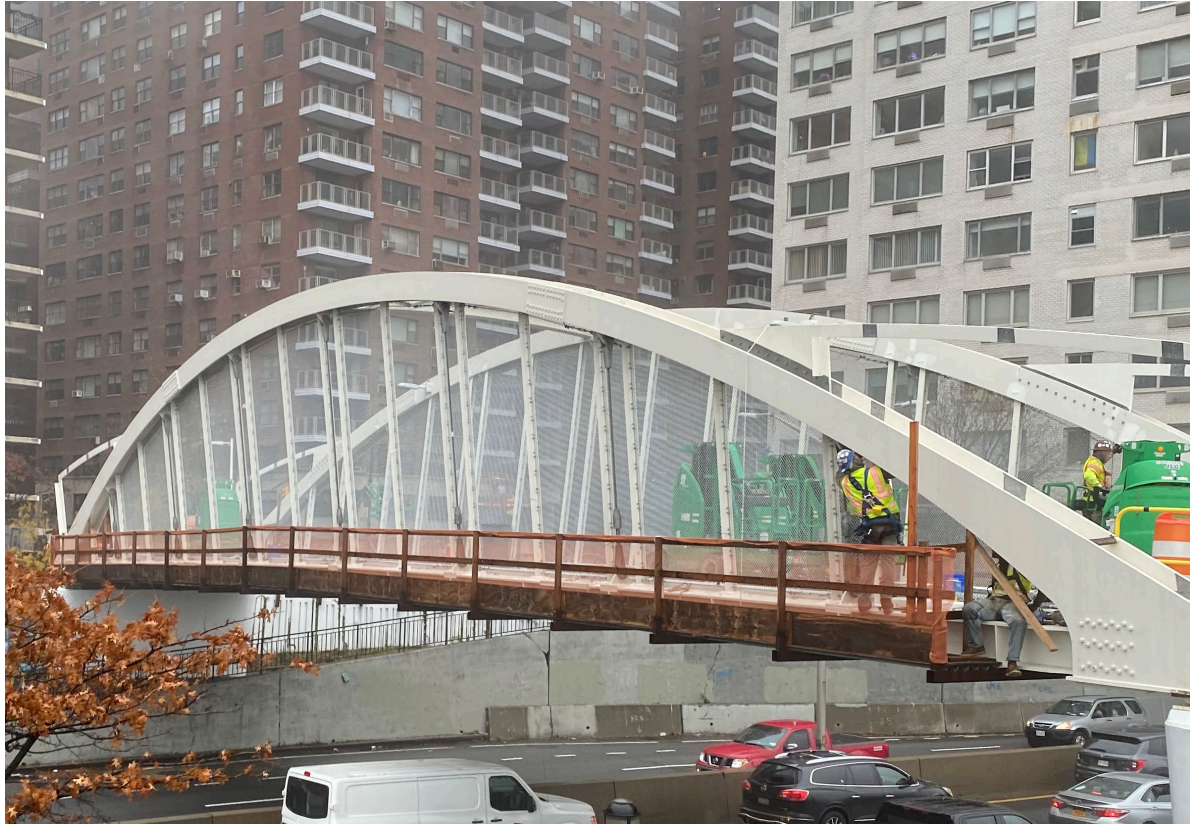
Installation of pedestrian bridge fencing
