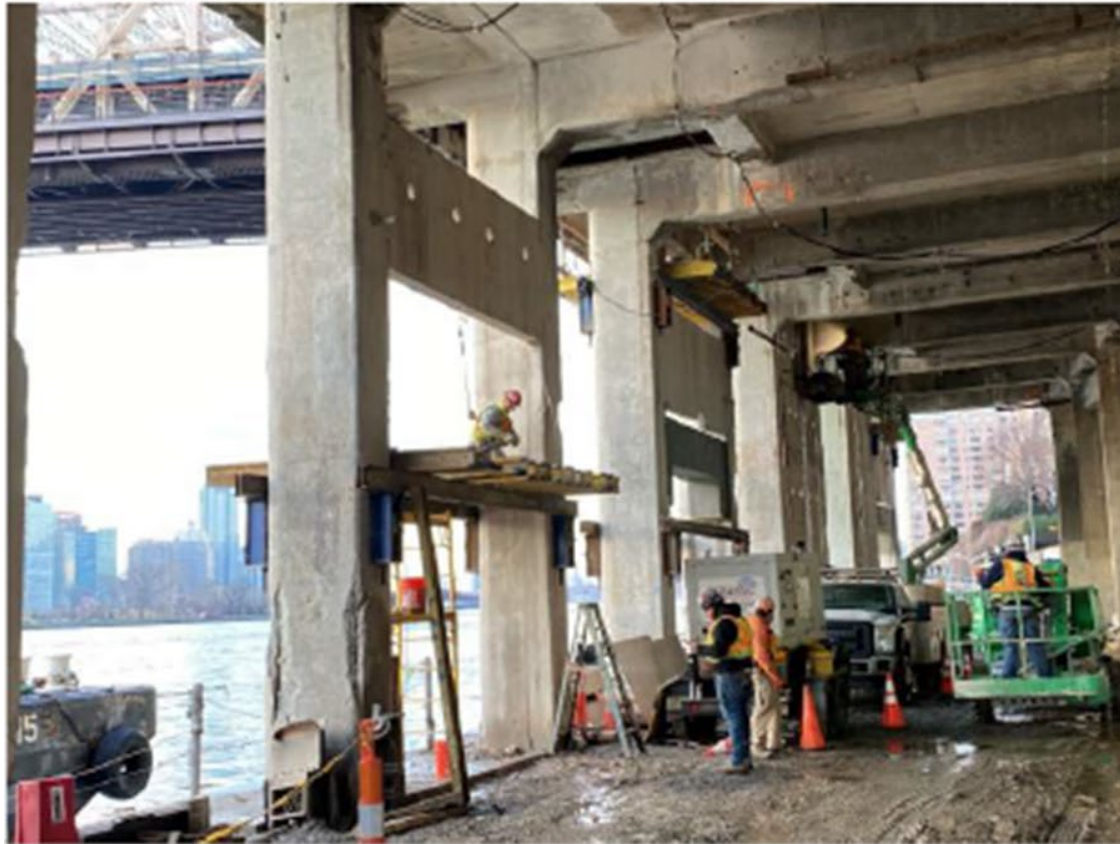
Concrete Curtain Wall removed under the Alice Aycock Pavilion
