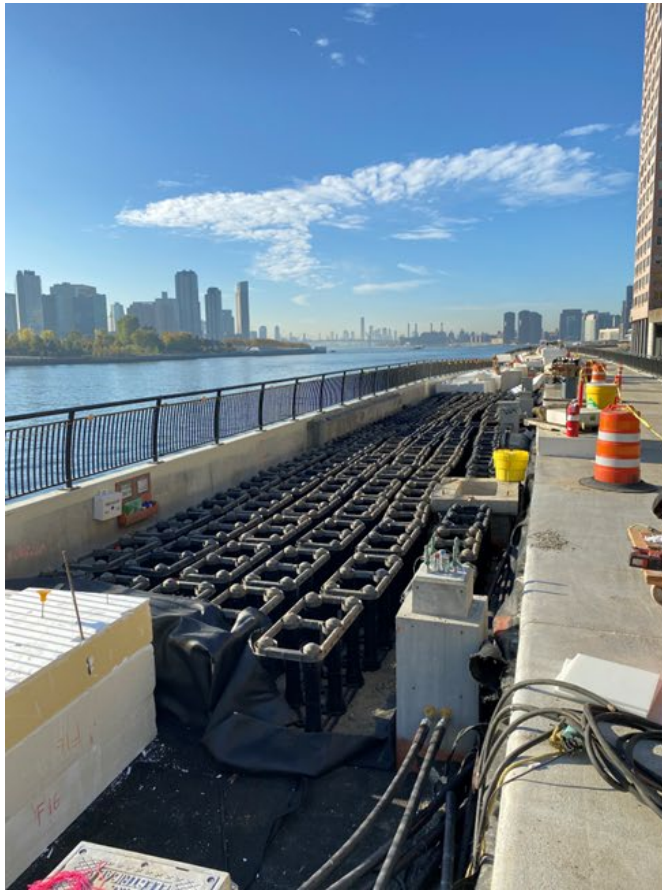
Placement of Silva Cells
