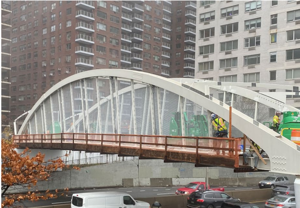
Installation of pedestrian bridge fencing
