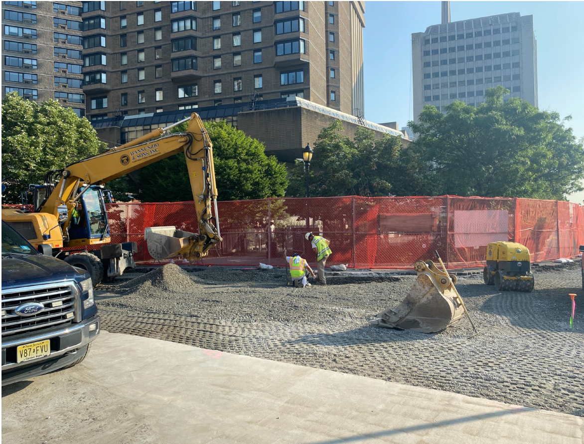
Repaving and paver preparation work along the East River
