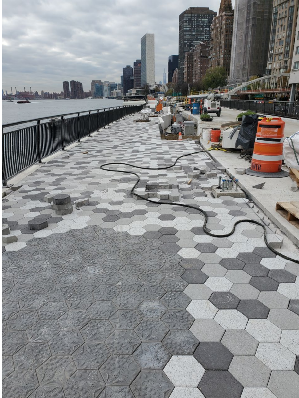
Standard pavers and artwork paver installed
