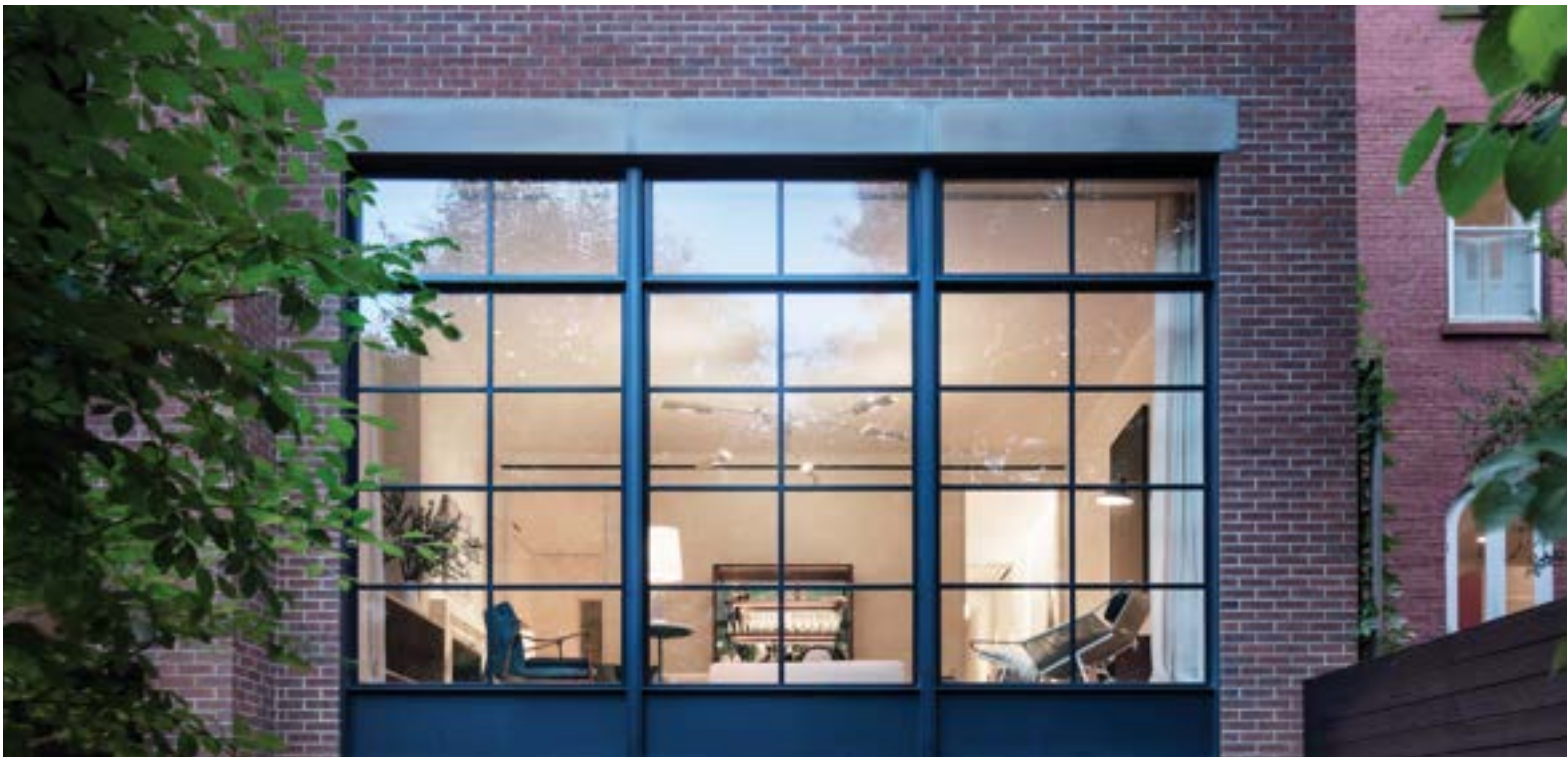
Steel Windows on Rear Penthouse
