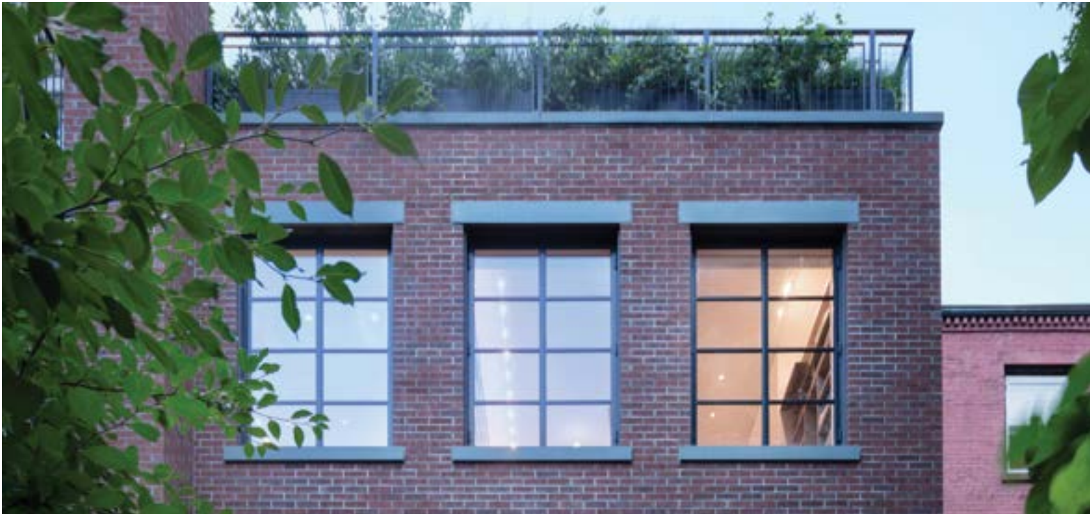
Steel Windows on Rear Facade
