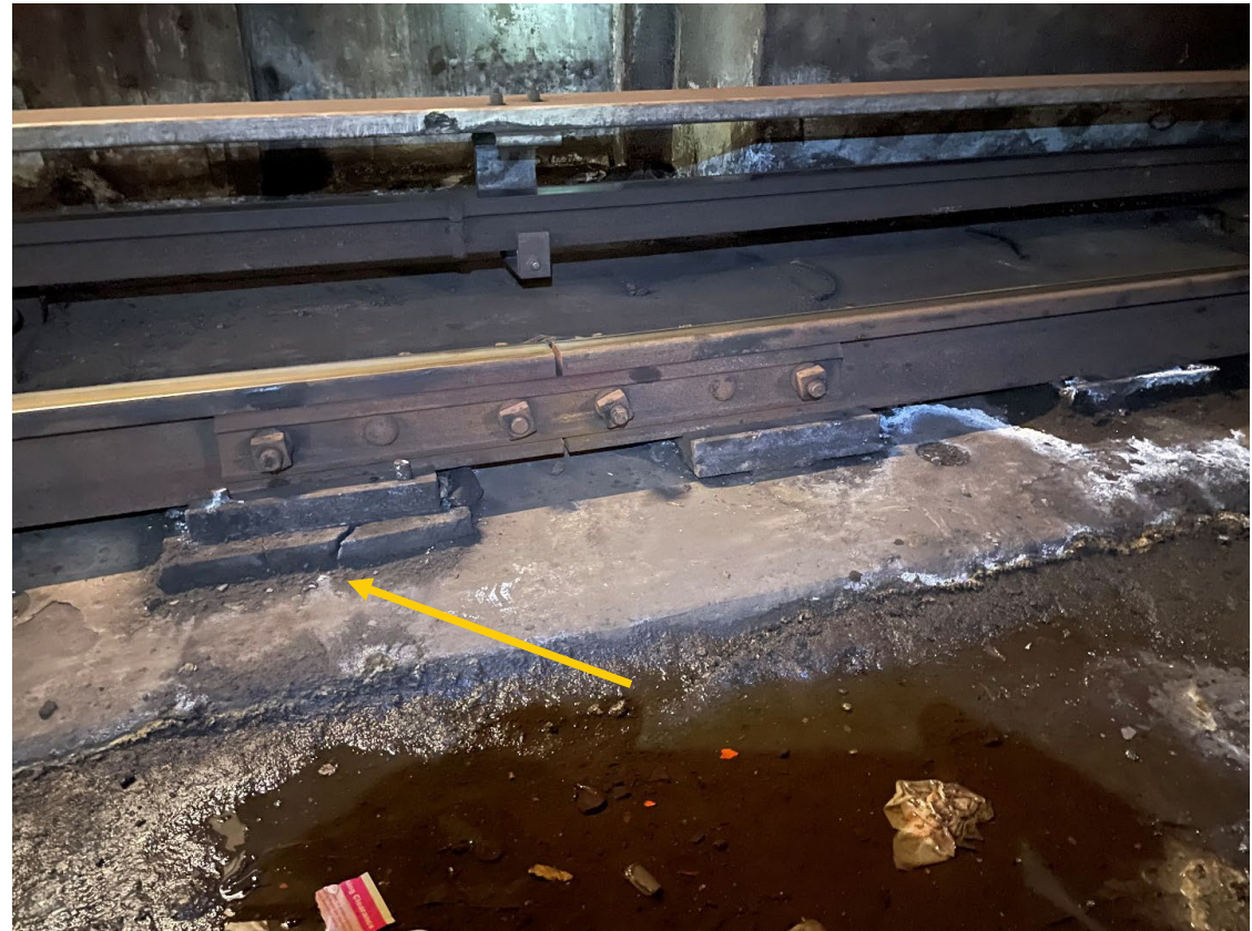
Above: Deteriorated concrete plinth supporting rail on 63 St Line
