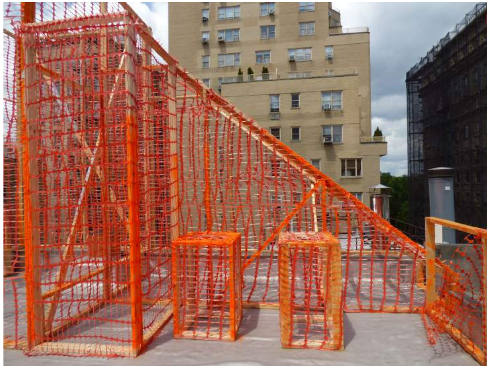
4 | Stair bulkhead, looking west
