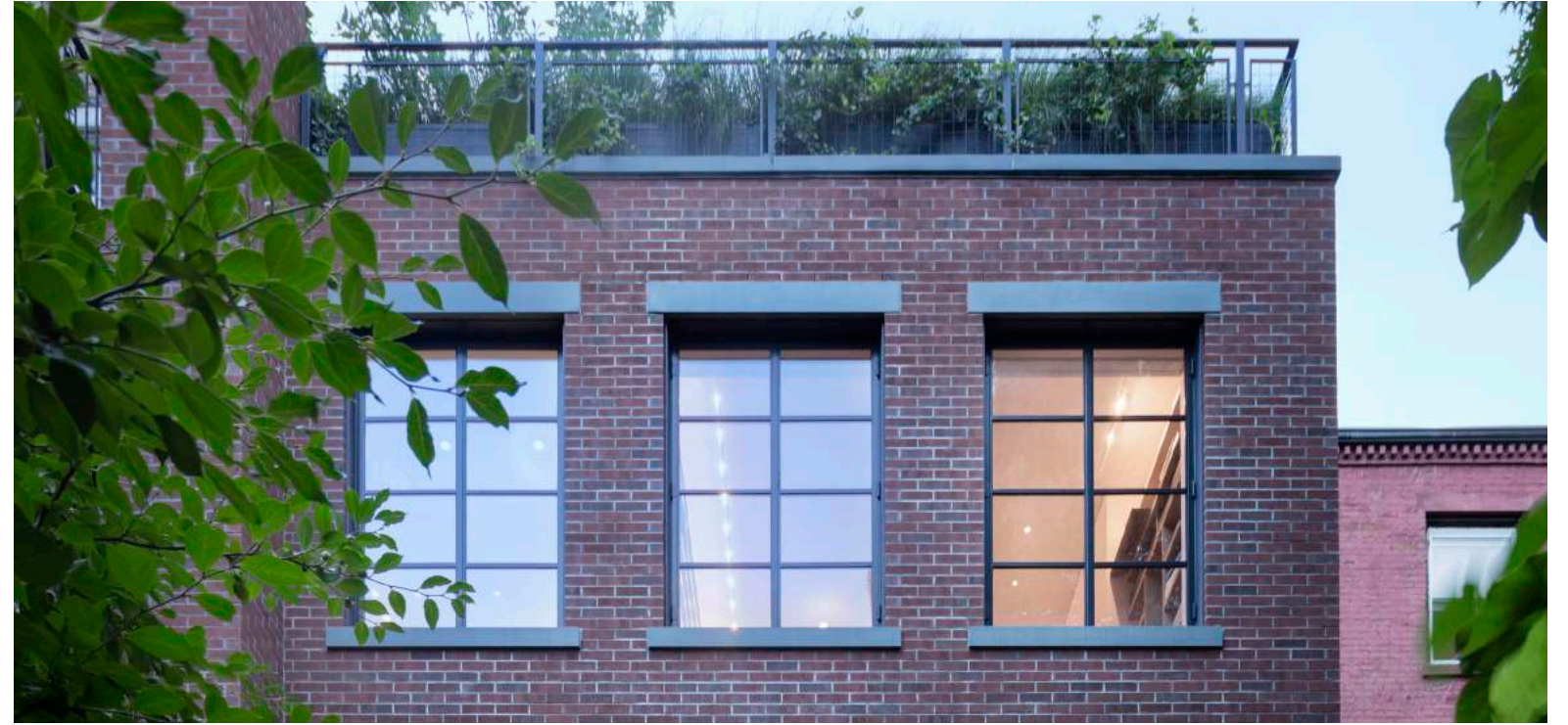
Steel Windows on Rear Facade
