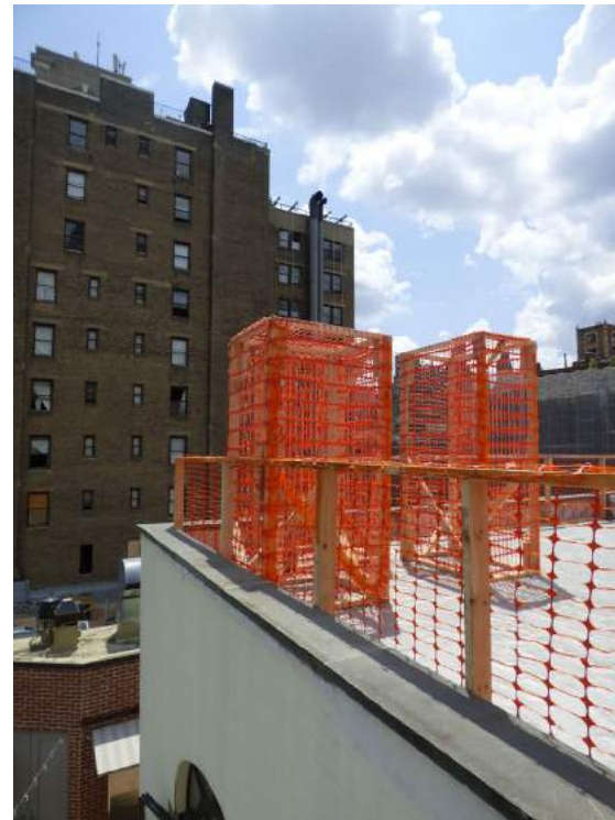
5 | Mechanical units and railing, looking east
