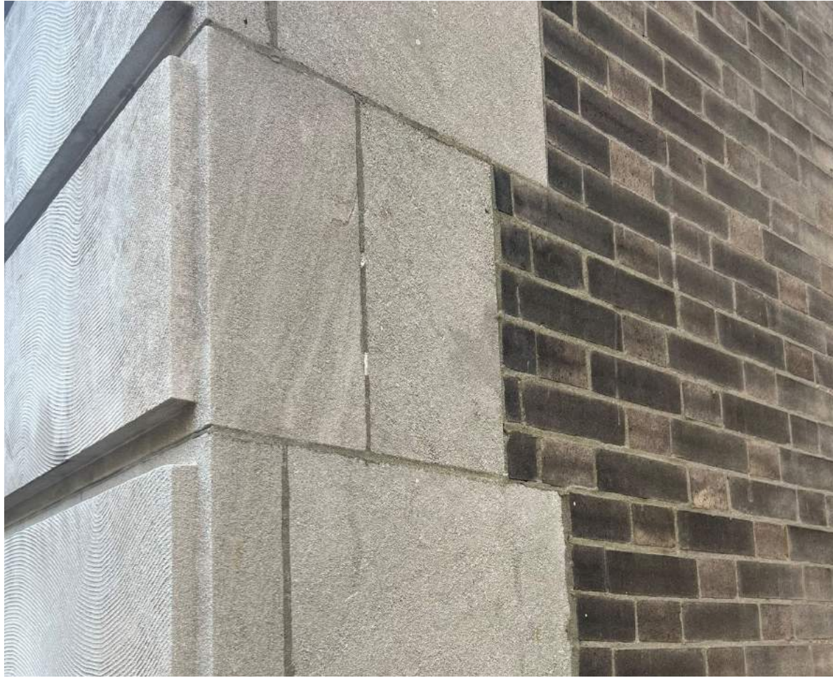
Street Facade Masonry
