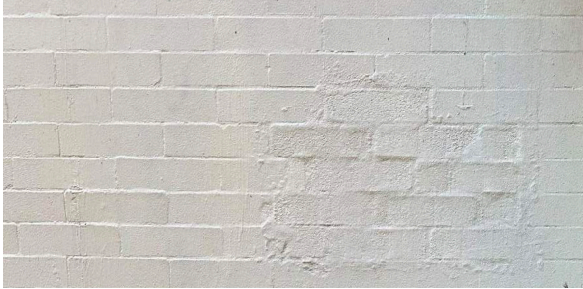
Rear Facade Masonry
