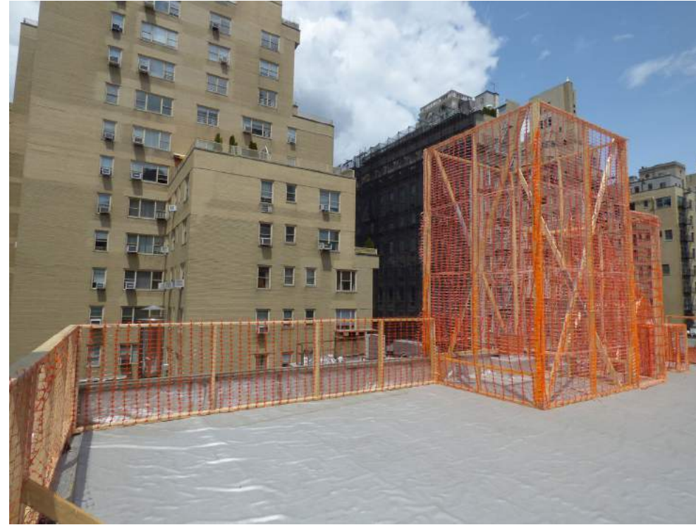
2 | Railing and elevator bulkhead, looking northwest
