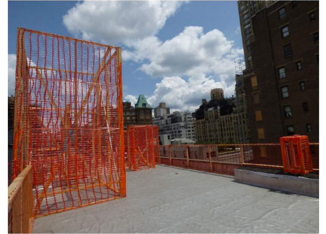
3 | Elevator bulkhead (at left), chimney extension (at right), mechanical (center), and railing, looking north
