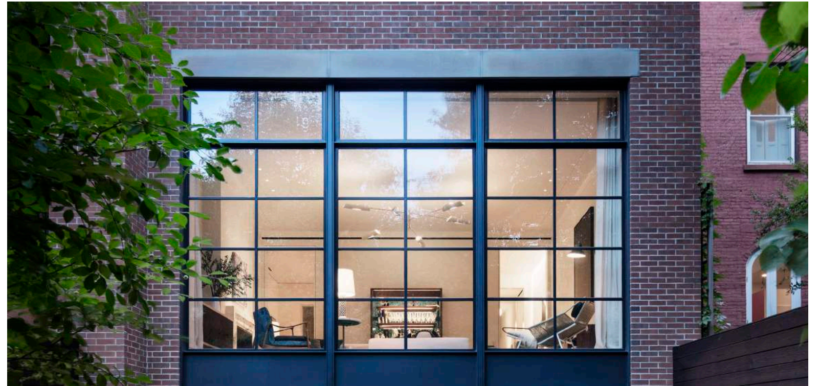
Steel Windows on Rear Penthouse
