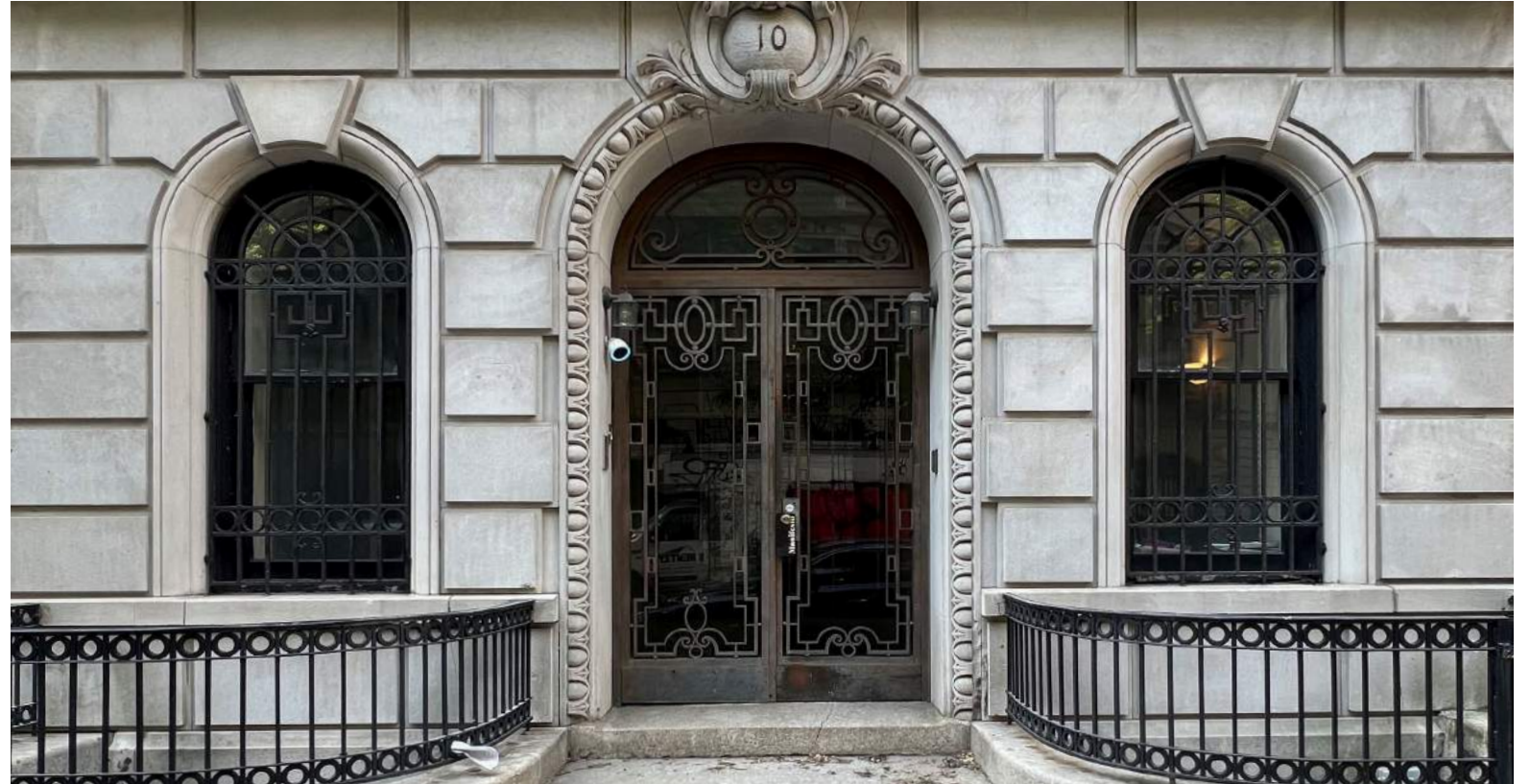
Lower Windows on Front Facade
