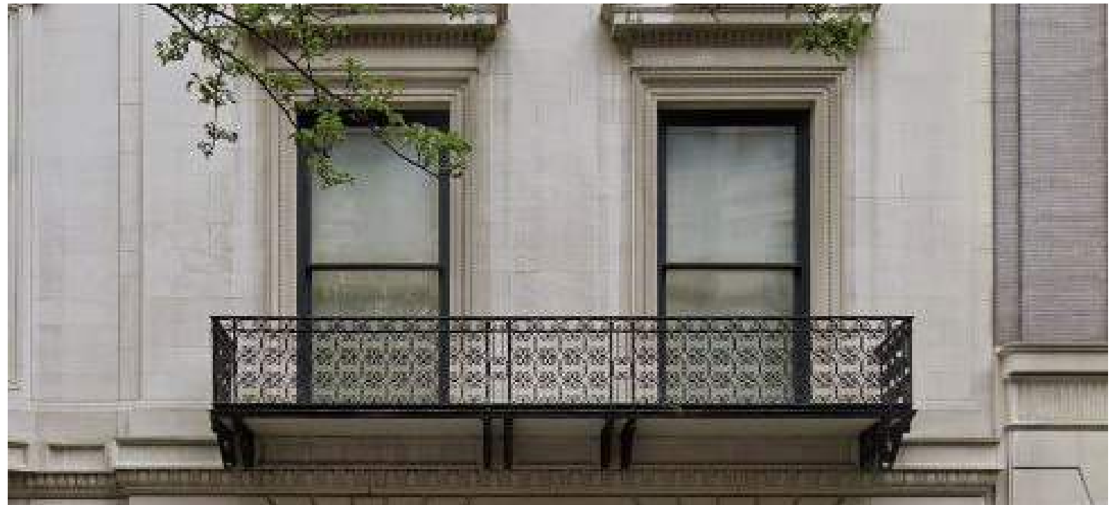
Upper Windows on Front Facade
