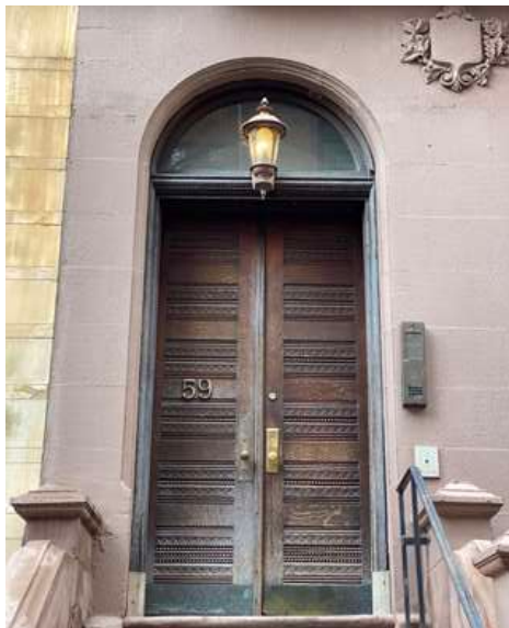
Wooden Door and Stone Crest
