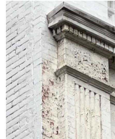
Paint Colors on Front Facade
