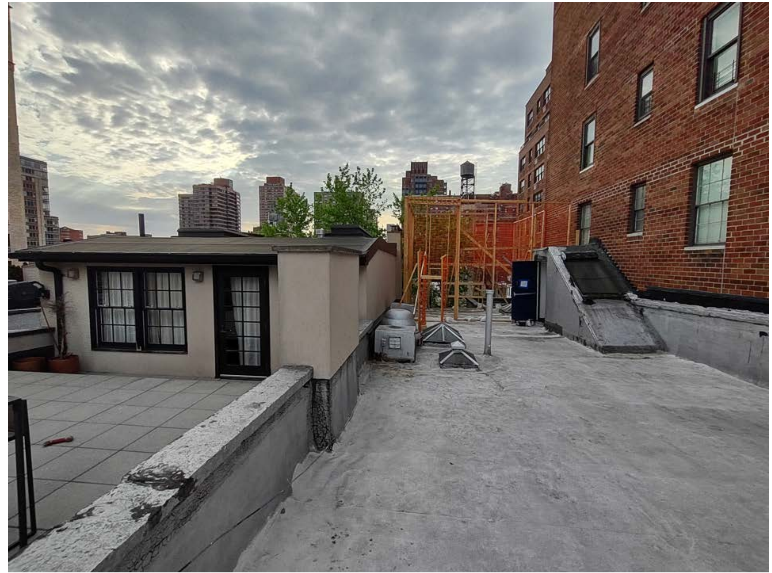
ROOFTOP, LOOKING EAST.
