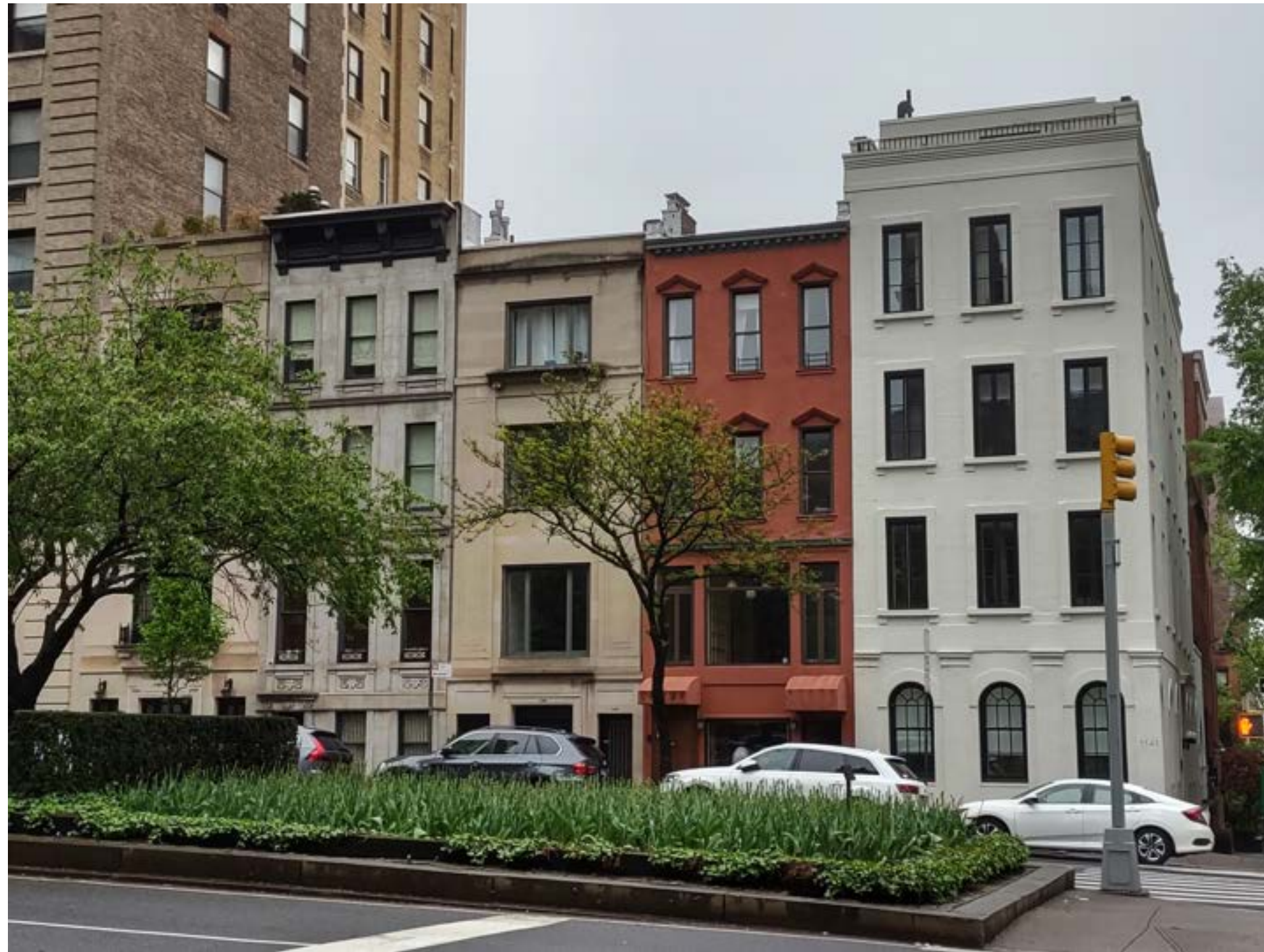
1141 - 1149 PARK AVENUE, VIEWED FROM THE WEST SIDE OF PARK AVENUE AT EAST 91ST ST. ROOFTOP ADDITION AT 1141 IS VISIBLE (MAY 2023)
