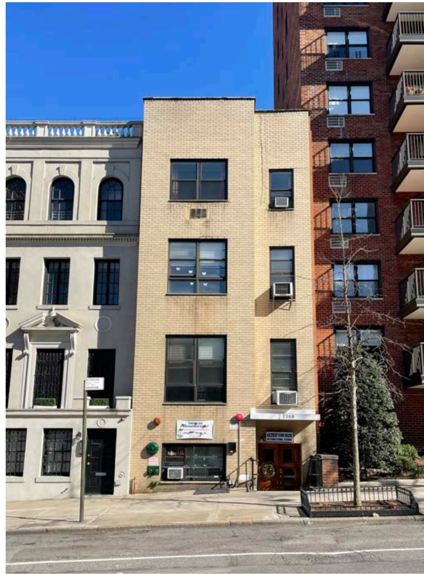
EXISTING FRONT FACADE
