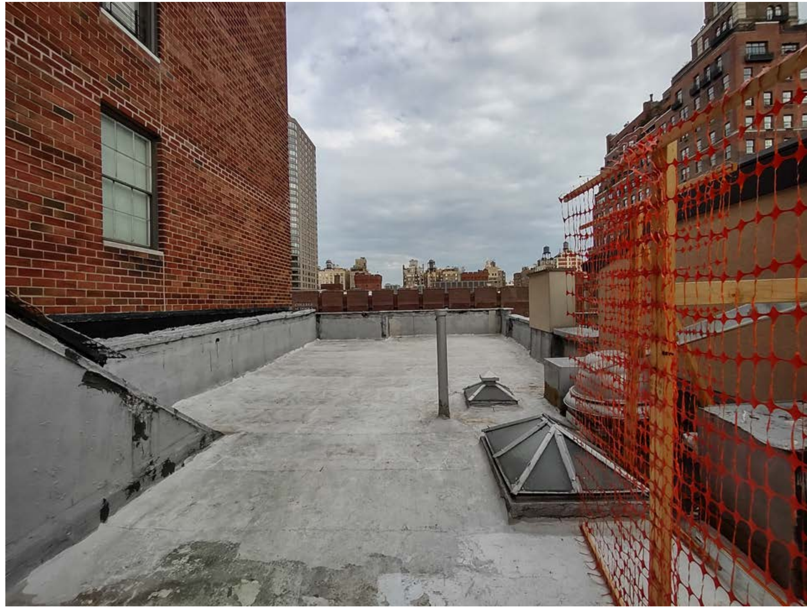
ROOFTOP, LOOKING WEST.
