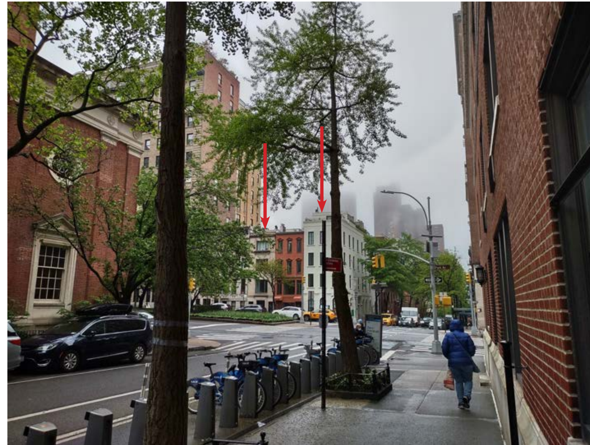
1141 - 1149 PARK AVENUE, VIEWED FROM THE WEST ON EAST 91ST ST. ROOFTOP ADDITIONS AT 1141 AND 1145 ARE VISIBLE (MAY 2023)
