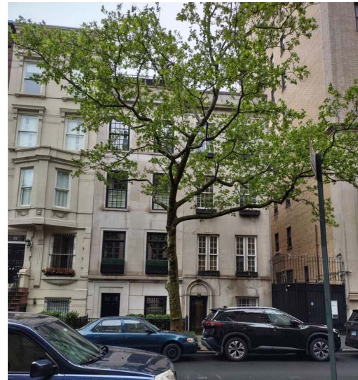
63 AND 65 EAST 92ND ST. VIEWED FROM ACROSS THE STREET. ROOFTOP ADDITIONS ARE NOT VISIBLE (MAY 2023)
