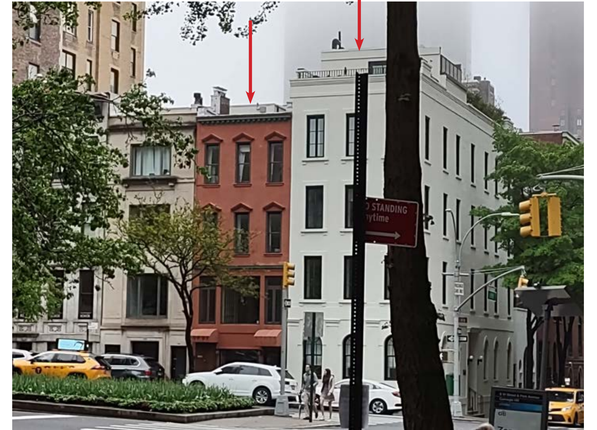
1141 - 1149 PARK AVENUE, ZOOMED IN VIEW FROM DOWN EAST 91ST ST. ROOFTOP ADDITIONS AT 1141 AND 1145 PARK AVENUE ARE VISIBLE (MAY 2023)
