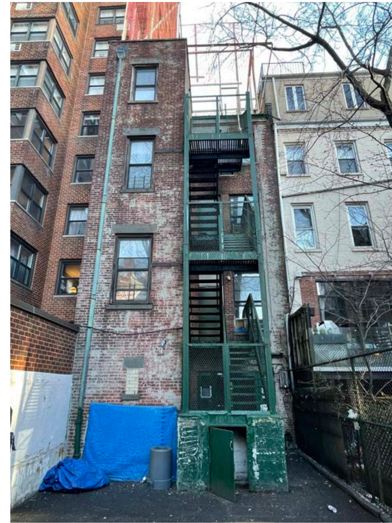
EXISTING REAR FACADE
