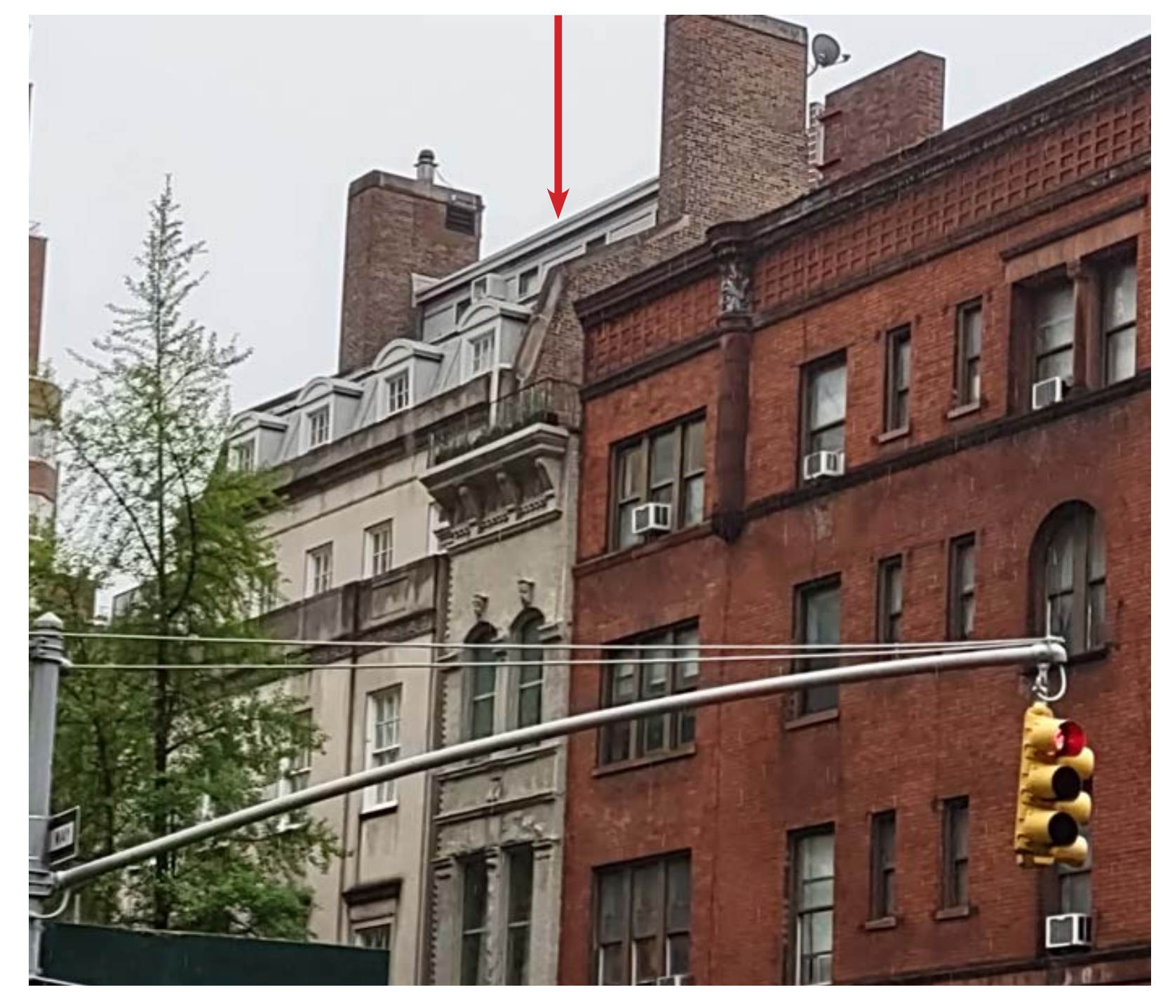
48 EAST 92ND ST. ZOOMED IN VIEW FROM MADISON AVENUE. ROOFTOP ADDITION IS VISIBLE. (MAY 2023)
