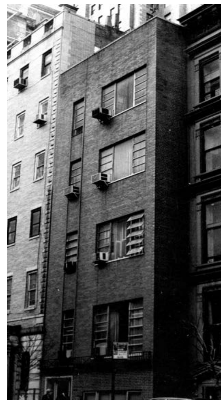
7 EAST 63RD ST. - DESIGNATION PHOTO UPPER EAST SIDE HISTORIC DISTRICT NO STYLE
