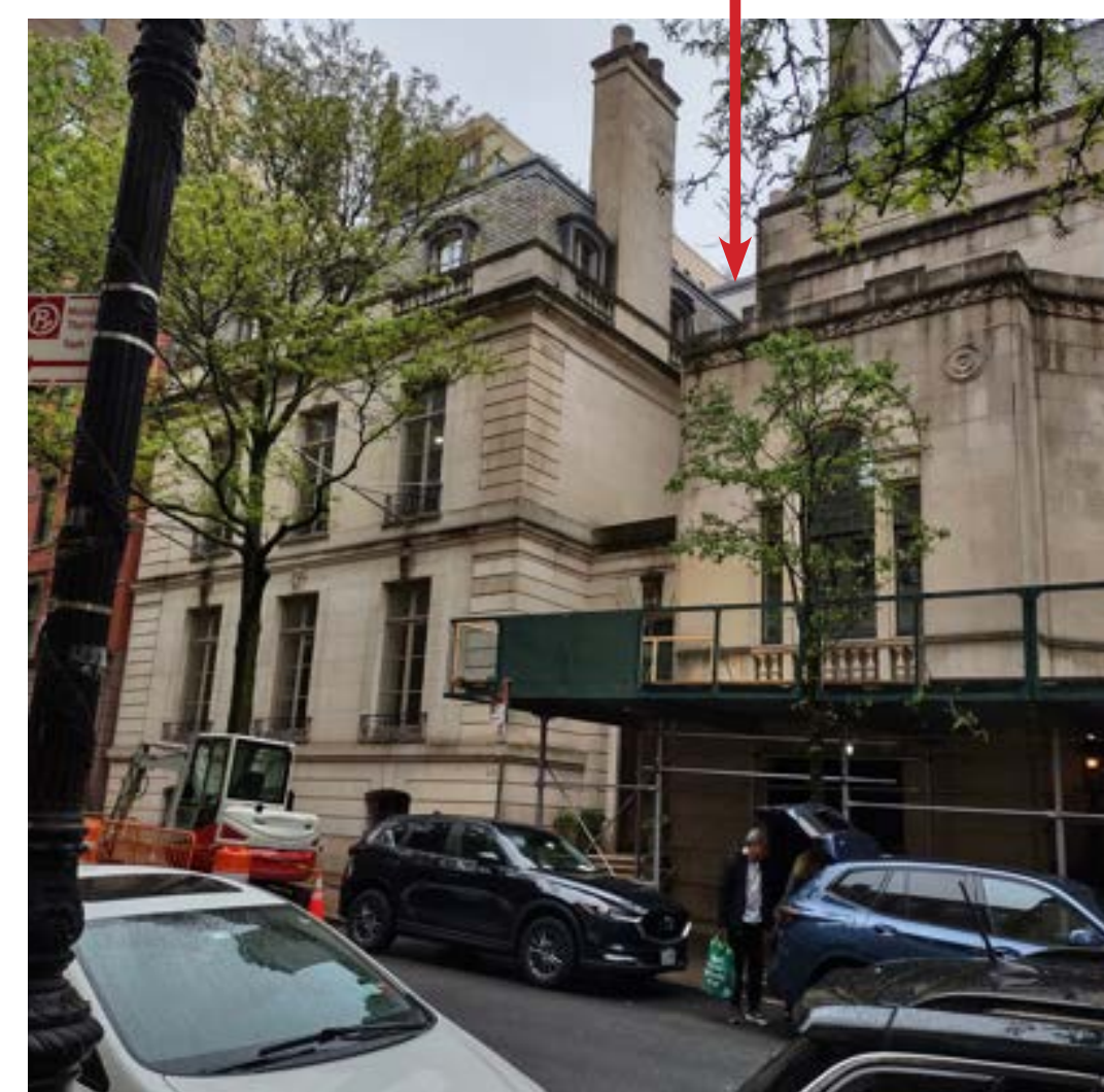
60 EAST 93RD ST. VIEWED FROM ACROSS THE STREET AND WALKING WEST. ROOFTOP ADDITIONS ARE VISIBLE (MAY 2023)
