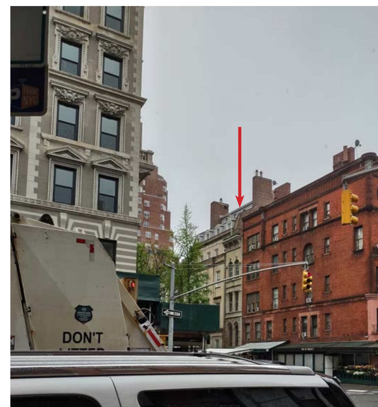
48 EAST 92ND ST. VIEWED FROM MADISON AVENUE. ROOFTOP ADDITION IS VISIBLE. (MAY 2023)
