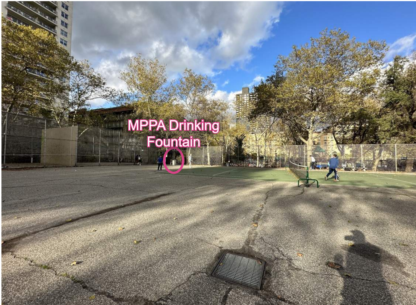
1 - MPPA with asphalt structural Damage. Drinking fountain in MPPA to be replaced with ADA approved Type “E” Hi-LO
