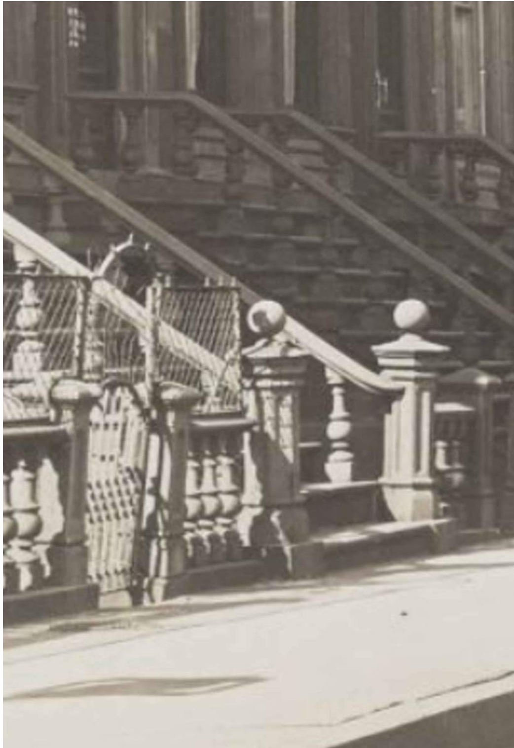
ENLARGEMENT OF 1912 PHOTOGRAPH SHOWING CAST IRON RAILINGS AT STOOPS ALONG 74TH STREET
