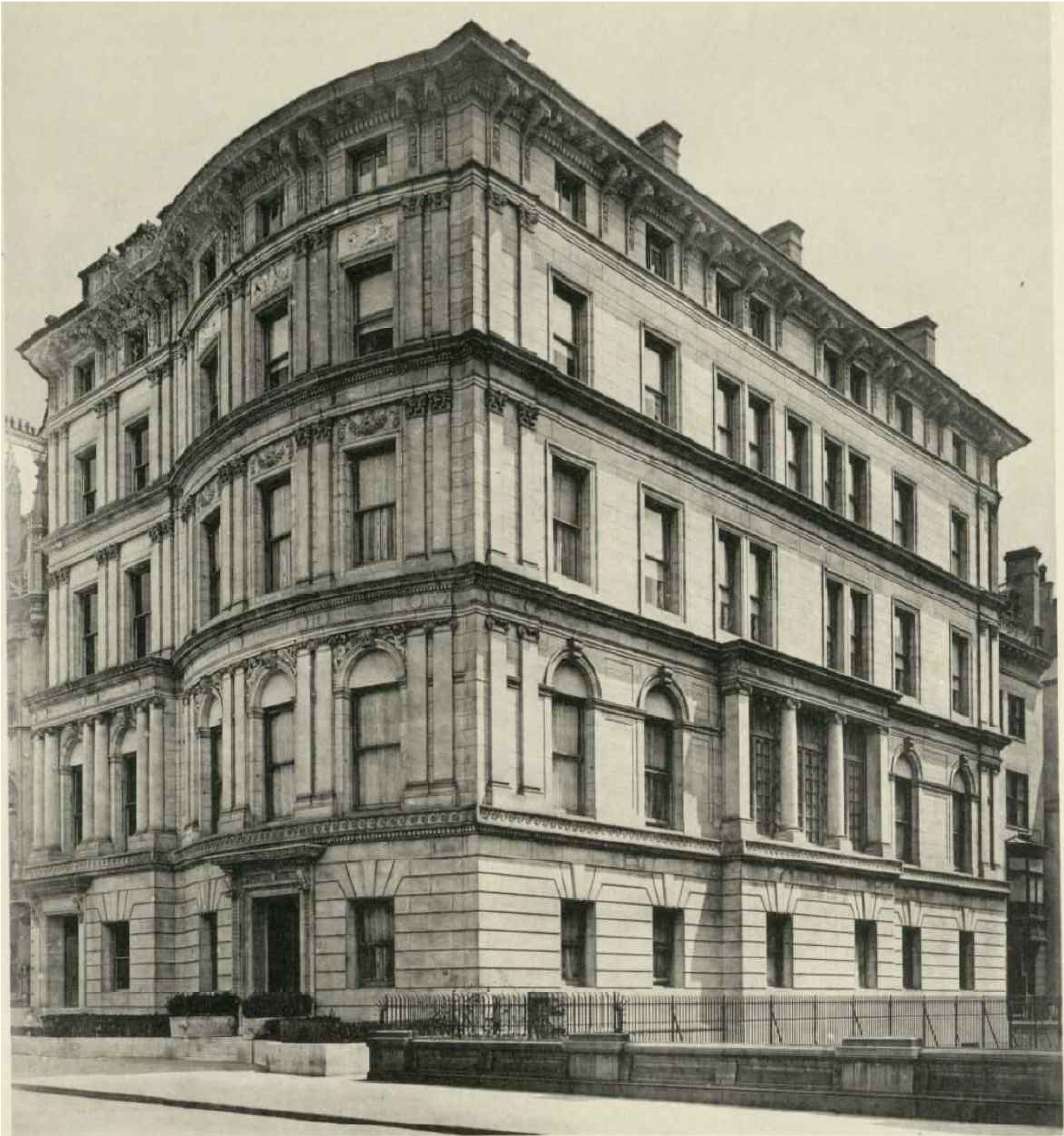
1 972 FIFTH AVENUE – HISTORIC PHOTOGRAPH AFTER CONSTRUCTION (“THE MONOGRAPH”, MCKIM, MEAD & WHITE, PLATE 290) SCALE: N.T.S.
