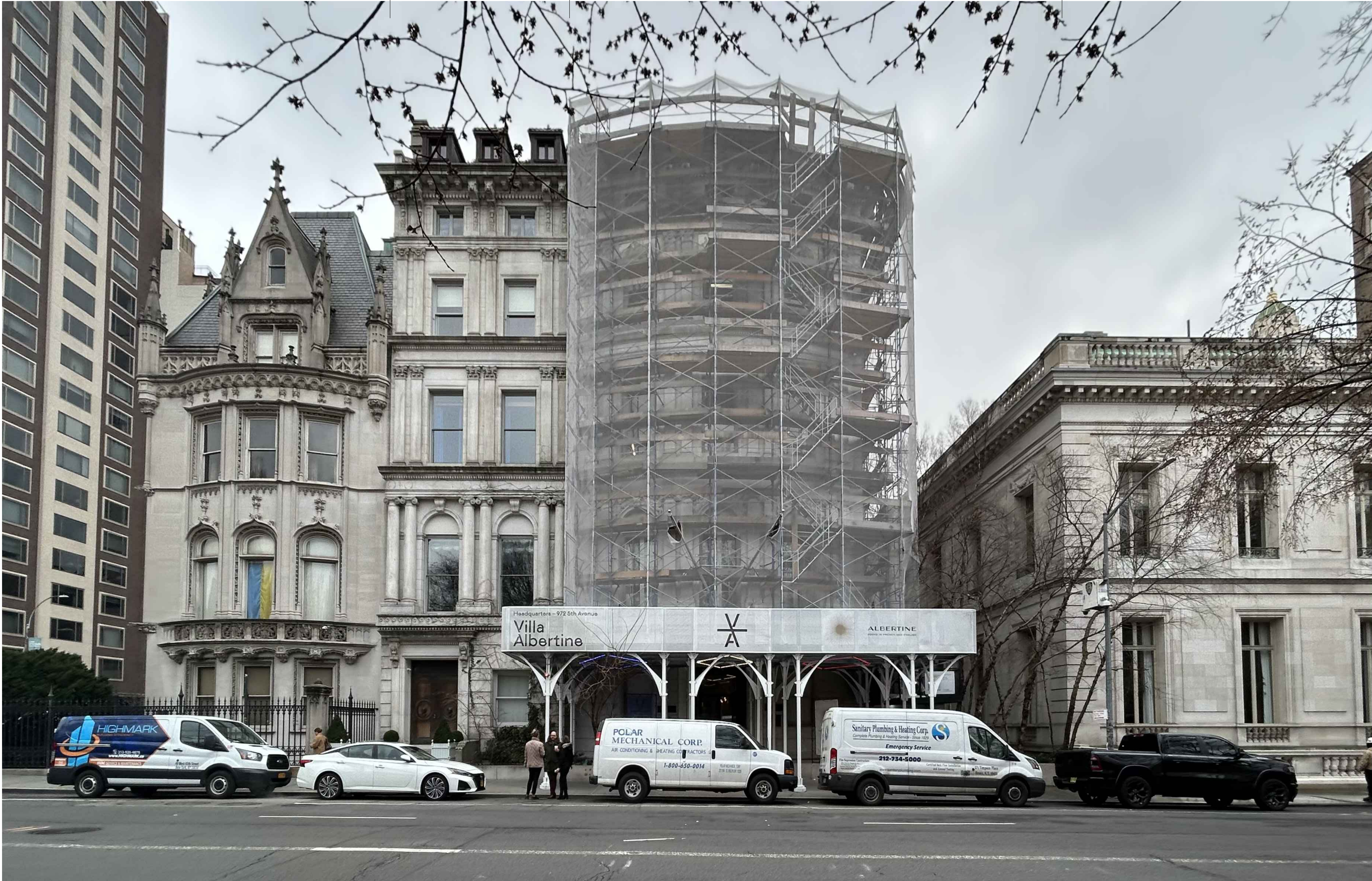
PHOTO DATED FEBRUARY 21ST, 2023. EXTERIOR FACADES AND WINDOWS ARE CURRENTLY BEING RESTORED UNDER DOCKET #LPC-21-09691
