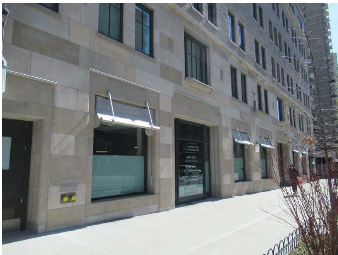
16. View of the ground floor retail facing south from Second Avenue.
