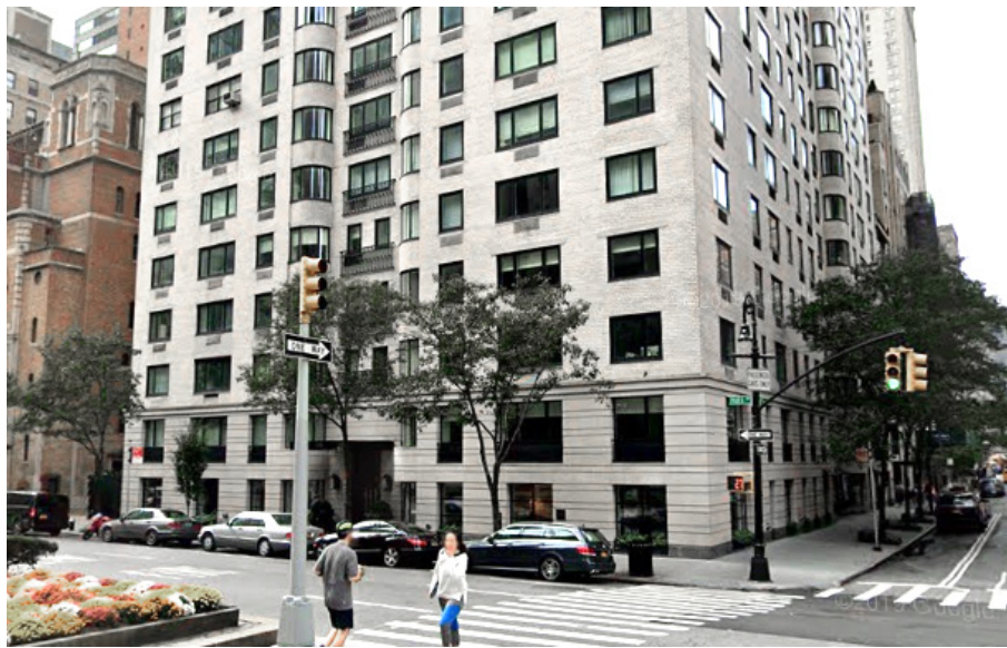
Park Avenue and 61st Street (530 Park Avenue) Two story base expression added; entry on Park; no commercial.
