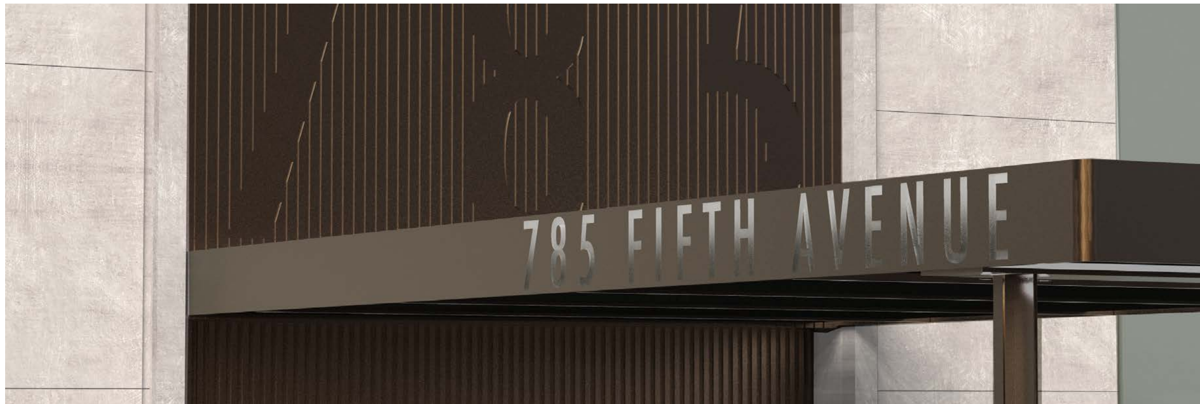
Canopy address in backlit sandblasted glass and cut-out characters and spandrel with large address numbers incised into ribbed pattern
