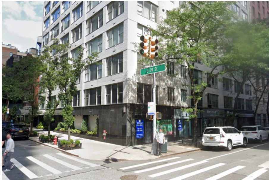
3rd Avenue and 69th Street (169 E 69th st) Single base expression; commercial on Ave. and entry on Street.
