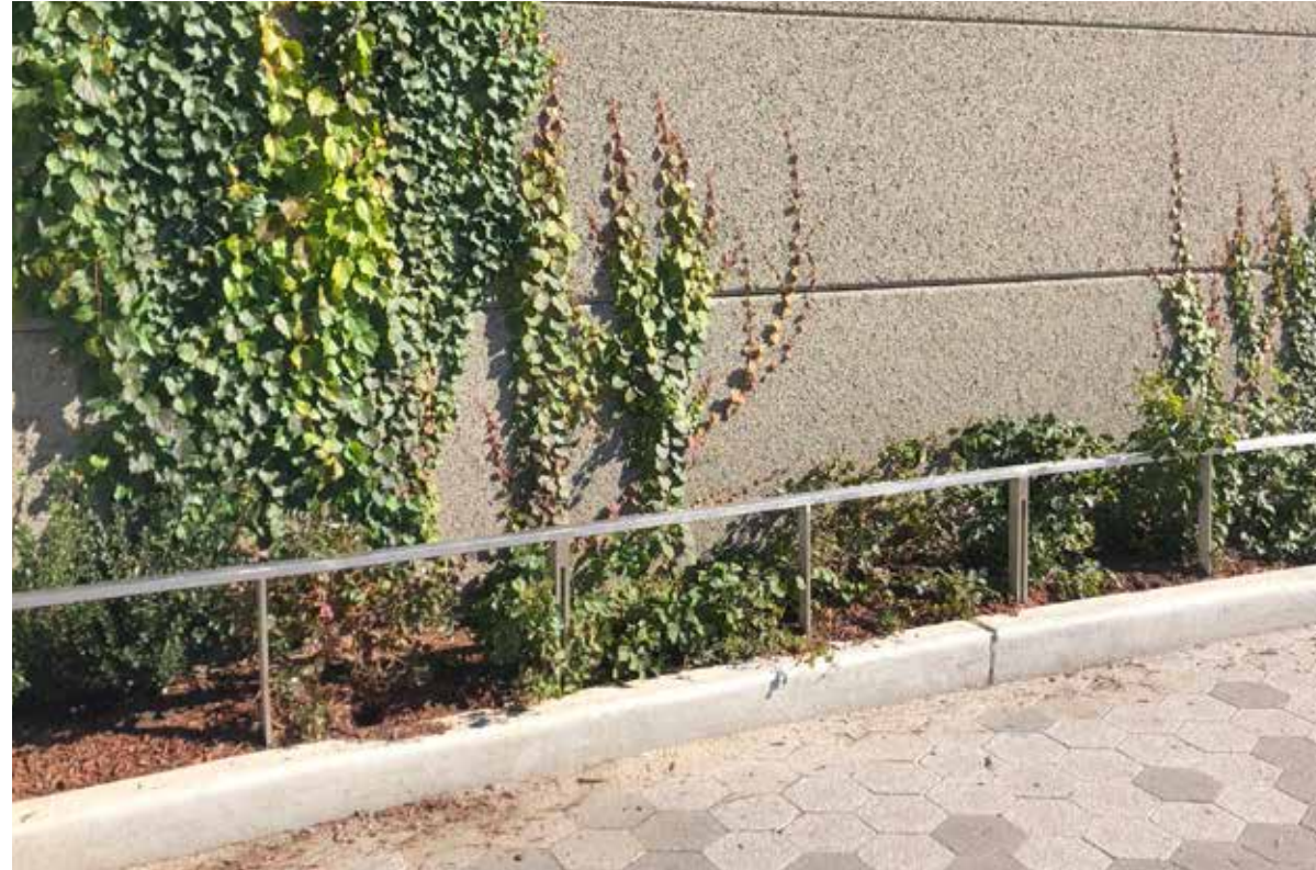
Revision: Stainless steel fence at planting beds
