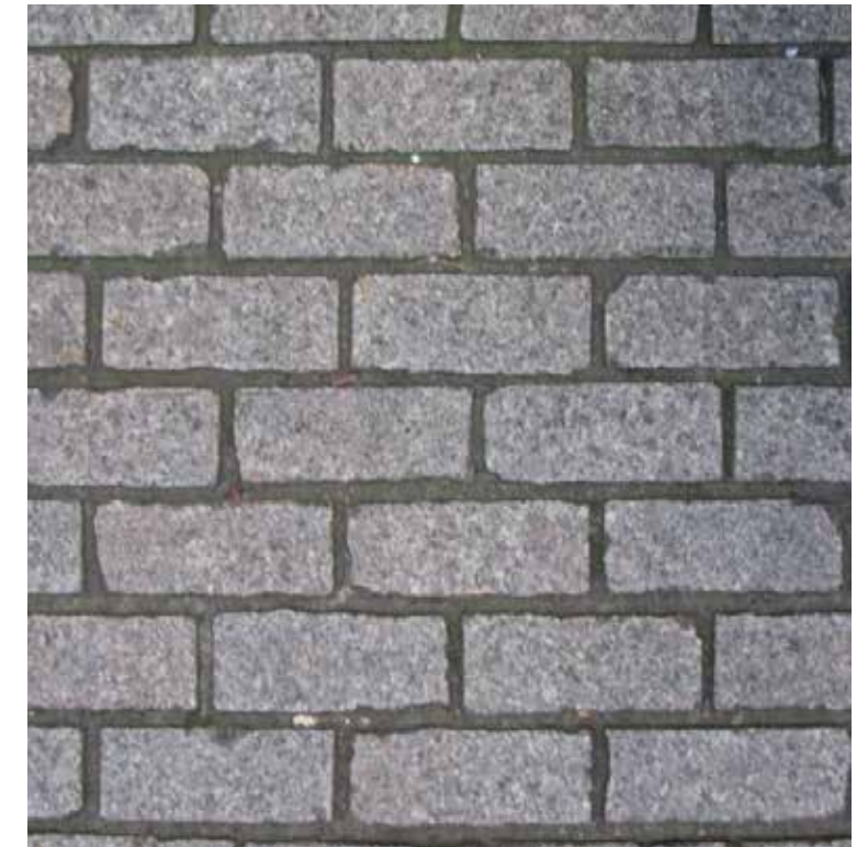
ADA Granite block pavers in running bond pattern (shown for finish and pattern only)
