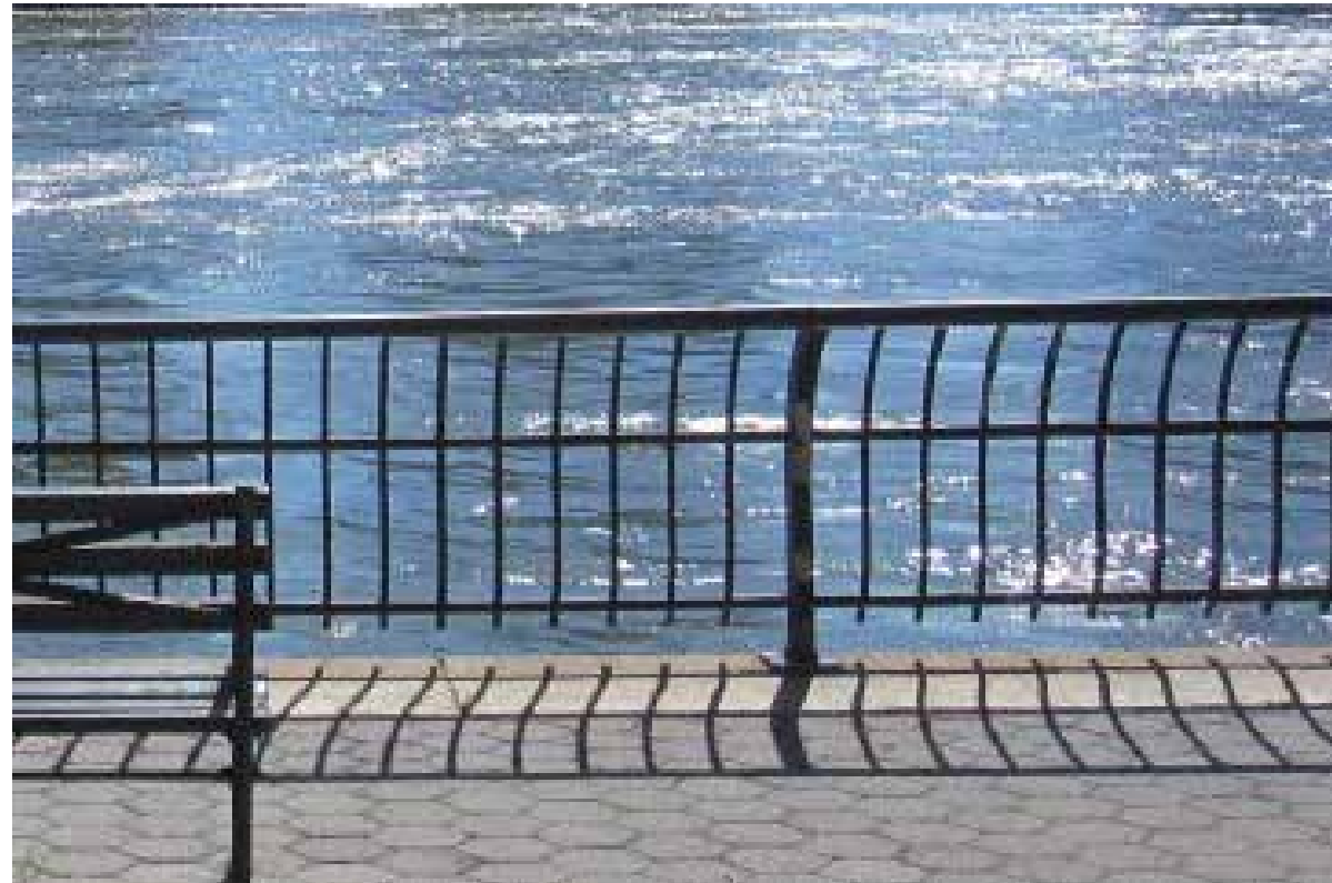
Existing bulkhead - Bow railing (refurbished)
