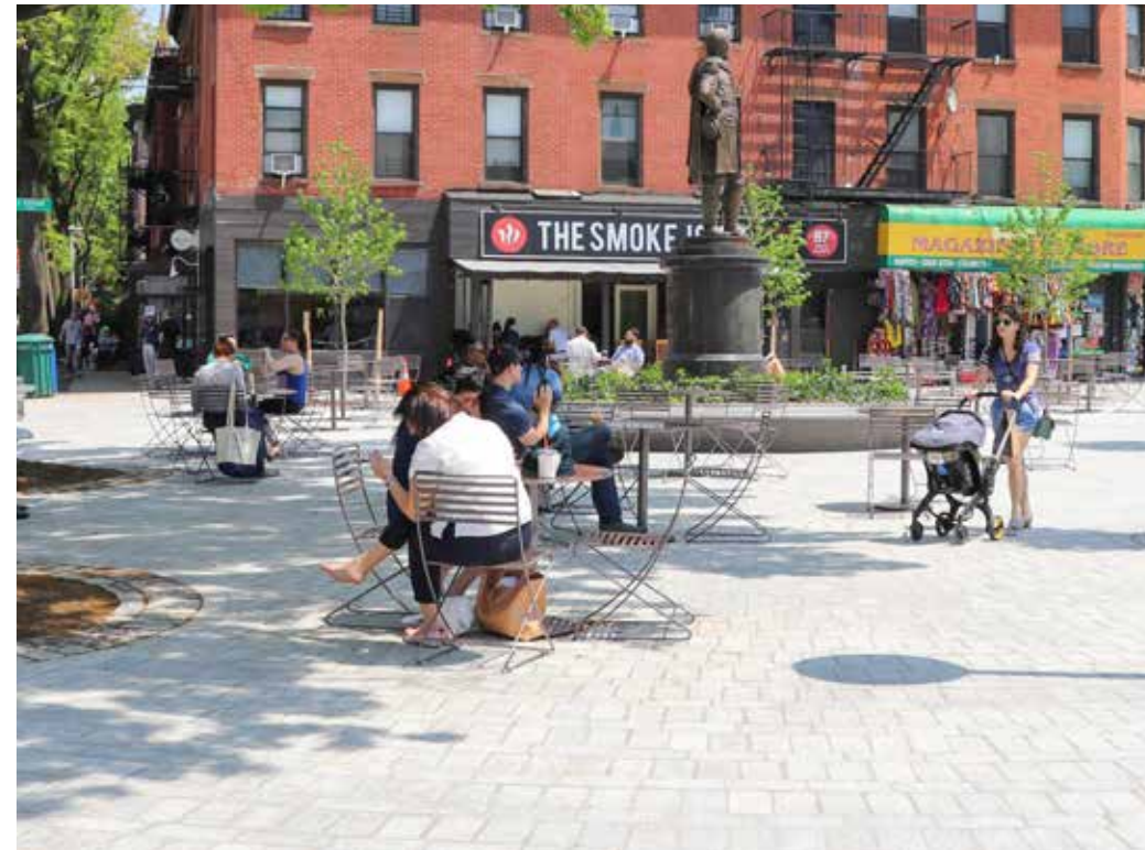
ADA Granite block paving at seating area and pedestrian pathway
