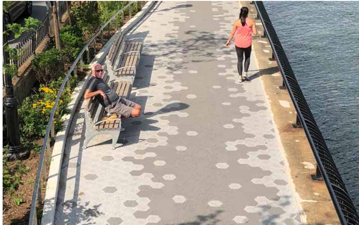
Asphalt hex block paving
