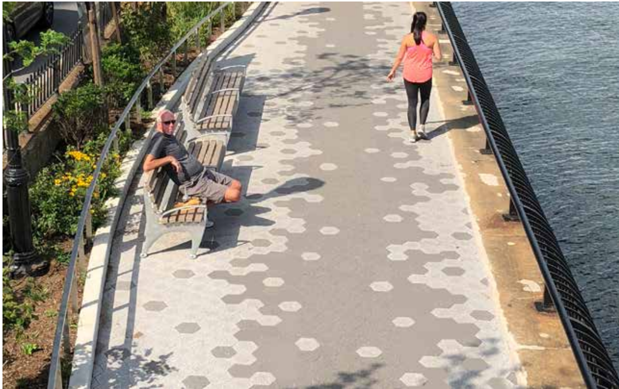
Asphalt hex block paving
