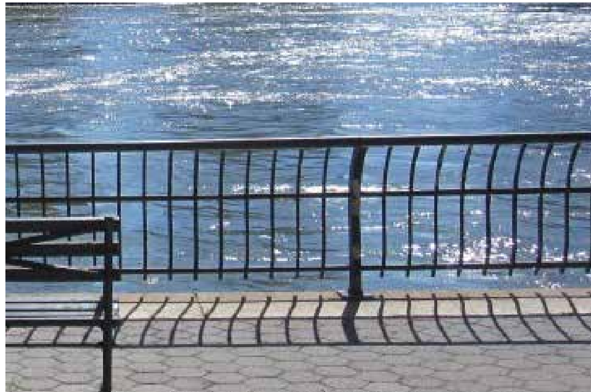
Existing bulkhead - Bow railing (refurbished)
