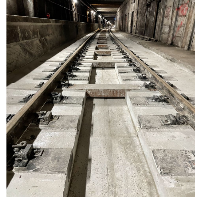
Left: Deteriorated direct fixation track on 63 St Line Below: Rebuilt concrete track on Archer Av Line
