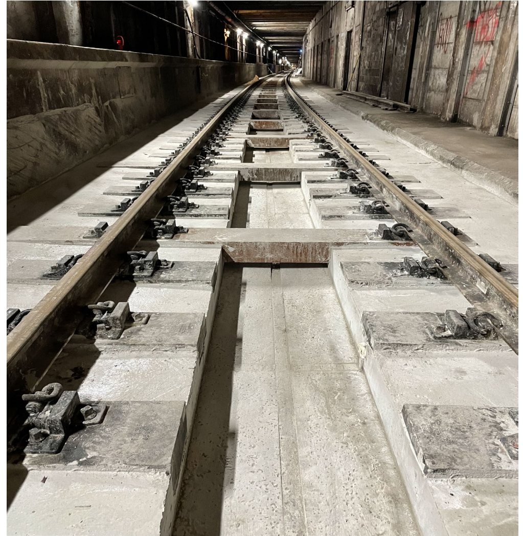
Above: Rebuilt concrete track on Archer Av Line
