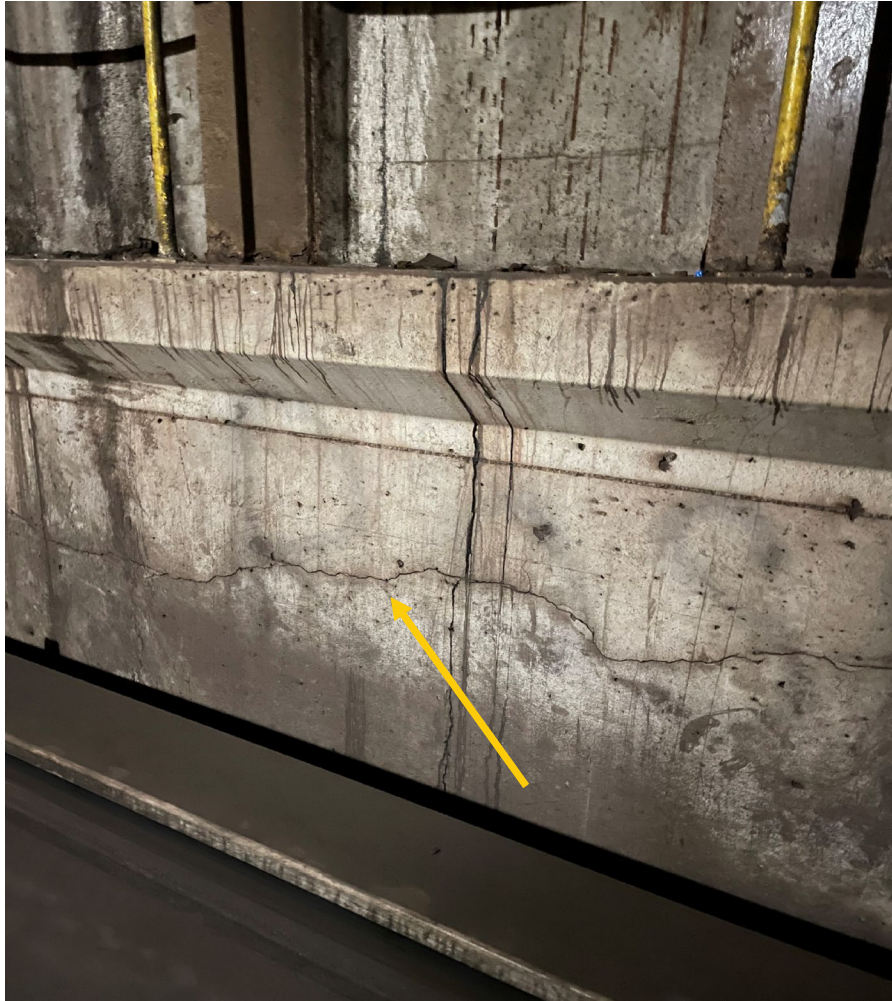
Above: Deteriorated concrete plinth supporting rail on 63 St Line
