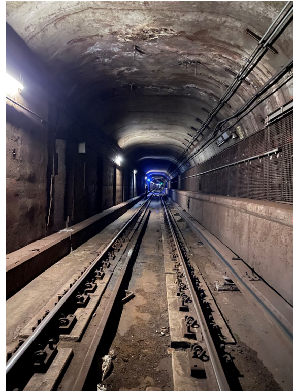
Left: Deteriorated direct fixation track on 63 St Line Below: Rebuilt concrete track on Archer Av Line
