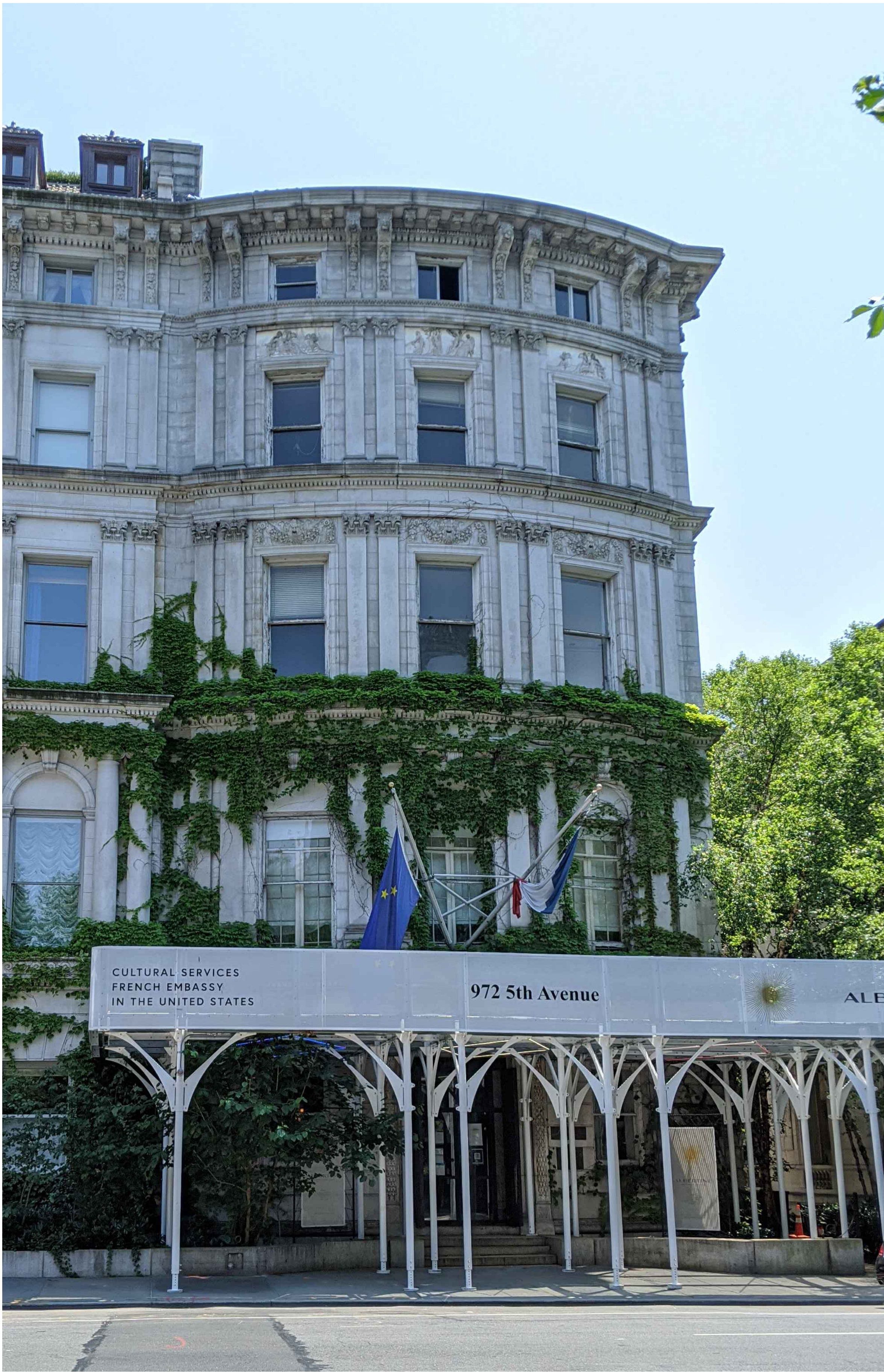
2 PHOTOGRAPH OF THE BUILDING STREET FACADE, FACING WEST SCALE: N.T.S.
