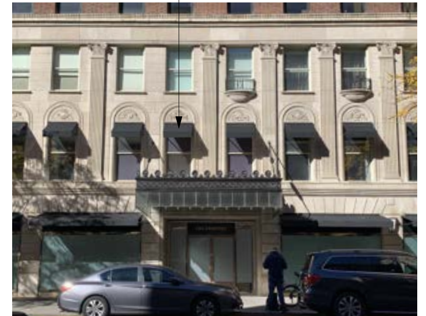
PARTIAL MADISON AVE. FACADE AT MID-BLOCK Existing white double hung windows @ 2nd Fl
