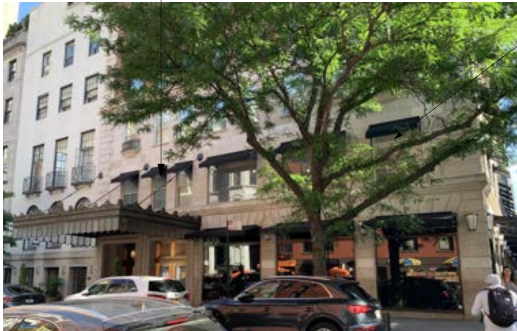
E69TH STREET FACADE Existing white double hung and bronze display windows @ 2nd Fl
