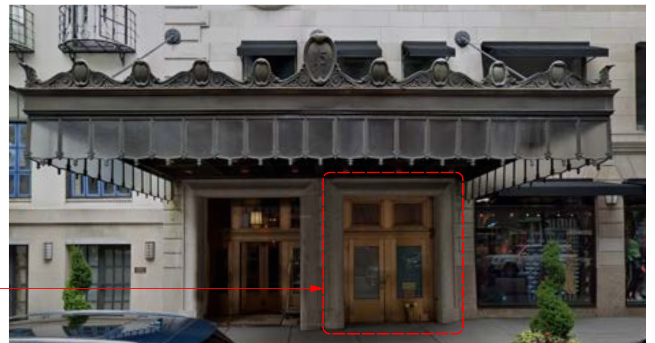
2023 EXISTING E69TH STREET RESIDENTIAL ENTRY AND CELLAR EGRESS DOORS
