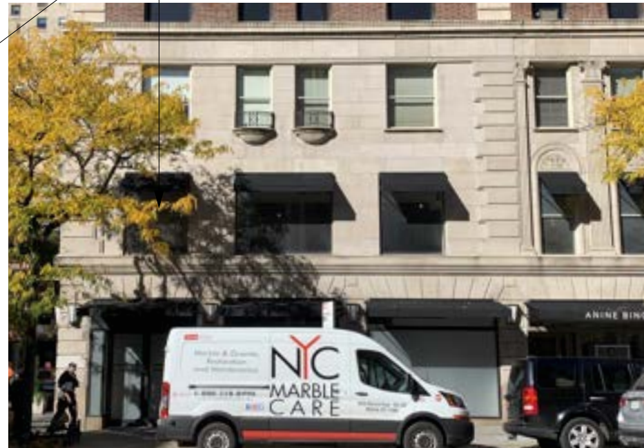
PARTIAL MADISON AVE. FACADE AT SOUTHEAST Existing white double hung and bronze display windows @ 2nd Fl
