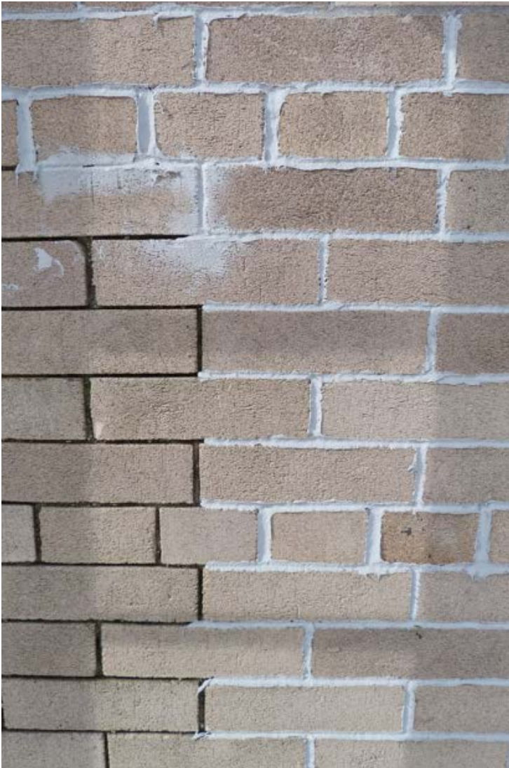
Detail view of poorly done repointing at penthouse elevation.
