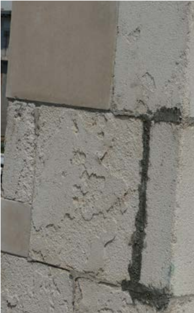
Detail view of stone deterioration at chimney.
