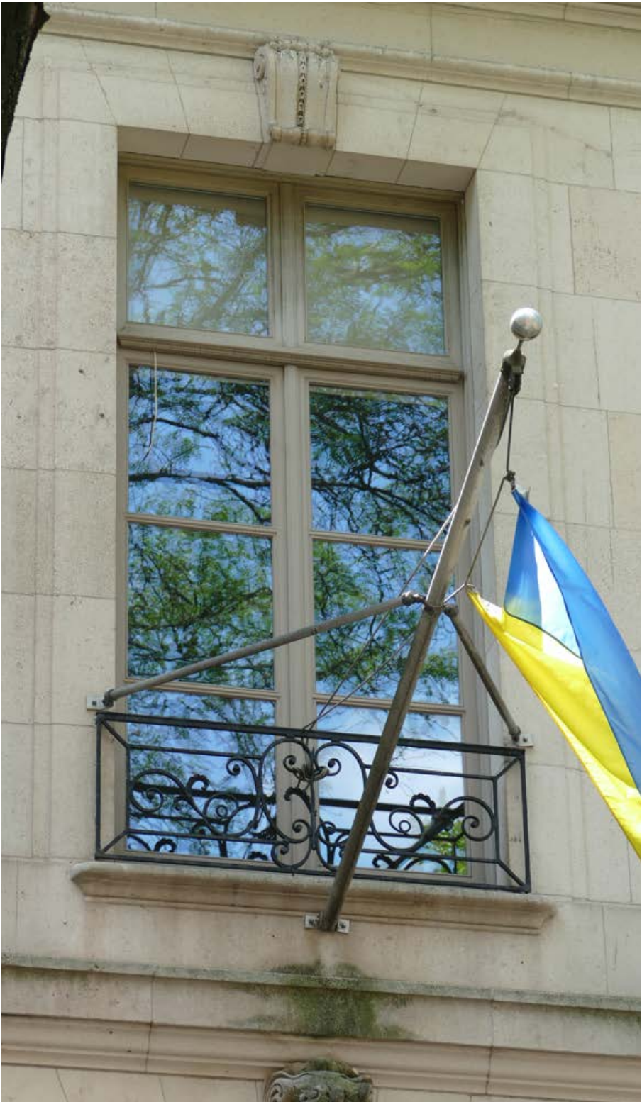
The existing windows at the front facade are retrofitted historic sash with new glazing. The flagpoles will be removed and masonry patched. Biological growth and soiling will be removed.
