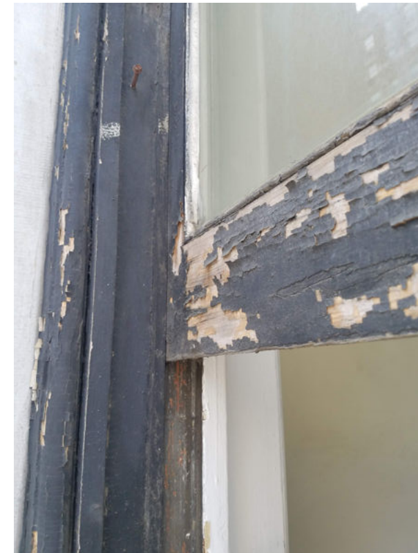
Existing Window - 4th Floor
