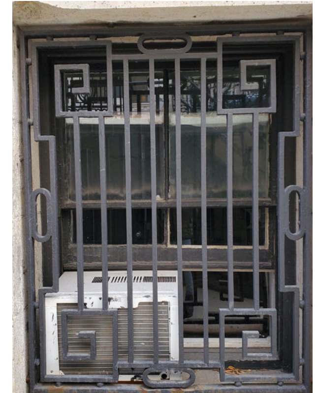
Existing Window - Basement
