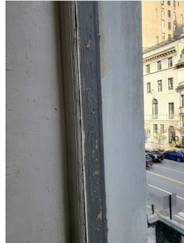
Existing Window - 2nd Floor
