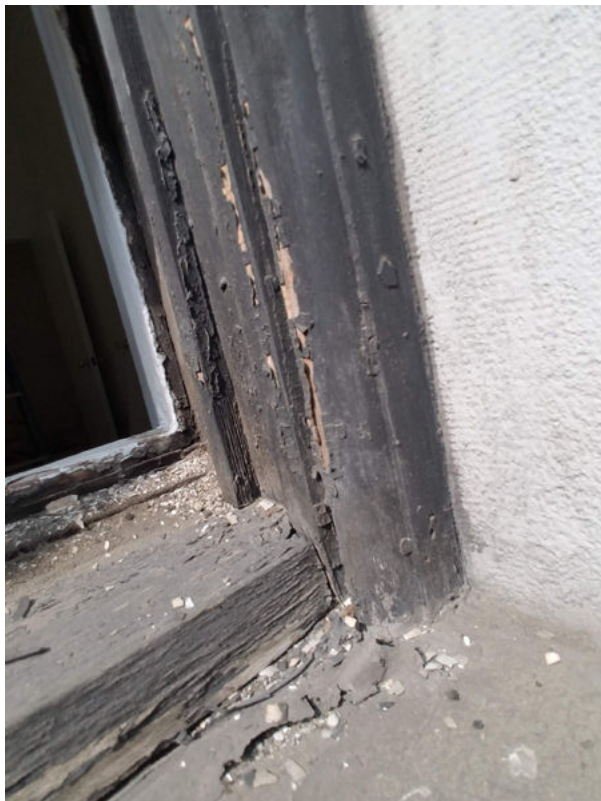
Existing Window - 3rd Floor
