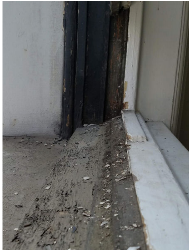
Existing Window - 4th Floor
