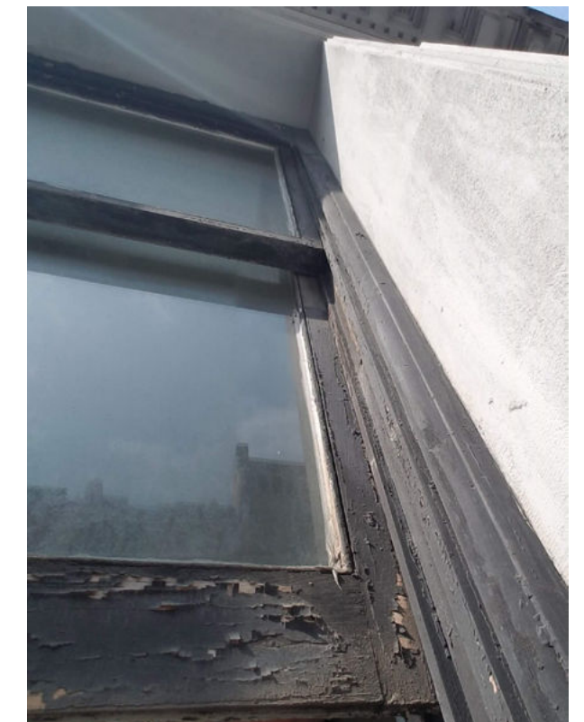
Existing Window - 4th Floor
