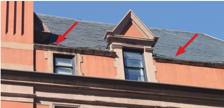
DAMAGED EXG SNOW GUARDS AT SOUTH FACADE
