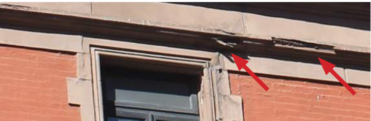
SOUTH ELEVATION: Spalls at sandstone cornice above 3rd floor window.
