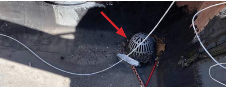
TYP. EXISTING ROOF DRAIN TO BE REPLACED AT FLAT ROOFS.
