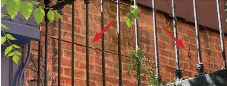
EAST ELEVATION: Cracked mortar observed on SE corner.
