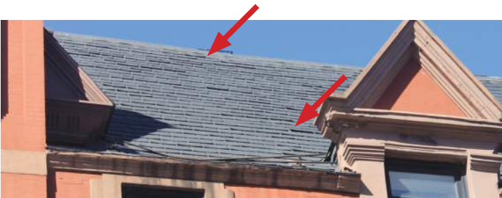
SOUTH ELEVATION: Displaced composite tiles.
