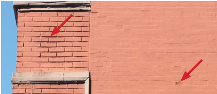
SOUTH ELEVATION: Peeling paint at brick masonry and newer brick veneer.
