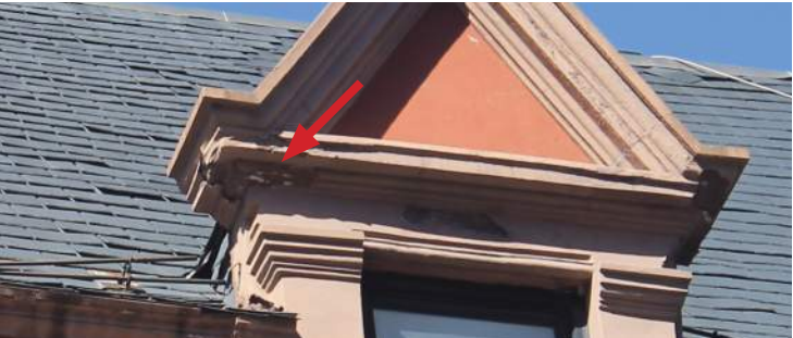
SOUTH ELEVATION: Spall at sandstone cornice at dormer window.
