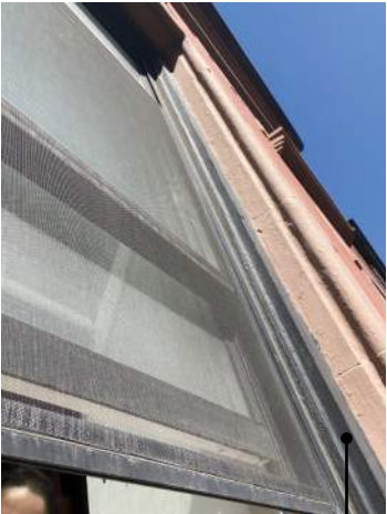
ORIGINAL PAINTED WOOD BRICK MOLD AT 3RD FL WINDOW, 1-1/2" WIDE X 1" DEEP PHOTO OF EXISTING WOOD BRICK MOLD AT THIRD FL WINDOW
