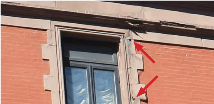
NORTH ELEVATION: Crack at granite unit.
