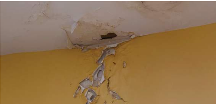
PLASTER WALL AT ROOF STAIR LANDING: Deteriorated plaster due to water infiltration.
