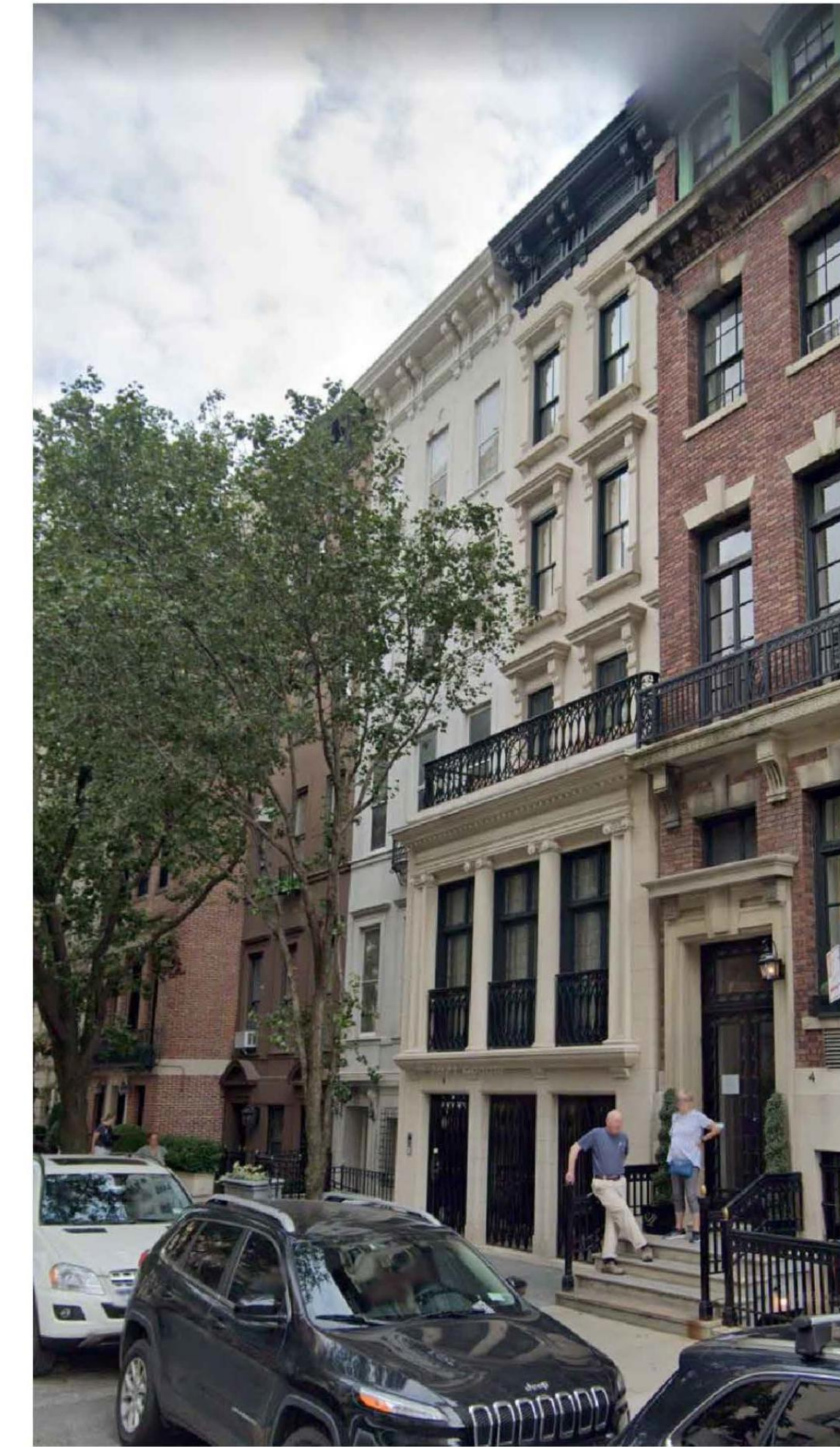
3 6 E 81ST ST - LIMESTONE FACADES Scale N.T.S.
