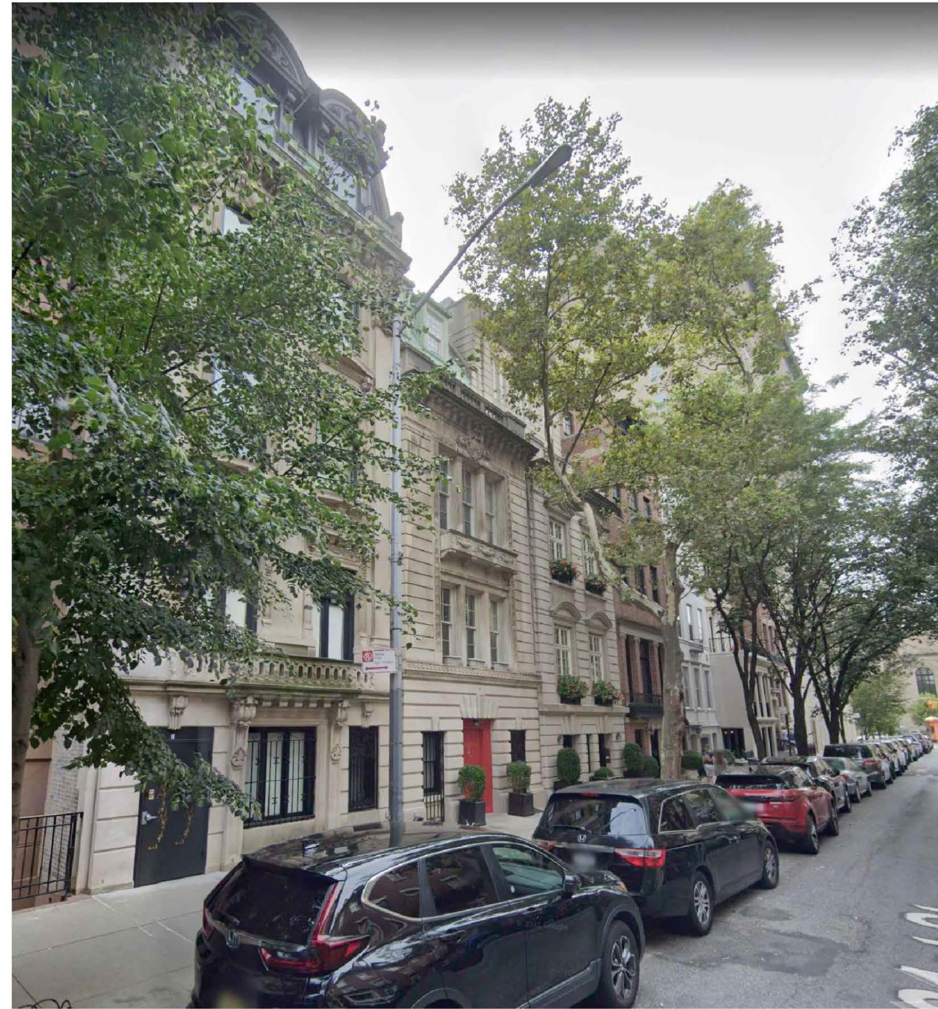
2 14-18 E 81ST ST - LIMESTONE FACADES Scale N.T.S.
