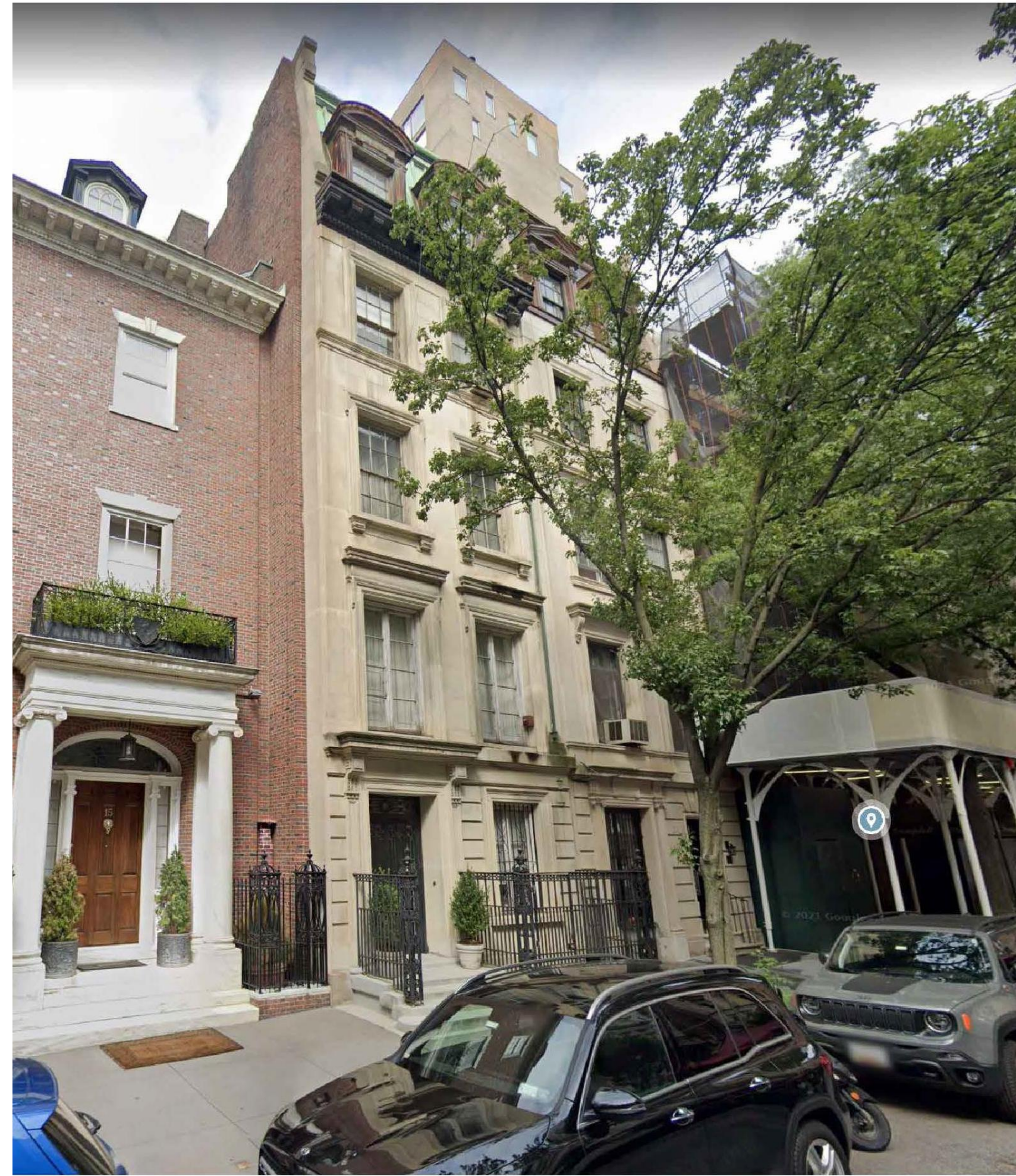
1-23 E 81ST ST - LIMESTONE FACADES Scale N.T.S.
