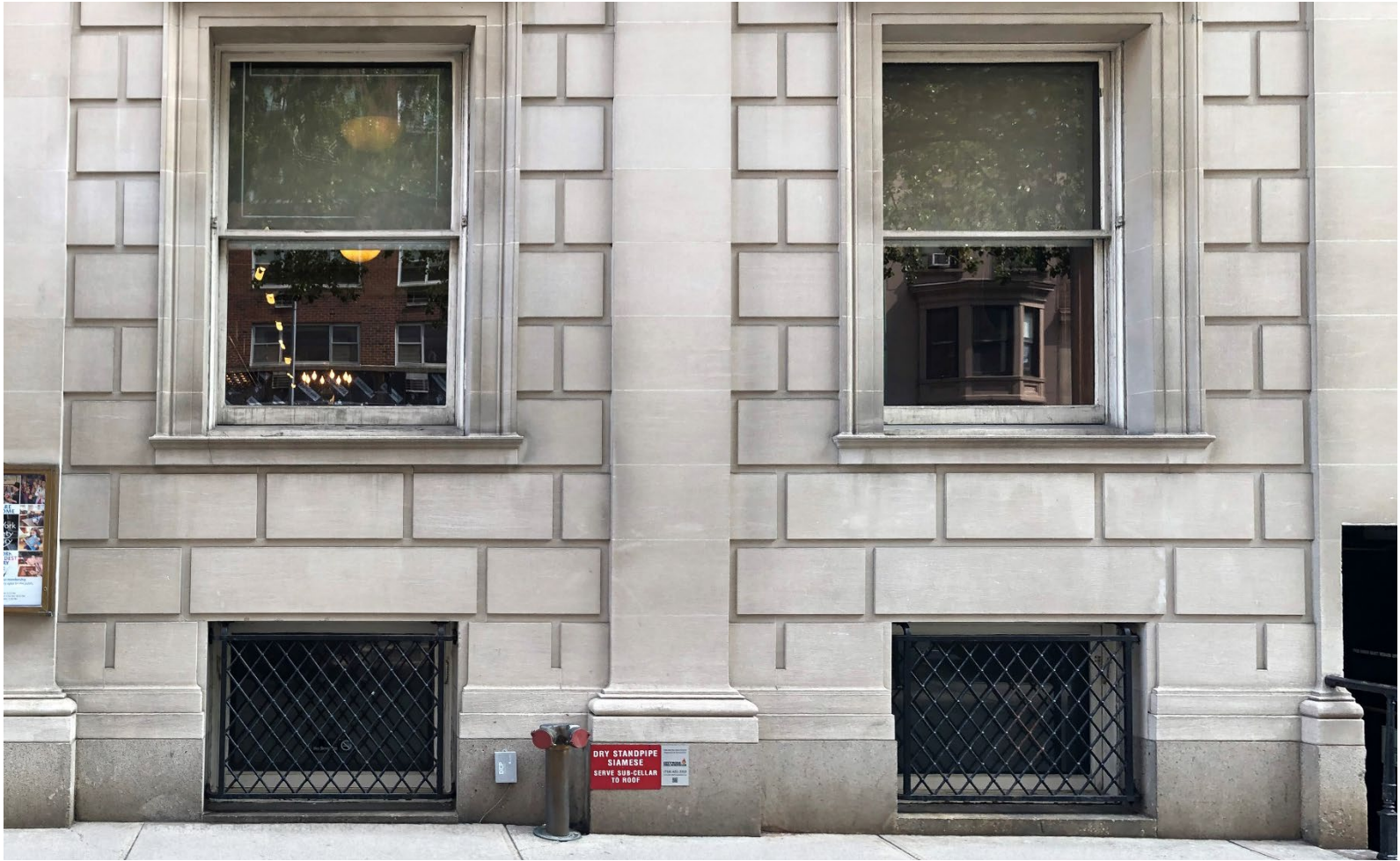
Current view of windows at sidewalk, to be replaced with operable hopper windows to match existing as closely as possible; Existing grilles to remain
