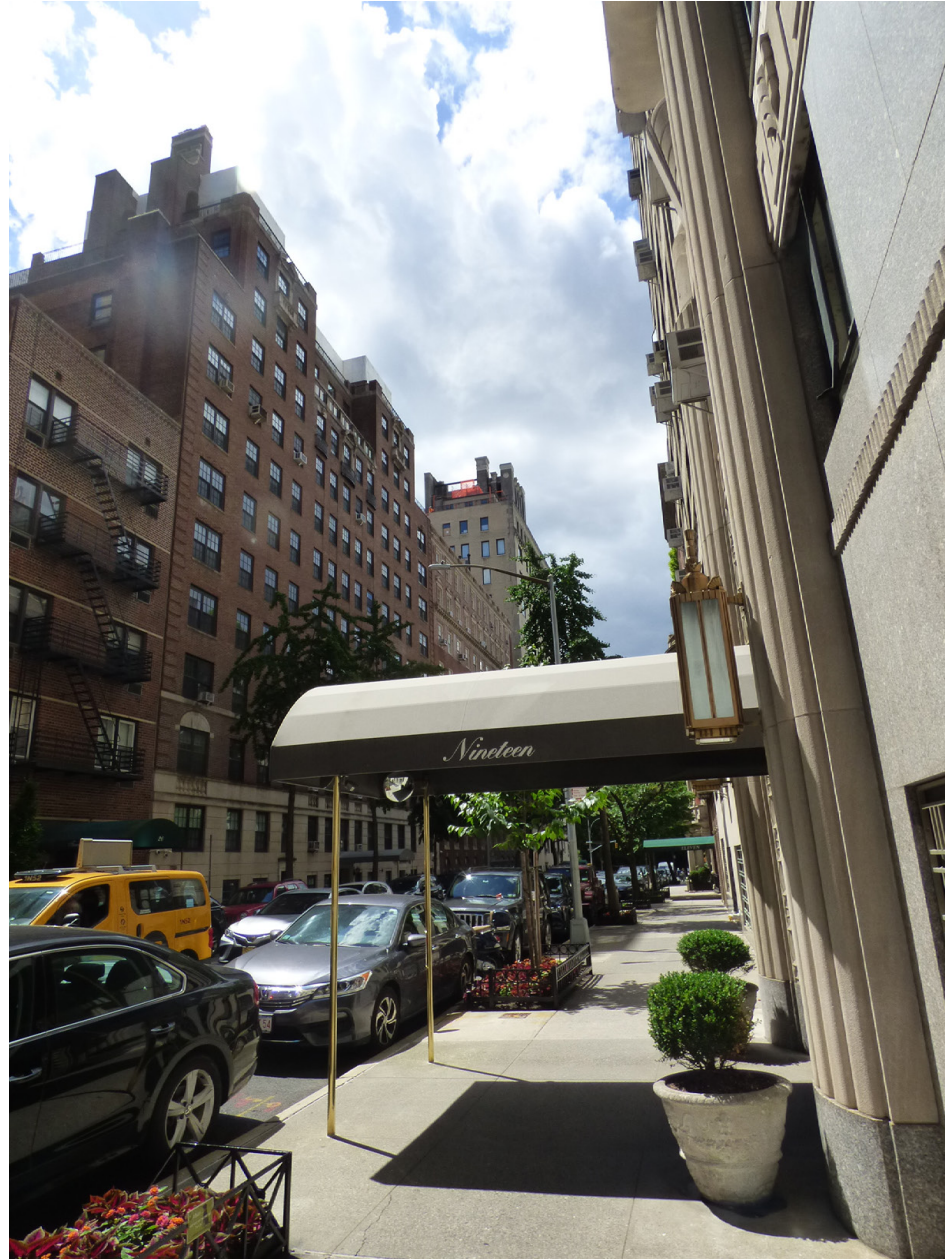
View looking southwest from 88th St and Madison Ave
