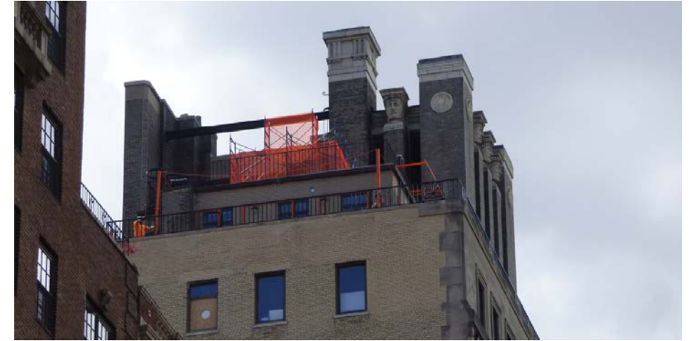
View looking southwest from 88th St and Madison Ave
