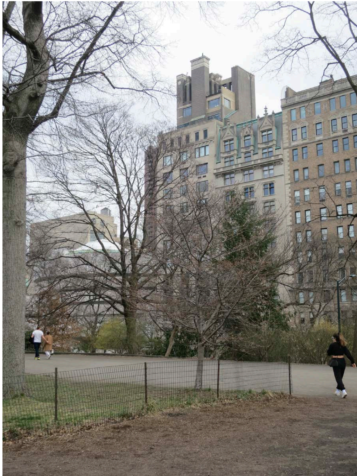
Fifth Avenue facade from Central Park looking northeast
