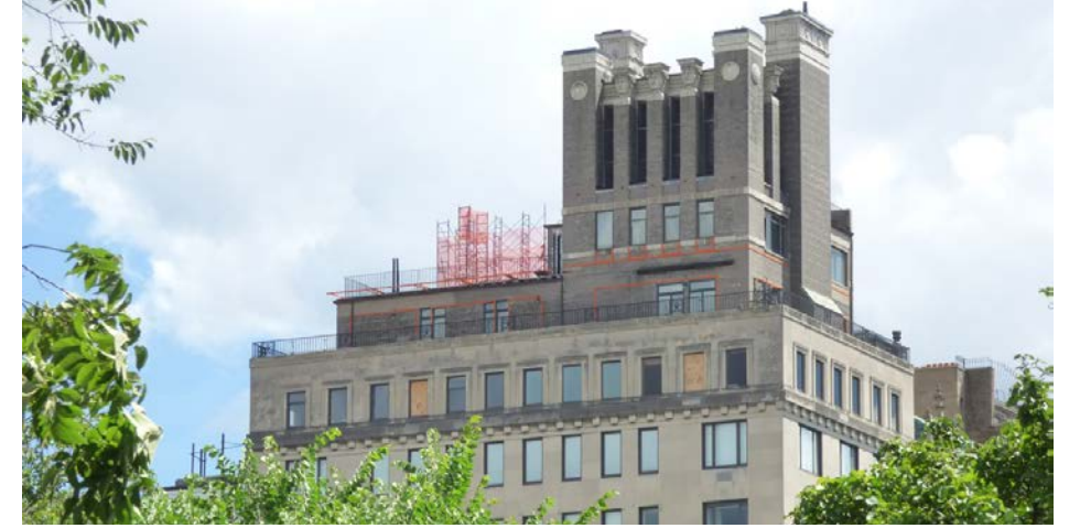
View looking southeast from Reservoir stairs
