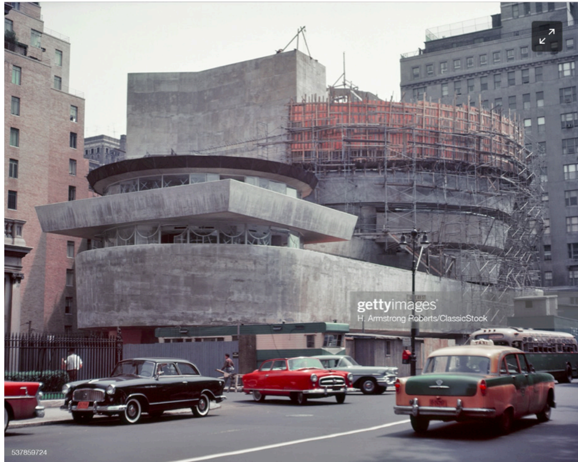
1958 view of Guggenheim under construction with 2 East 88th Street in background (Getty)
